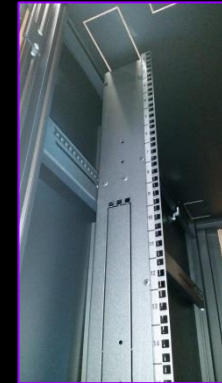
The air guide ensure that the cold air does not pass on the wrong side.
