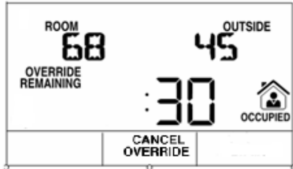
Fig. 36. Override display for Tenant.
