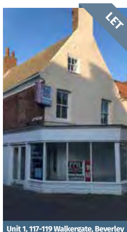
Unit 1, 117-119 Walkergate, Beverley
