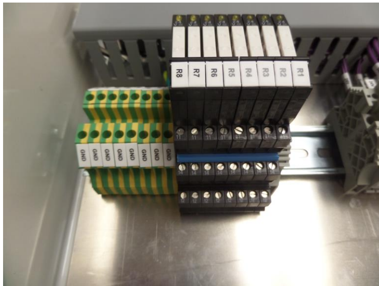
Figure 2 – Pilot Relay Terminal
