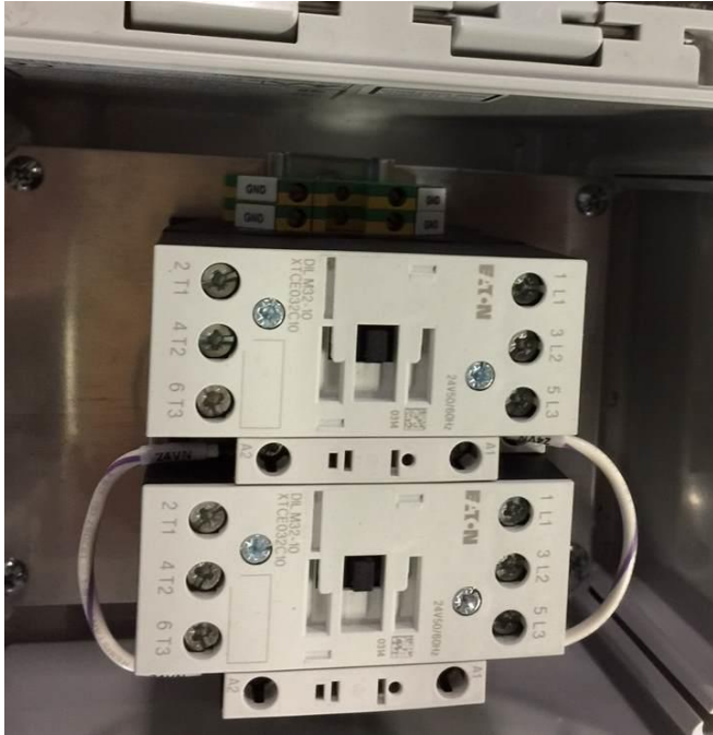
Figure- 3 Daisy Chained Remote Contactors
