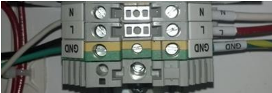
Figure 1: Controller (cPod) Power Connections
