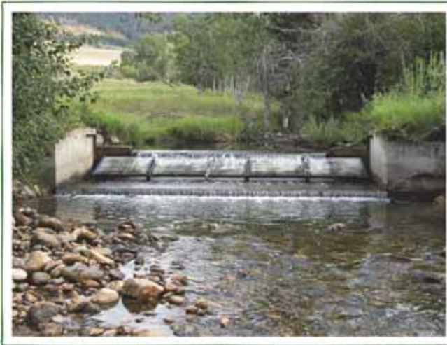
Temporary fish movement barrier on Cherry Creek
