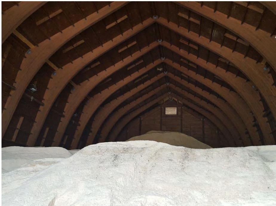
8. Storage Barn Interior
