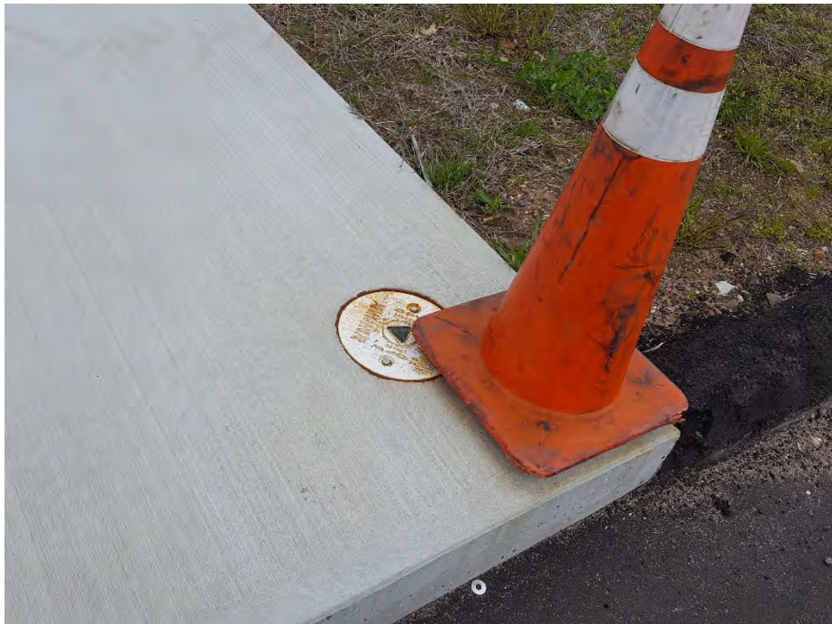
18. Typical Groundwater Monitoring Well
