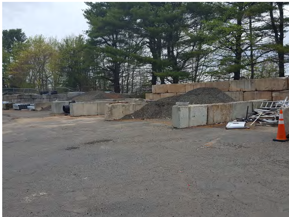
10. Typical Soil Stockpiling
