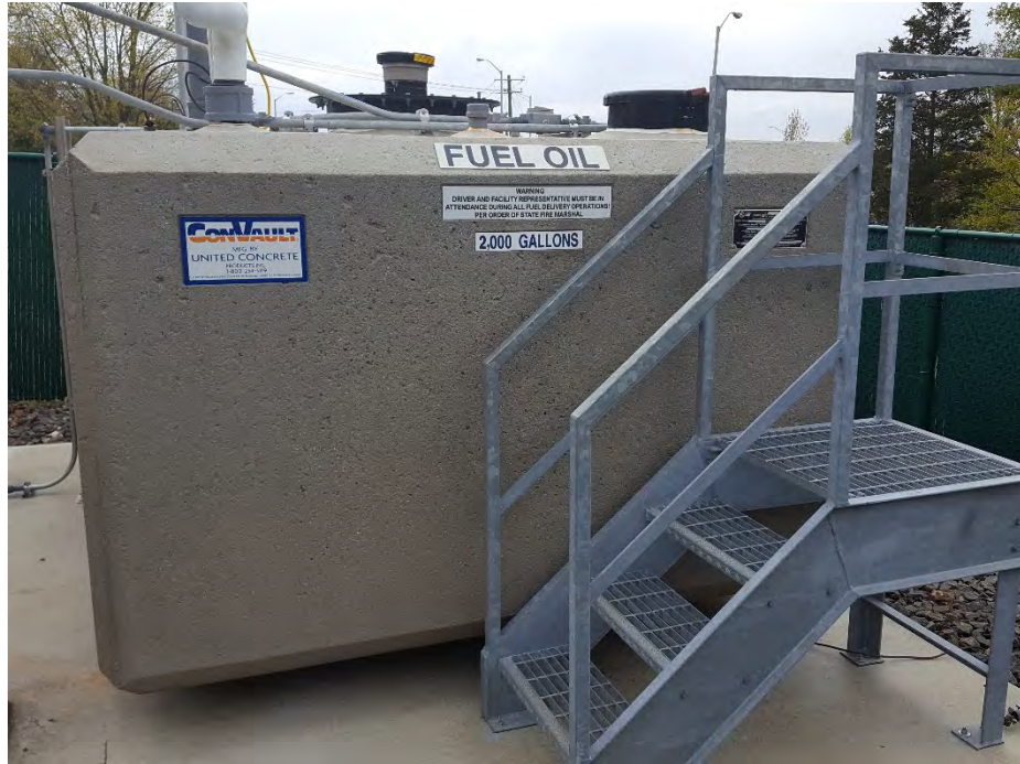
15. 2,000-Gallon Heating Oil AST
