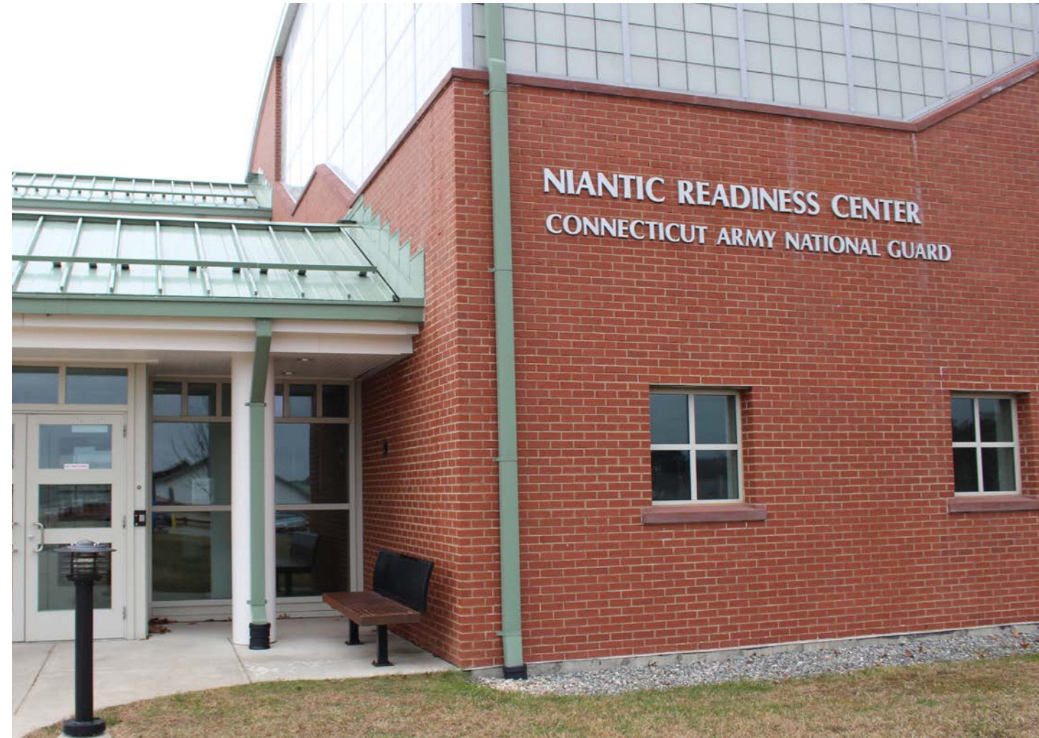
Pictured above is the Niantic Readiness Center for the CTARNG, which is an enduring mission of the CTC. The Niantic Readiness Center features red-brown brick with white accents and a green roof. The design is consistent with new development at Camp Niantic.
