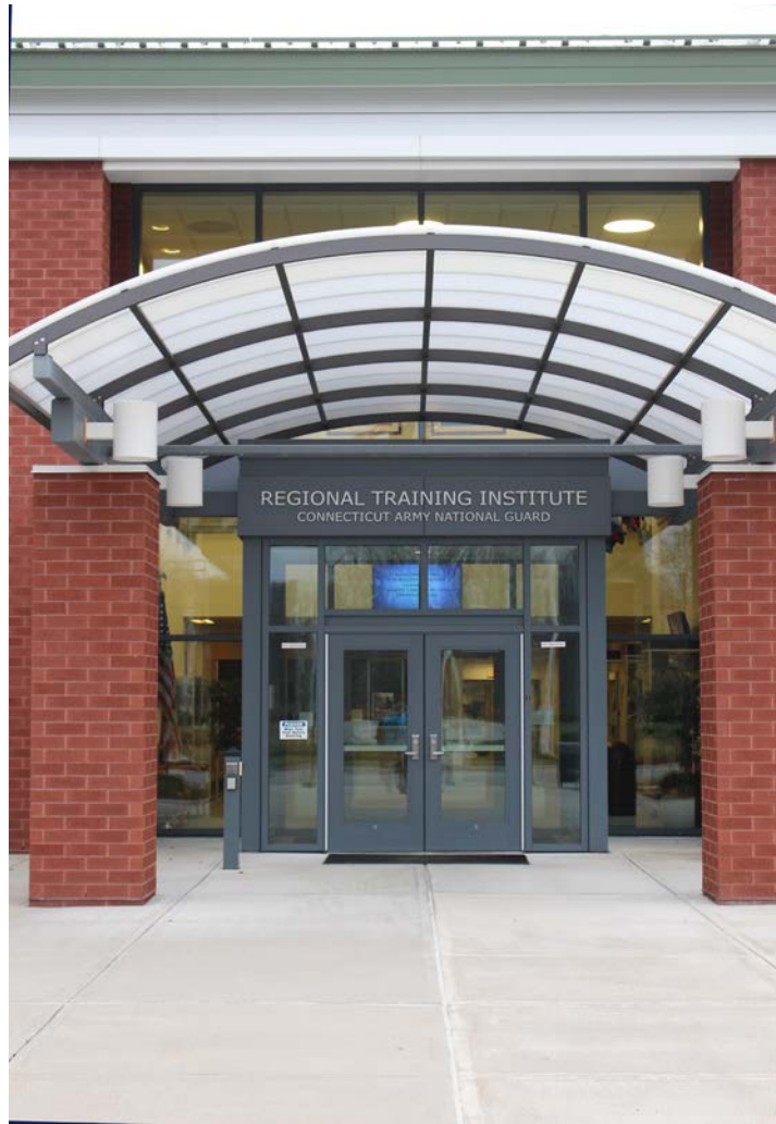
Shown above is the entrance to the RTI for the CTARNG, located at Camp Niantic.
