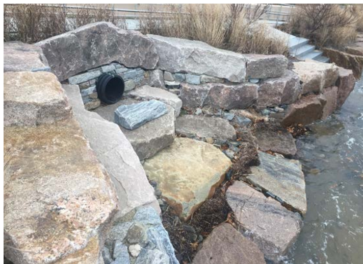
Stormwater culvert at Camp Niantic.
