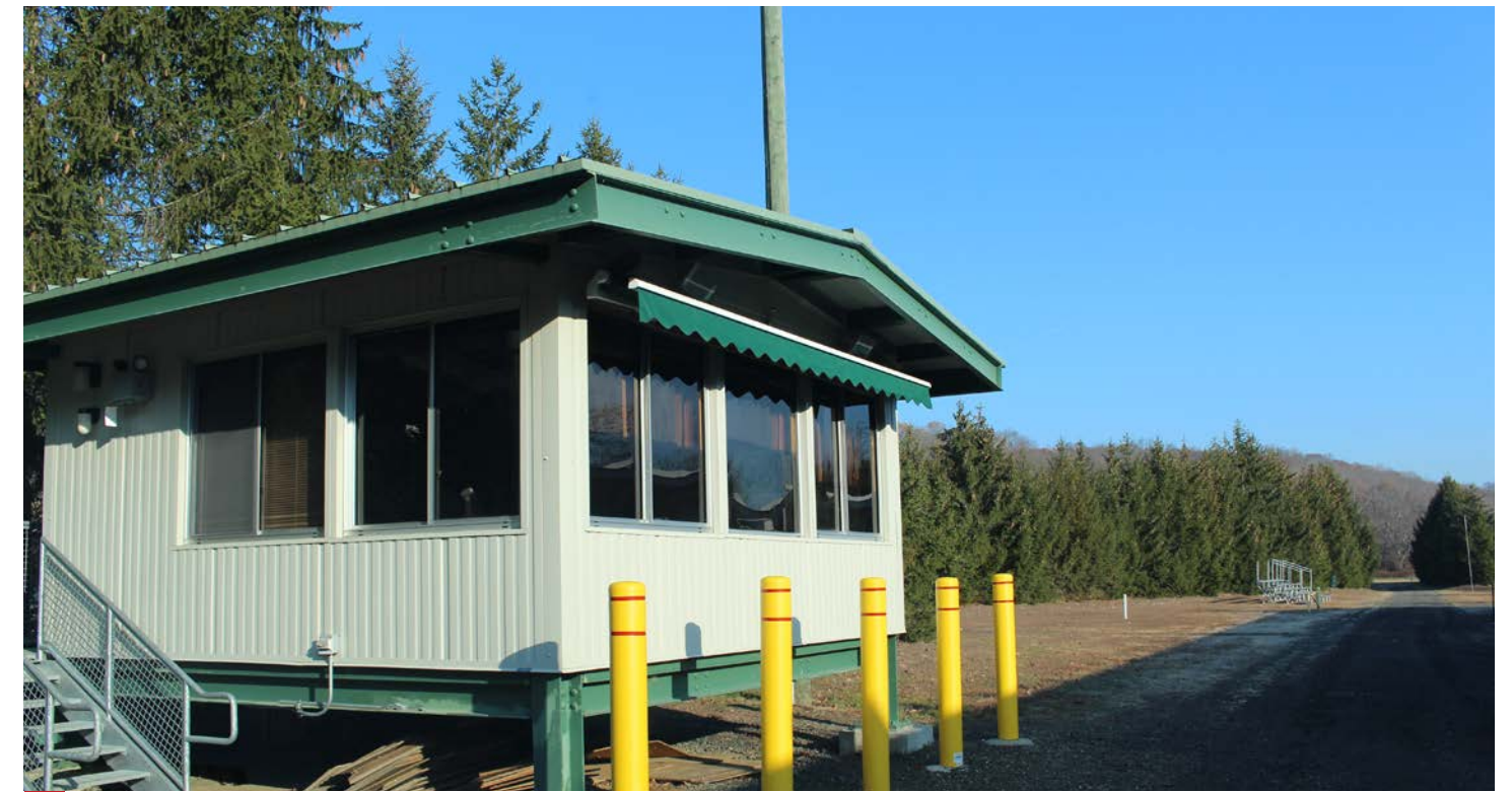
Range Operation Building, East Haven Rifle Range
