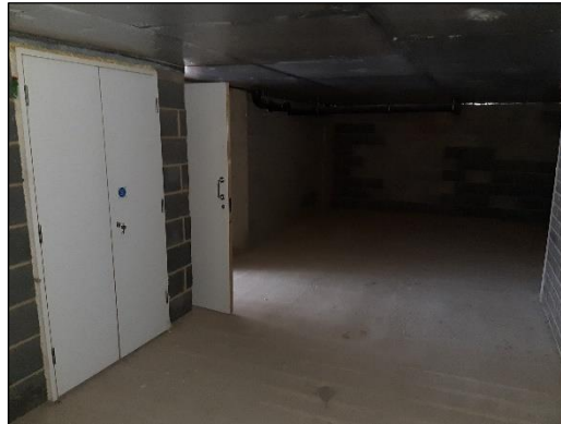
Figure 6: Unit 7 storeroom interior (view southwest).
