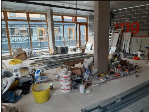
Figure 3: Unit 5 interior (view south).
