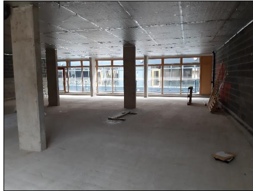
Figure 4: Unit 6 interior (view south).
