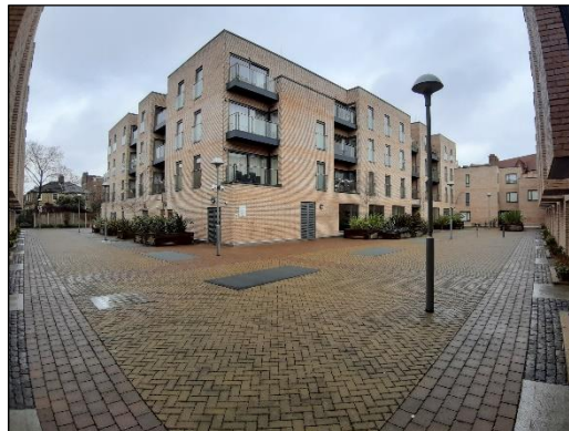
Figure 12: View of external open space over basement car park (view northeast).
