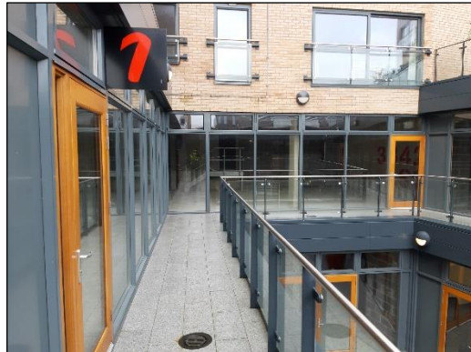
Figure 2: Unit 7, occupying the southwestern corner of the ground floor (view west).
