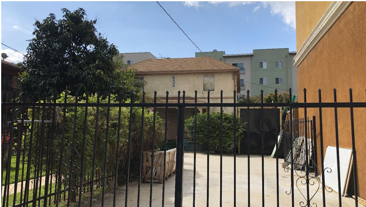
Photograph 2. View of the front of the existing duplex on the site, located at 5446 West Harold Way, looking to the south. The building would be demolished as part of the Project.
