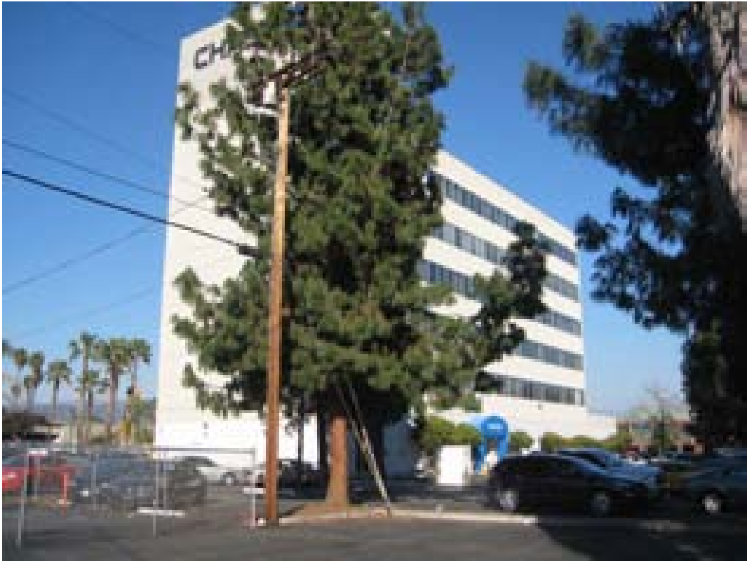
VIEW OF SUBJECT SITE FACING NORTHEAST
