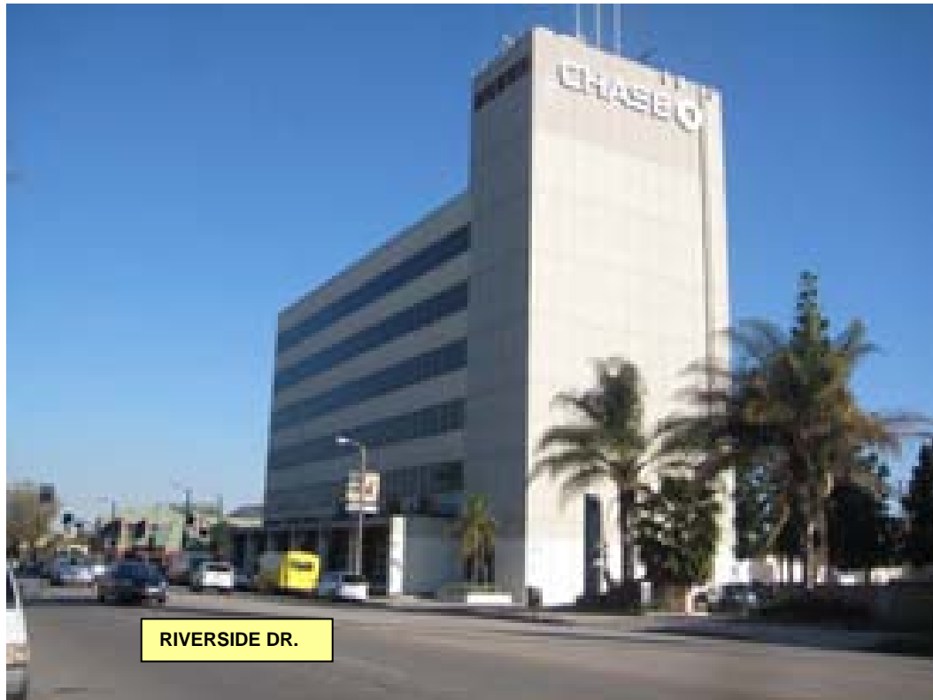
VIEW OF SUBJECT SITE FACING SOUTHEAST
