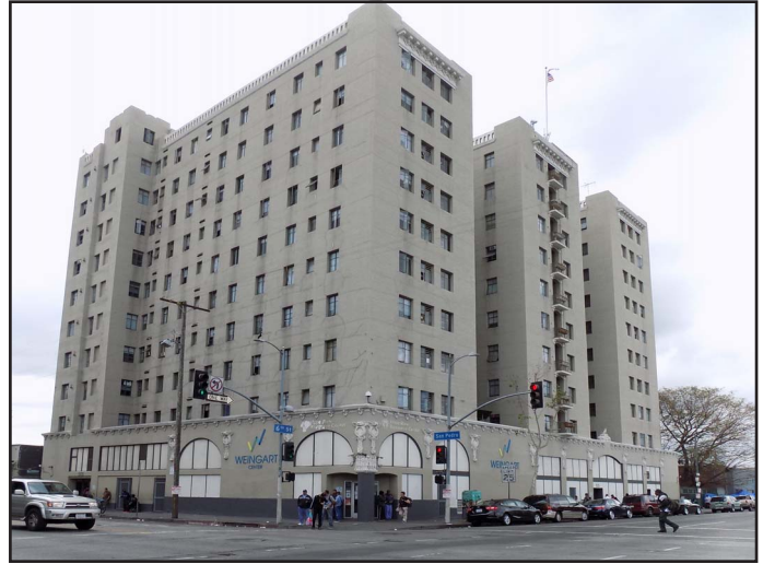
View 6: View looking northeast on the intersection of San Pedro Street and 6th Street at the Weingart Tower adjacent to Site 1.
