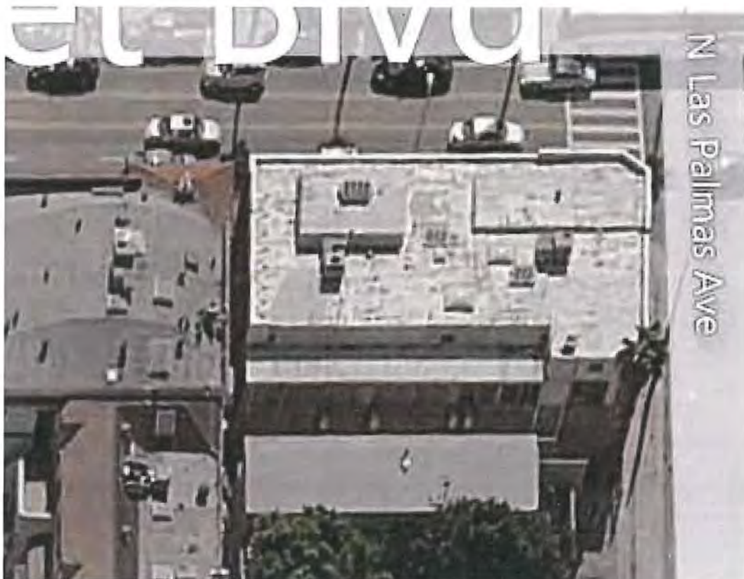
Aerial view: Sunset Blvd/south; N Las Palmas/west, view south.
