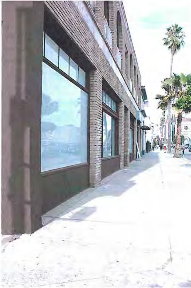
View along Sunset Blvd, east, from southwest entry/6693: Showing theme & variations on display windows. Note Slight downgrade of sidewalk away from building for drainage.
