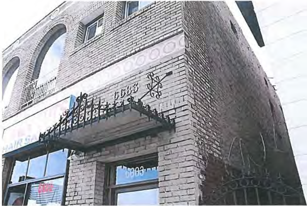
Limited view of east elevation: Executed in red brick; appears to have little fenestration, view northwest.
