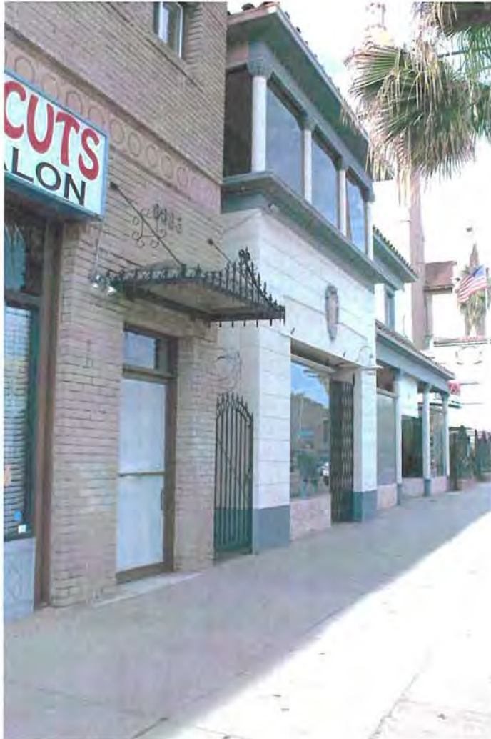
View east along Sunset Blvd, to east end of Bullinger: Non-original glass and wrought iron canopy above entry to 6683/second story apartments/studios/offices.
