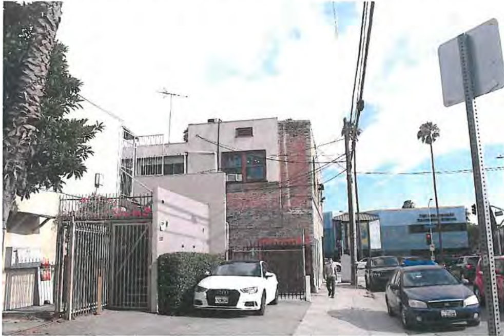
Rear of Bullinger Building: 1510 Las Palmas in foreground. Shows addition and plastered brick wall at rear of vehicle entry, gated, view south.
