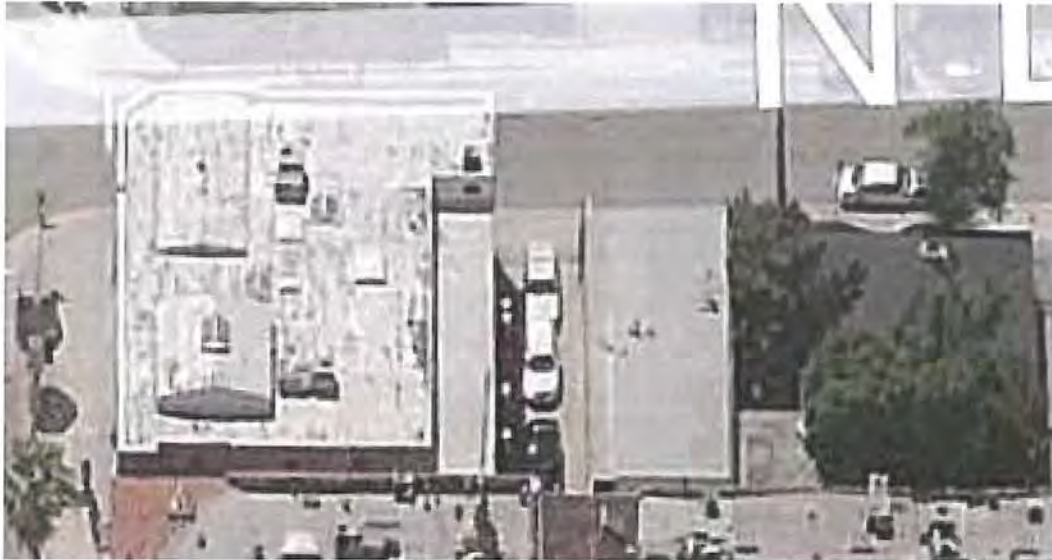
Aerial view: Sunset/south, left; N Las Palmas/top, view west.
