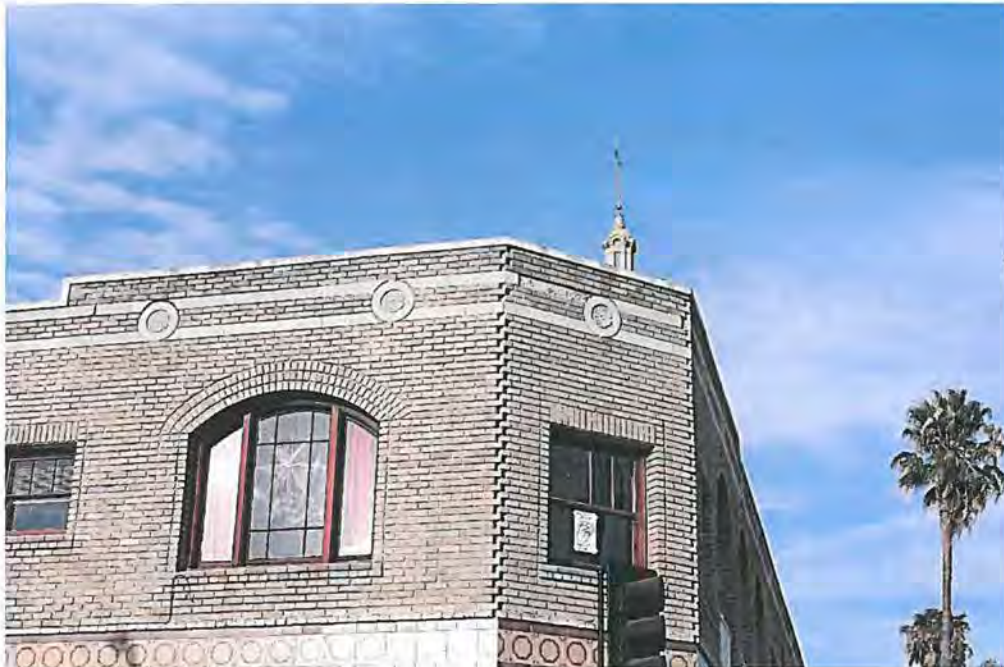
West elevation, northeast corner entry: Parapet wall with strip of marble at top edge, double marble stripes enclose flowers within circles; one of pair of three-over-onewindows; arched window, 9-panes/plain sidelights; interlocking bricks at diagonal corner; tile band replaces original concrete molding band; four-over-onewindow in diagonal wall; view east.
