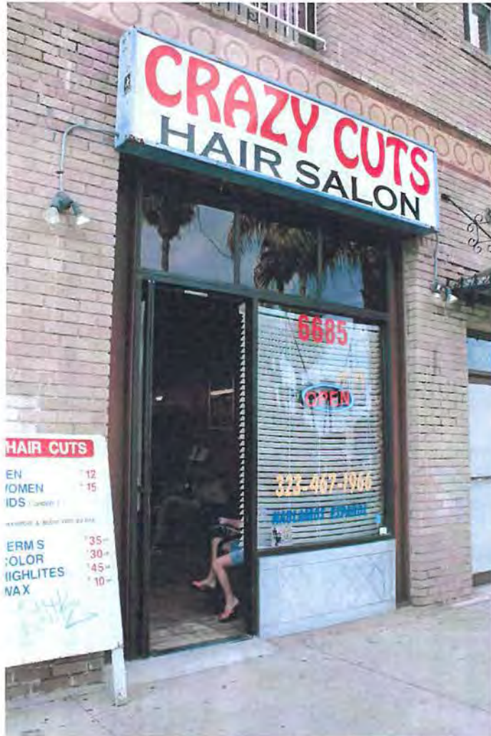
Exterior 6685 Sunset Blvd: The smallest ground floor space with original entry and diamond patterned scored concrete beneath window, view northeast.
