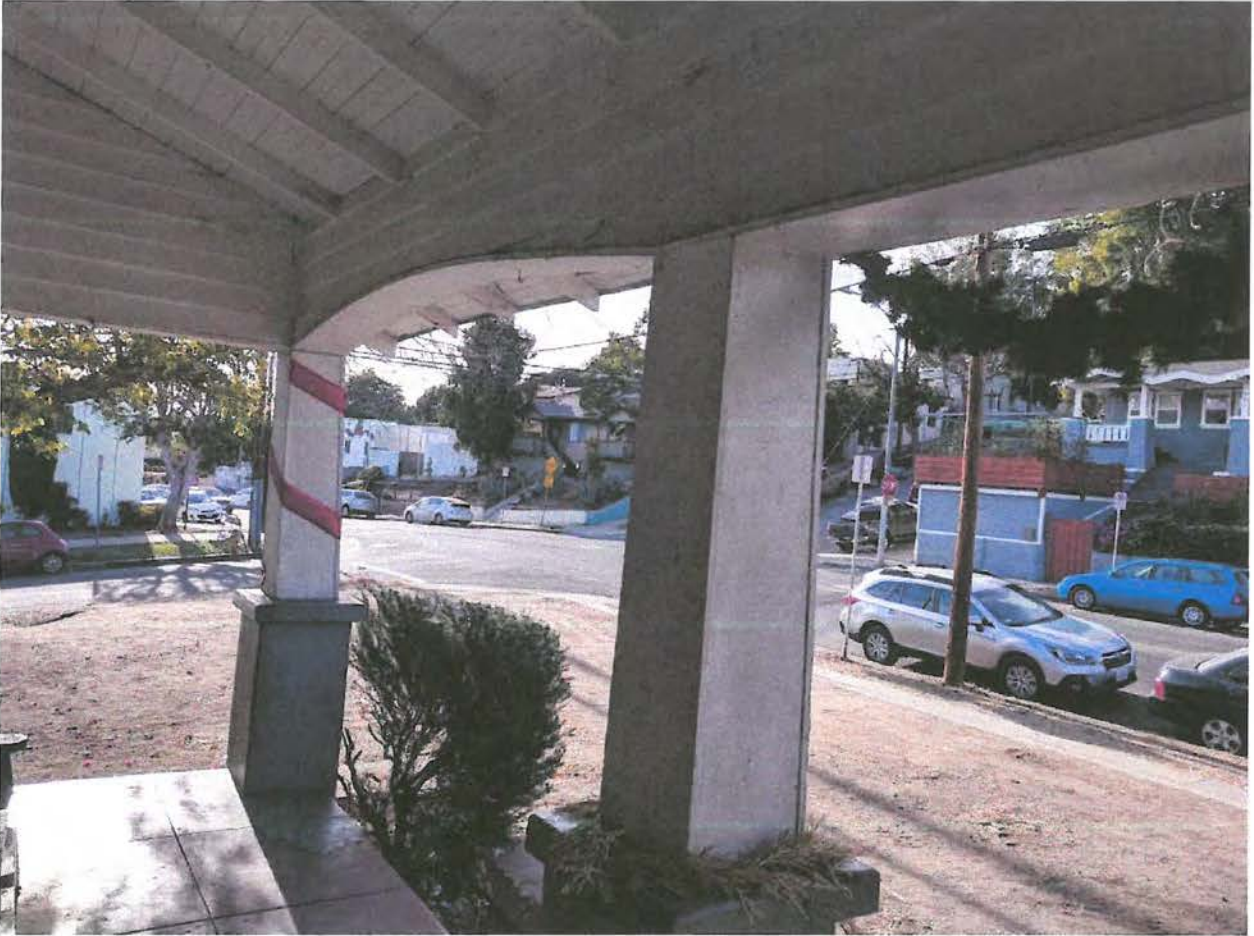
Tapered columns, concrete bases, roof eaves and arched façade of porch
