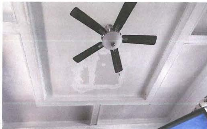
Living Room Box Beams
