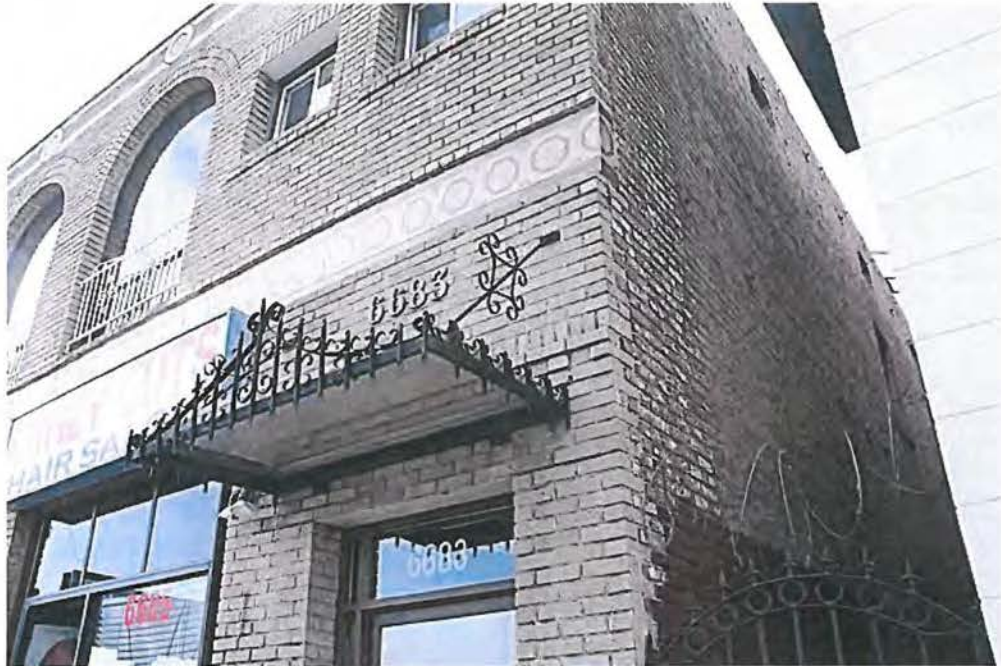
Limited view of east elevation: Executed in red brick; appears to have little fenestration, view northwest.
