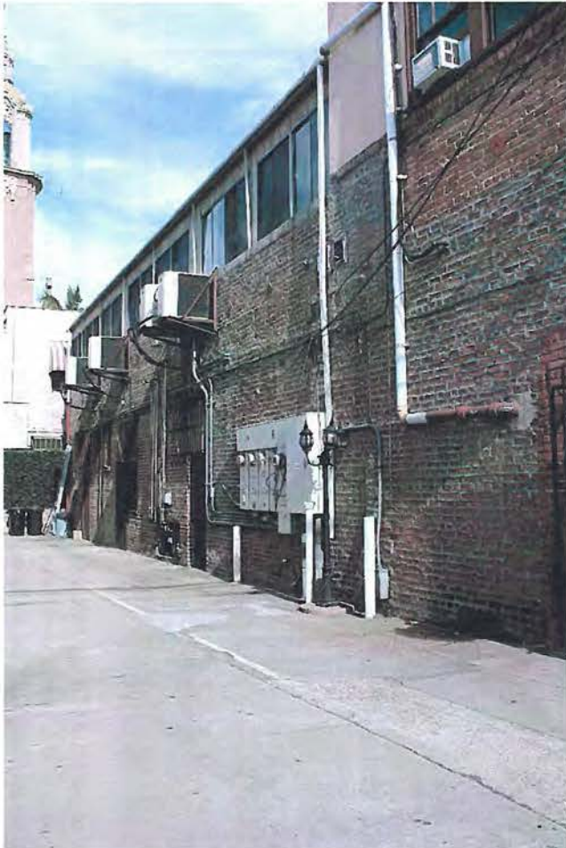
North elevation: Second level added slider windows at breezeway, racked AC units; seismic reinforcement; added pipes/conduit at building exterior; power panel with pipe buffers; rear entries w/ original fenestration at ground floor; cement paving, view southeast.
