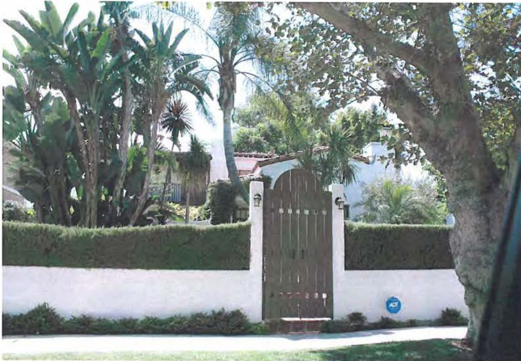
451 Milton Street, currently 451 Mansfield Avenue in Spanish type architecture.
