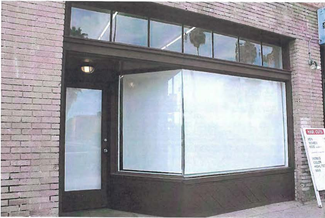
Final bay of Overduin Art Gallery at east on Suset Blvd, next to 6685, view northeast.
