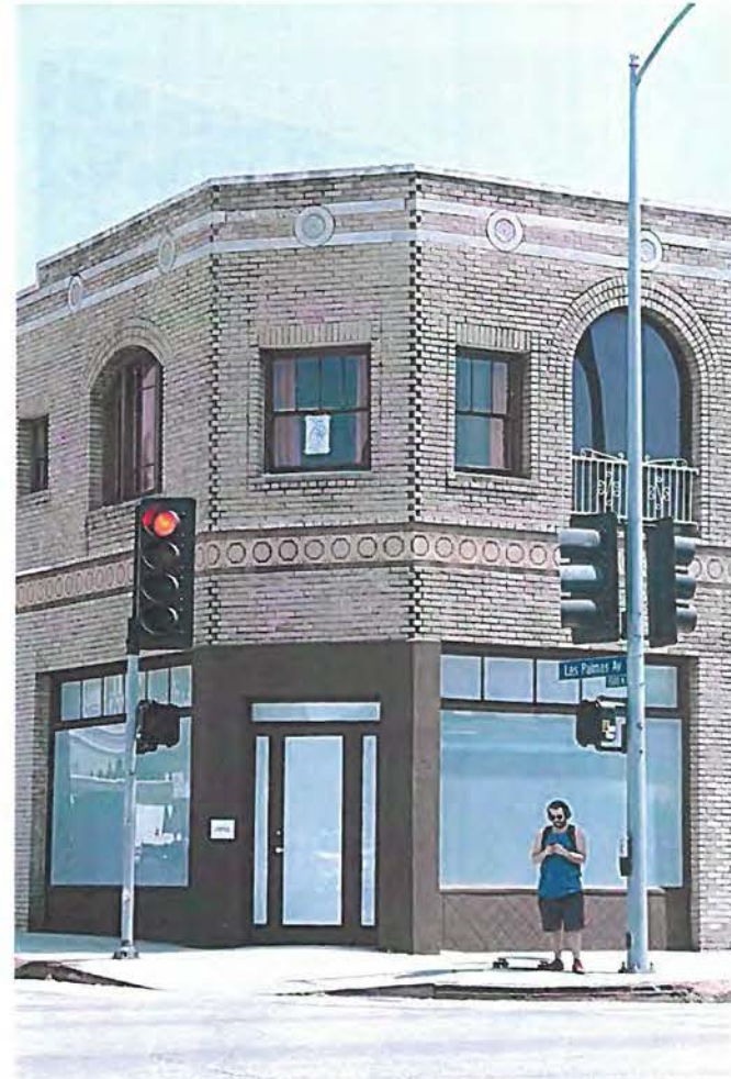
Two story diagonal entry from NE intersection of Sunset Blvd. & Las Palmas Ave. topped by low parapet wall of brick and marble with intersecting bricks. Only non-original element is tiled band.
