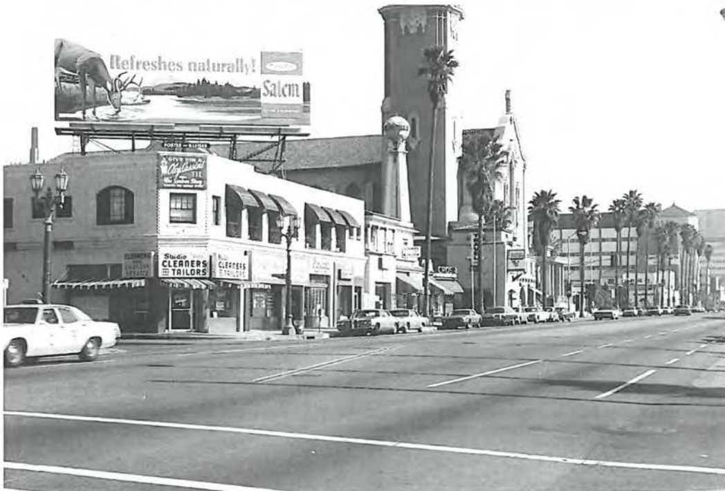
Bullinger Building at corner of Sunset Blvd and Las Palmas Ave with billboard on roof: 1963. The Bruce Torrance Hollywood Photograph Collection.
