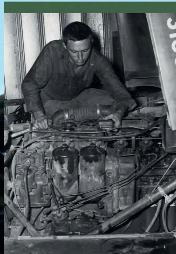
Sergeant Larry Don Stock of the 1st Motor Transport Battalion carries out routine engine maintenance on an M35 series truck on September 19, 1967. The engine is multi-fuel/diesel, making the truck either an M35A1 or an M35A2 (SERGEANT RP CURRY / 26393805)
