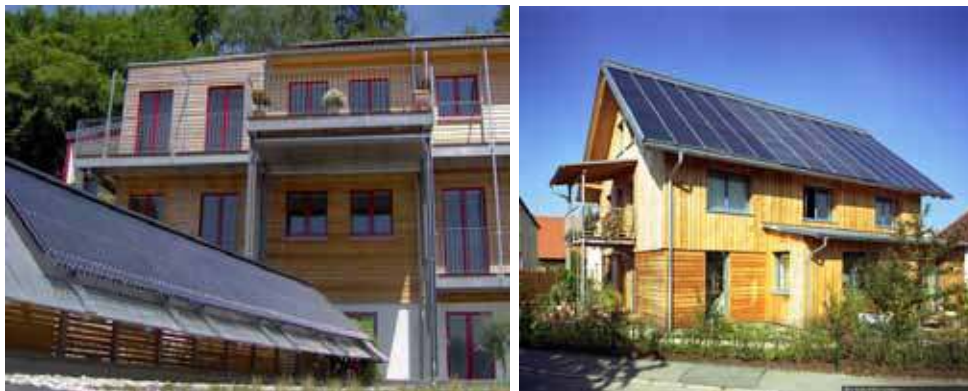
Figure 2.11. Two examples of aesthetic placements of collectors. At the right the collectors are integrated into the roof cover together with PV collectors at either side.
