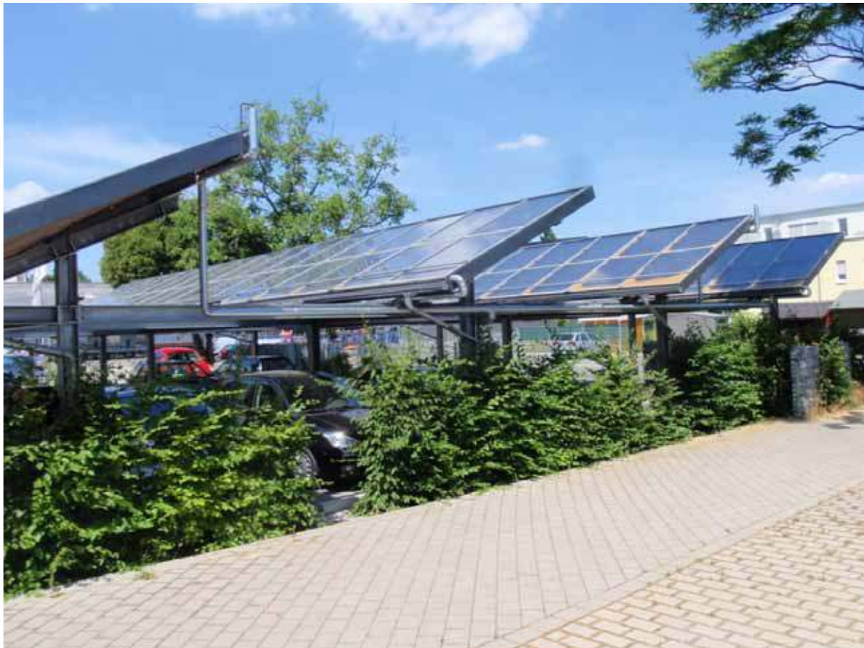
Figure 5.1. Solar hot water collectors placed above automobiles where they are parked.
