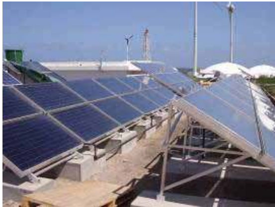
Figure 2.10. Flat plate collectors on mounting construction.
