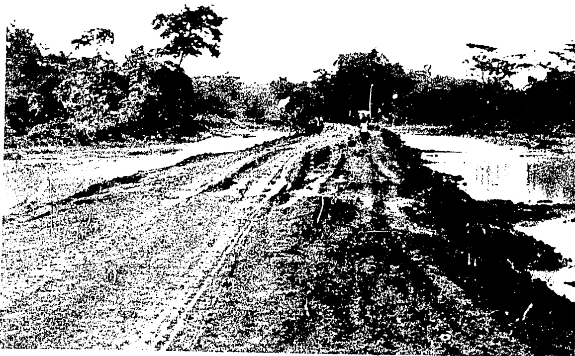
Sideborrow construction often creates standing water, a situation that requires proper ditching before road is completed (Liberia). (Photo courtesy of USAID/Liberia.)
