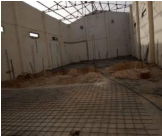
Figure 11: Diourbel PRA renovation image 1 of 2
