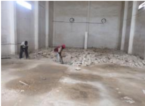
Figure 9: Fatick PRA renovation images 1 of 2
