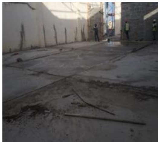
Figure 12: Diourbel PRA renovation image 2 of 2
