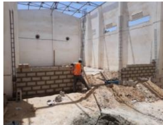
Figure 10: Fatick PRA renovation images 2 of 2
