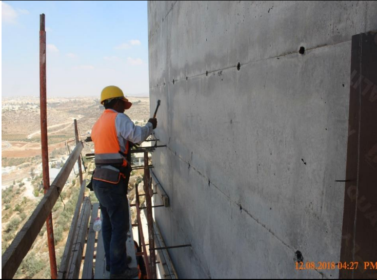
Photo #23 – Formwork De-Shuttering of the Reservoir’s Walls
