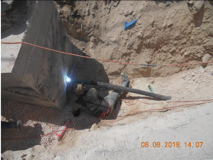
Photo #17 – Welding for Chambers Connection
