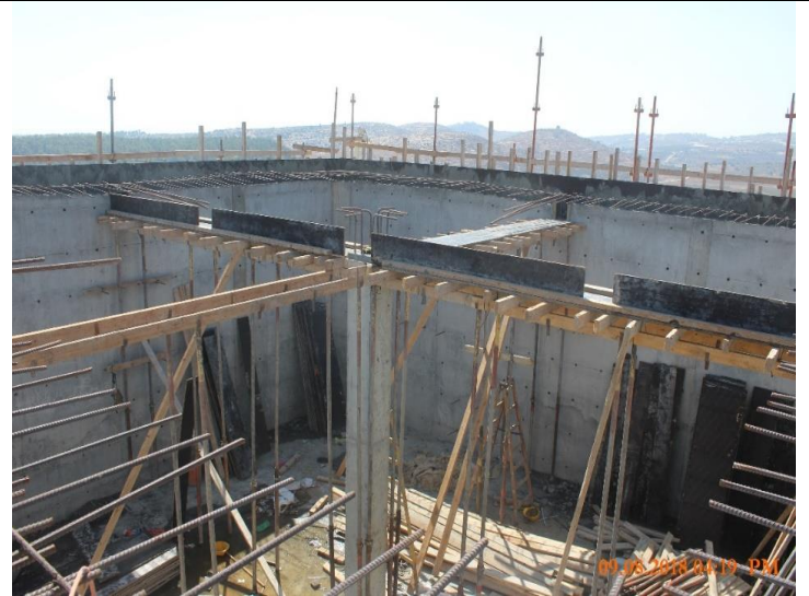
Photo #18 – Formwork for the Reservoir's Top Slab
