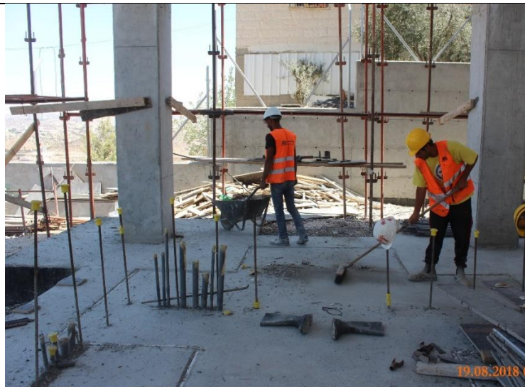
Photo #46 – Housekeeping at the Reservoir's Site
