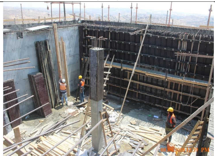
Photo #16 – De-shuttering of Formwork for the Reservoir's Walls
