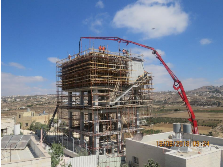
Photo #41 – Casting Concrete for the Reservoir's Top Slab
