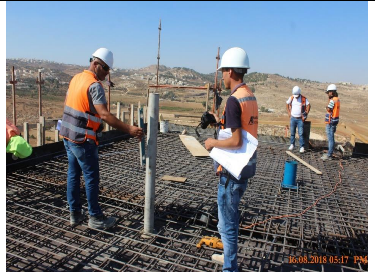
Photo #38 – Inspecting of Roof Slab Thimbles
