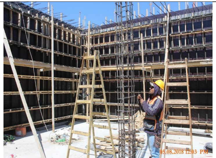
Photo #10 – Steel Reinforcement for the Reservoir's Central Column
