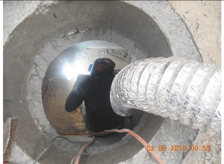
Photo #06 – Installation of Mechanical Fittings
