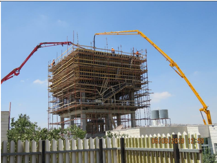
Photo #13 – Casting Concrete for the Reservoir's Walls
