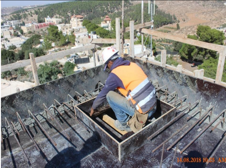
Photo #29 – Formwork for the Reservoir’s Top Slab
