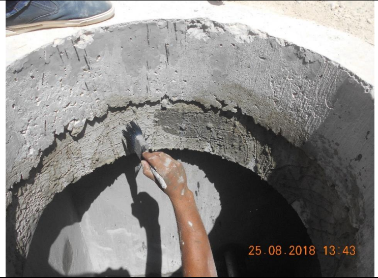
Photo #48 – Internal Concrete Repair inside Pre-Cast Manholes
