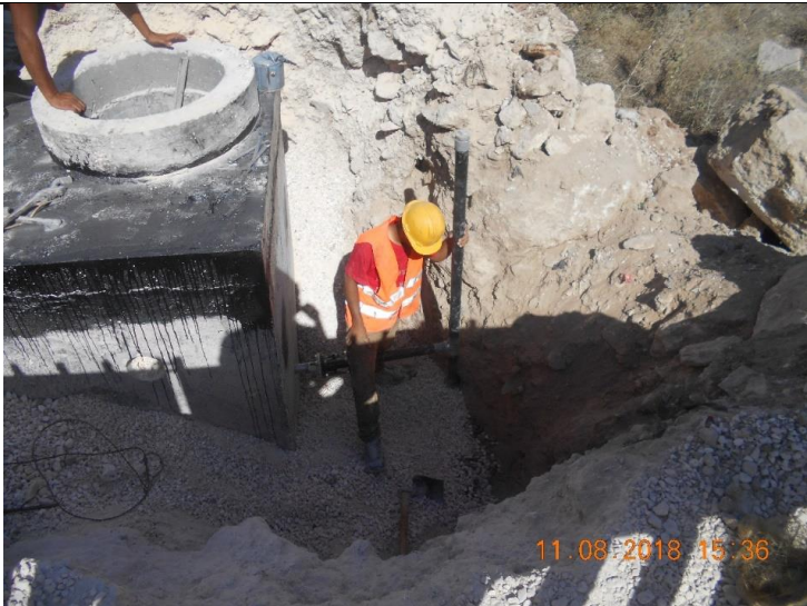
Photo #21 – Installation of Washout Outfall
