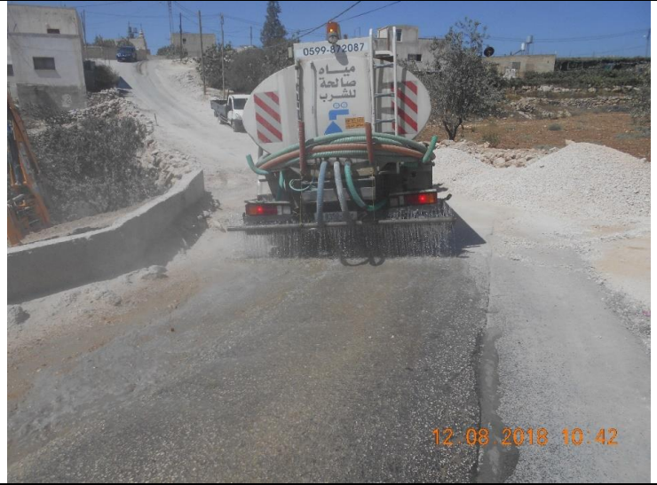
Photo #24 – Dust Control at the Network Site
