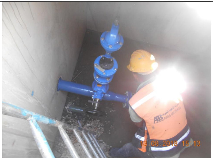
Photo #28 – Installation of Mechanical Fittings inside Main Connection Chamber
