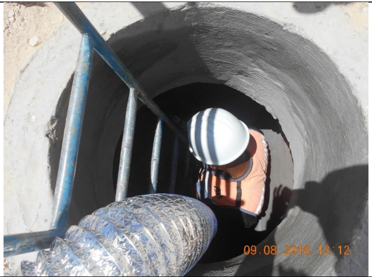
Photo #20 – Internal Concrete Repair for Pre-Cast Manholes
