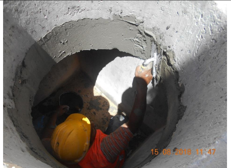
Photo #36 – Internal Concrete Repair for Pre-Cast Manholes
