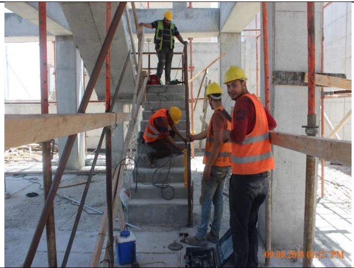
Photo #19 – Erecting Handrail Sample
