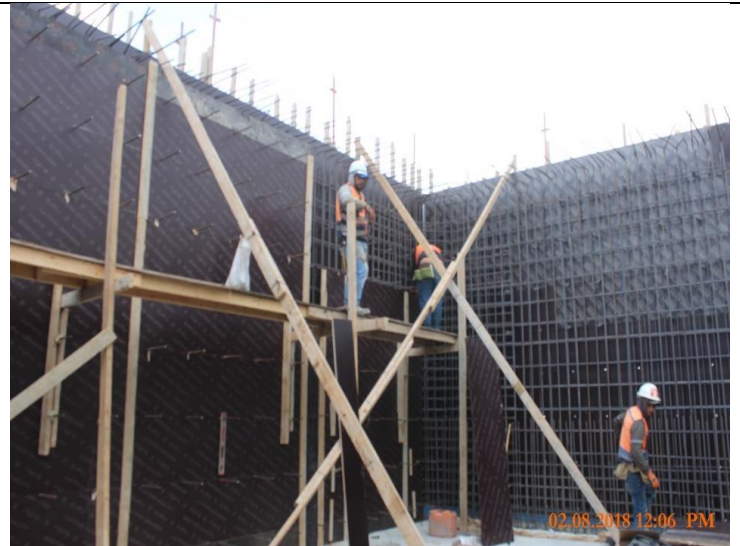
Photo #04 – Steel Reinforcement for Reservoir’s Walls
