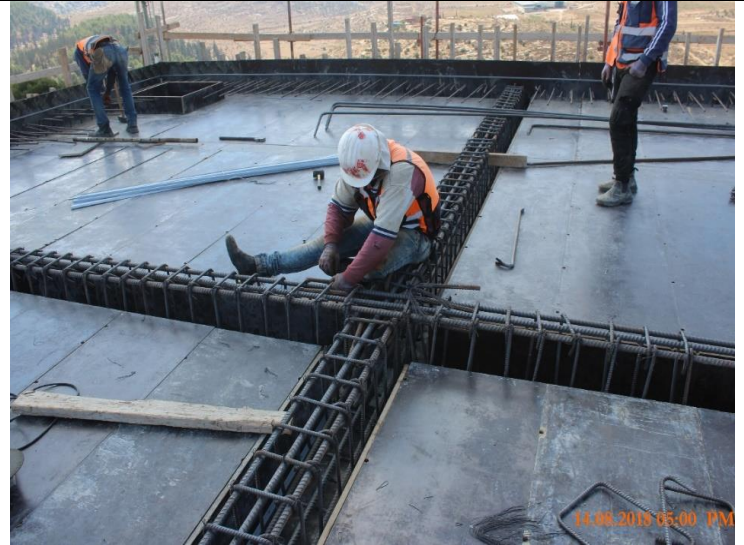
Photo #30 – Steel Reinforcement for the Reservoir’s Top Slab
