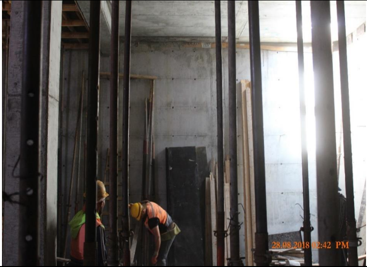
Photo #53 – Formwork De-Shuttering
