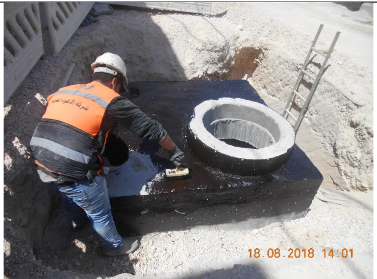
Photo #44 – External Coating for the Pre-cast Manhole
