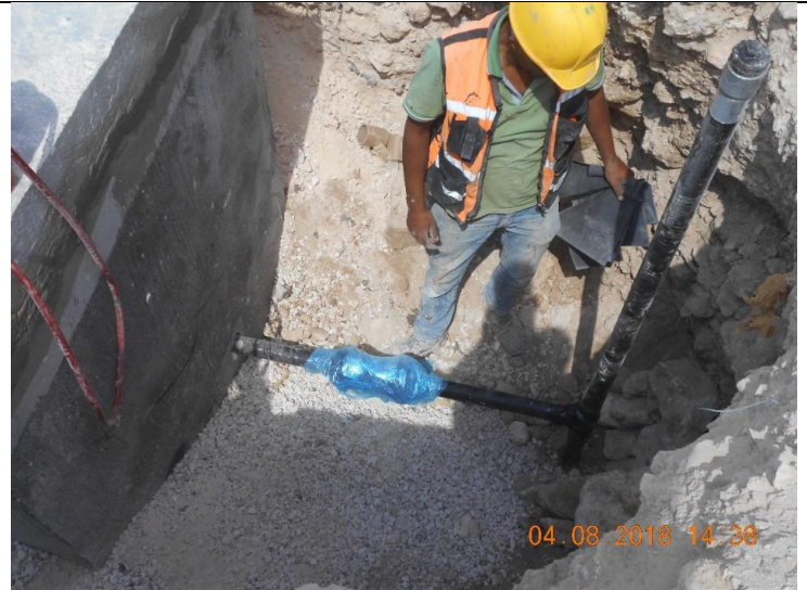
Photo #08 – Connections for Pre-Cast Washout Manhole
