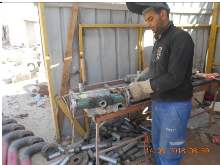
Photo #33 – Fabrication of Fittings
