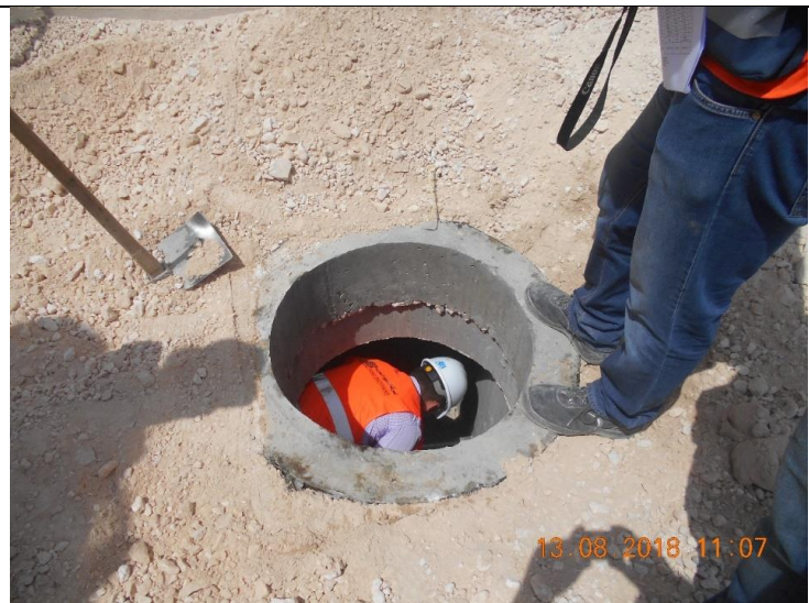
Photo #27 – Inspection of Flange Welding by CWI inside Pre-cast Gate Valves
