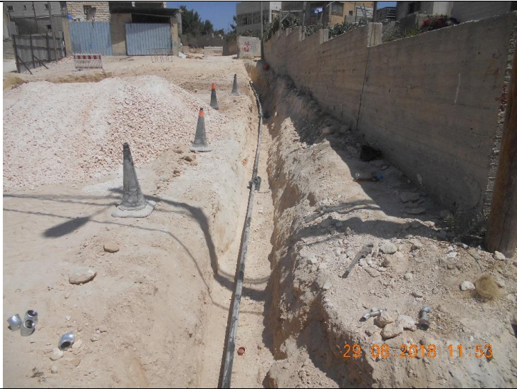
Photo #55 – Pipeline Installation
