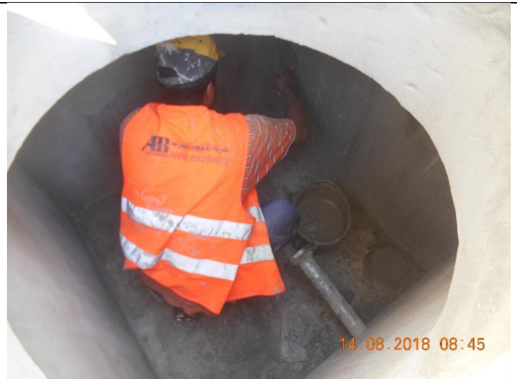
Photo #32 – Internal Concrete Repair for the Pre-Cast Manholes
