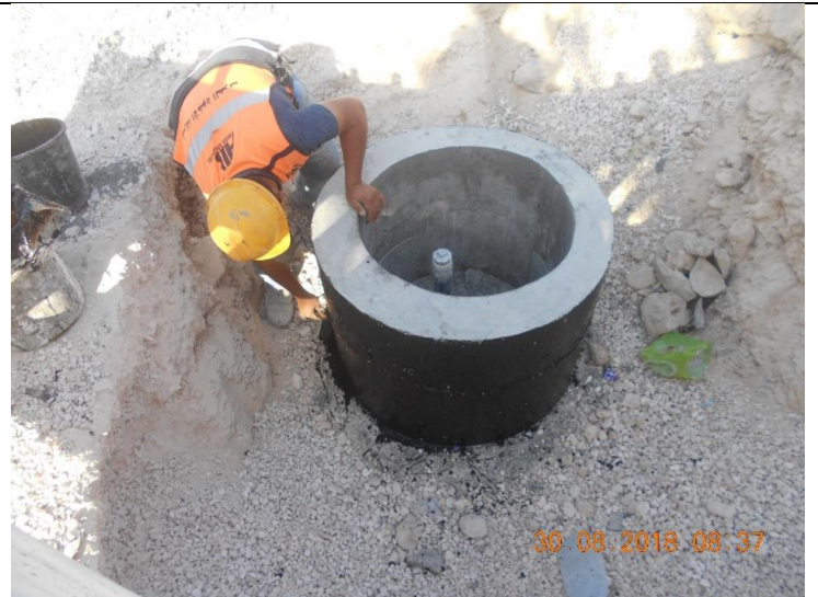
Photo #58 – External Coating for Washout Urban
