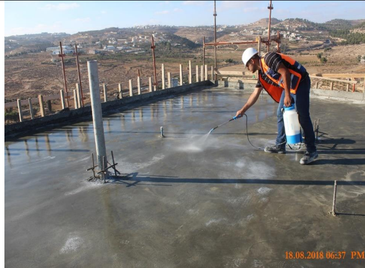
Photo #04 – Concrete Curing for the Reservoir’s Top Slab
