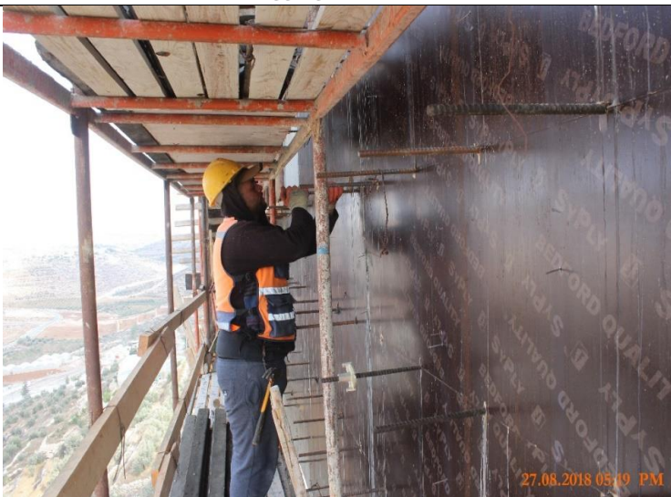
Photo #51 – Formwork De-Shuttering
