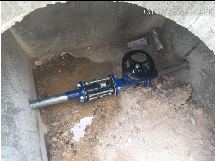
Photo #07 – Installation of 2" Gate Valve
