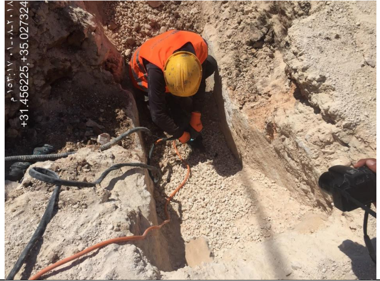
Photo #02 – Anode Installation along Alignment KAR-1
