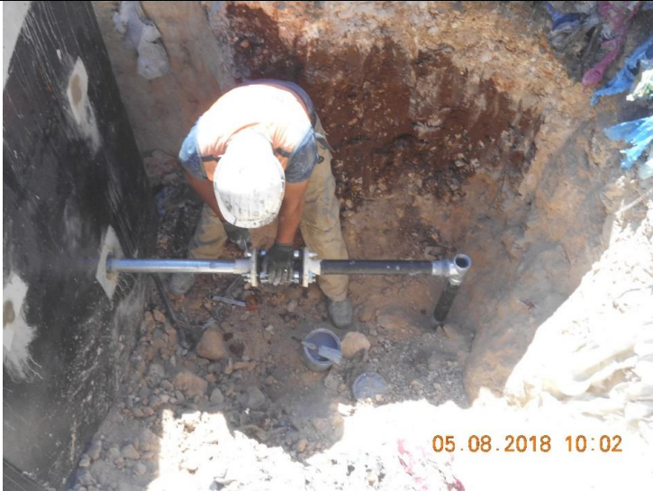
Photo #11 – Connections for Pre-Cast Washout Manhole
