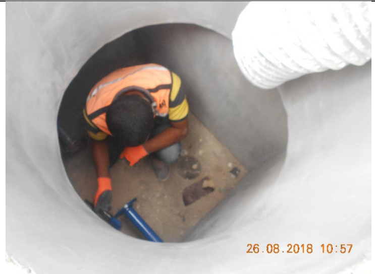
Photo #50 – Epoxy Paint for Pipes
