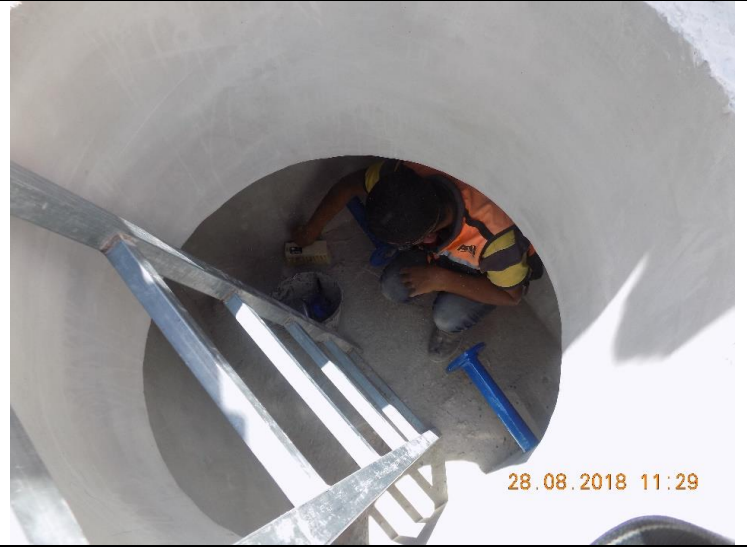
Photo #54 – Epoxy Paint for Pipes
