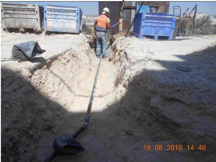
Photo #45 – Installation of Future House Connections
