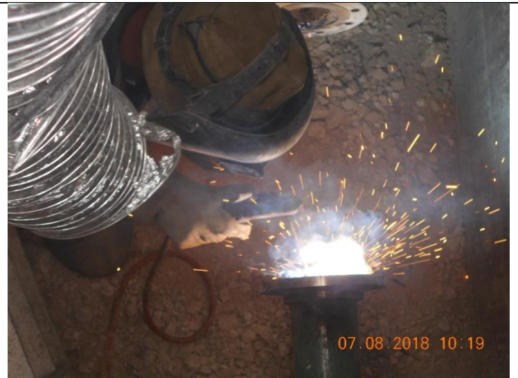
Photo #14 – Welding Flanges inside Chambers
