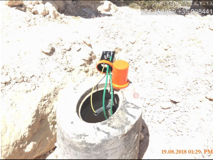
Photo #47 – Installation of Test Station at KAR-1 at Sta. 0+250
