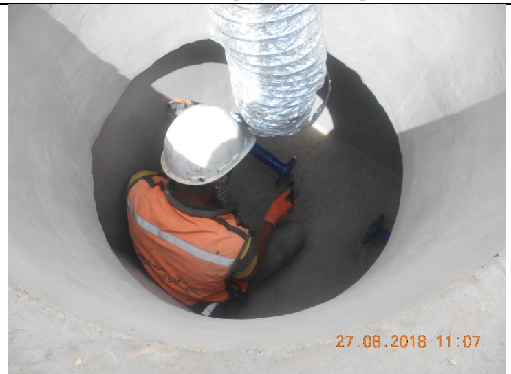
Photo #52 – Epoxy Paint for Pipes
