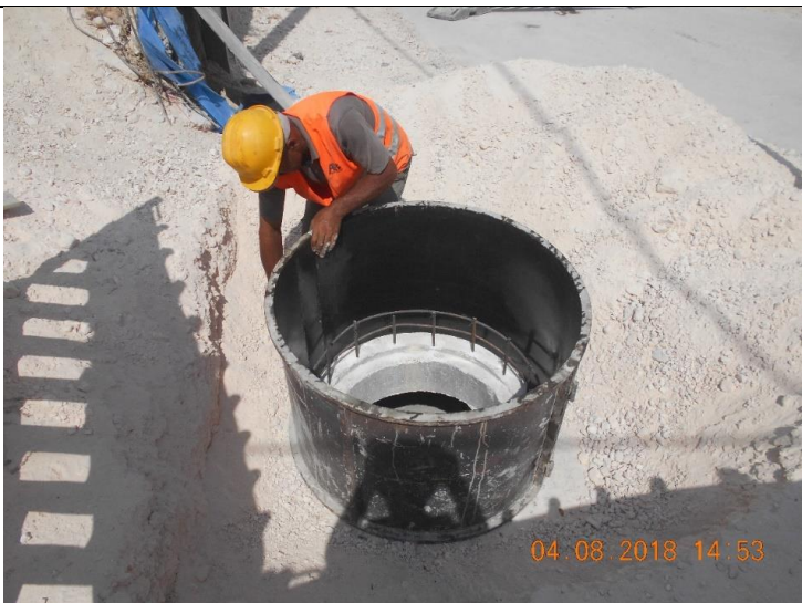
Photo #09 – Neck Extension for Precast Manhole
