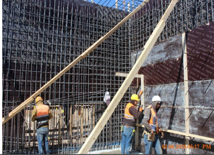
Photo #01 – Formwork for Reservoir’s Walls
