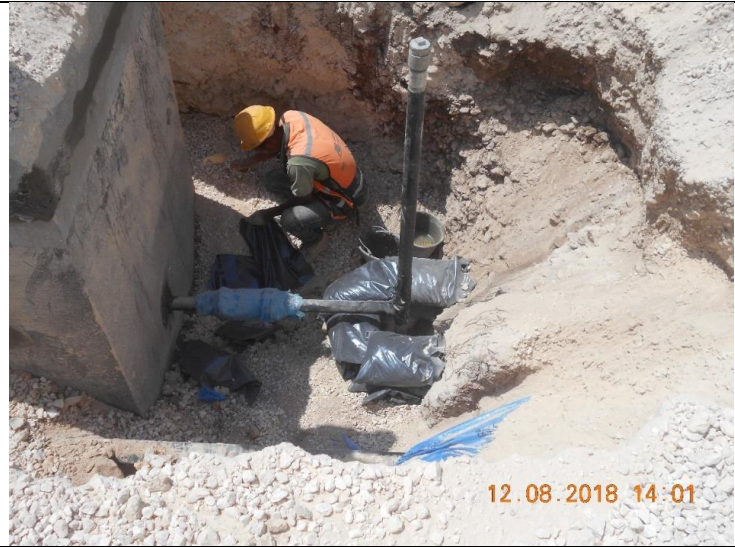
Photo #25 – Installation of Washout Outfall
