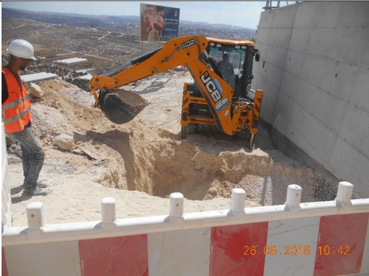
Photo #49 – Digging for Pre-Cast Manholes
