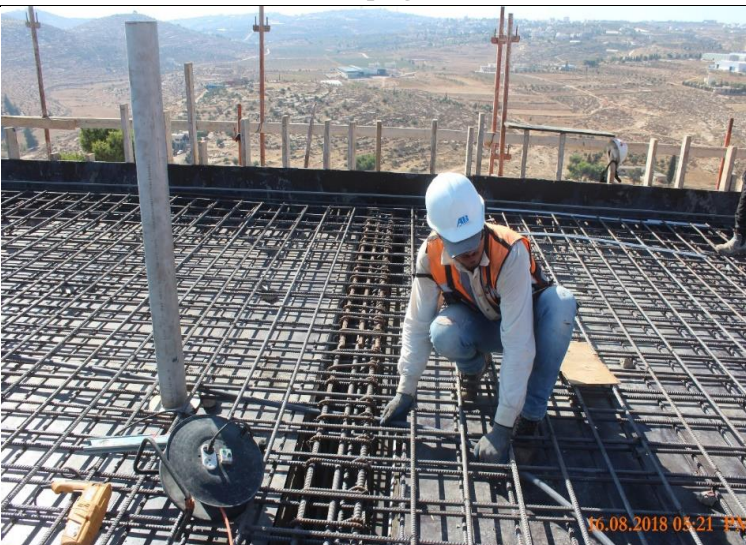
Photo #39 – Electrical Works for the Reservoir’s Top Slab
