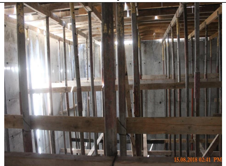
Photo #34 – Formwork for the Reservoir’s Top Slab
