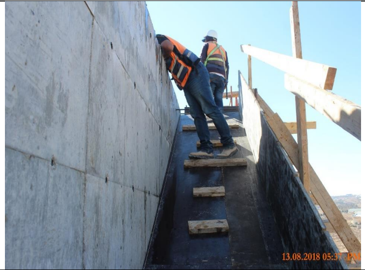
Photo #26 – Formwork for the Reservoir’s Stair Case
