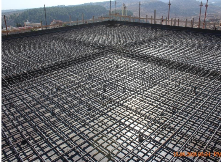
Photo #35 – Steel Reinforcements for the Reservoir’s Top Slab
