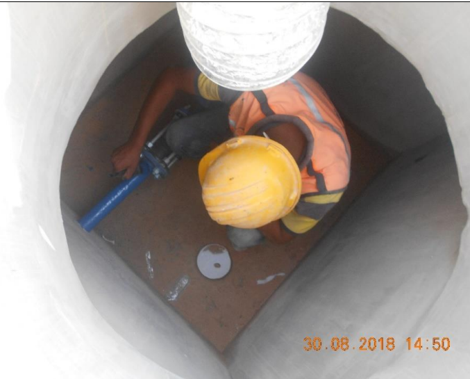
Photo #57 – Epoxy Painting for Steel Flanges and Pipes
