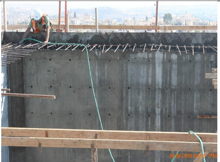
Photo #02 – Concrete Curing for the Reservoir's Walls
