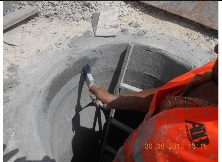
Photo #56 – Concrete Repair for Pre-Cast Manholes
