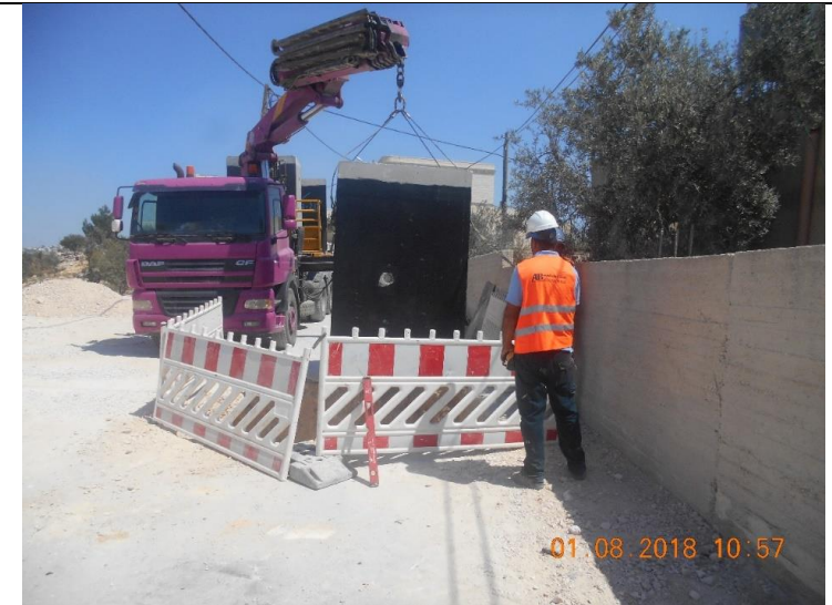
Photo #03 – Pre-Cast Manhole Installation
