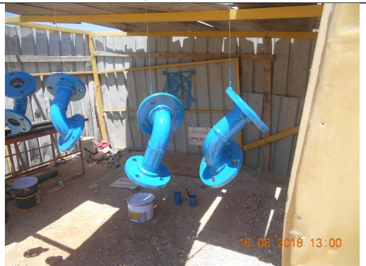
Photo #40 – Epoxy Coating for Fittings
