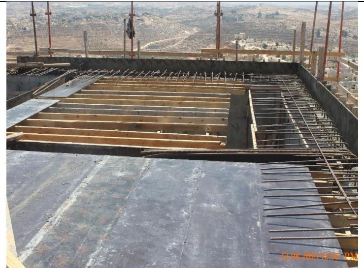
Photo #22 – Formwork for Reservoir's Top Slab
