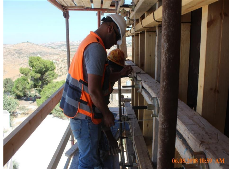
Photo #12 – Inspecting Formwork for the Reservoir's Walls
