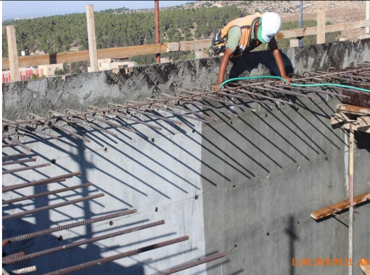
Photo #03 – Concrete Curing for the Reservoir’s Walls
