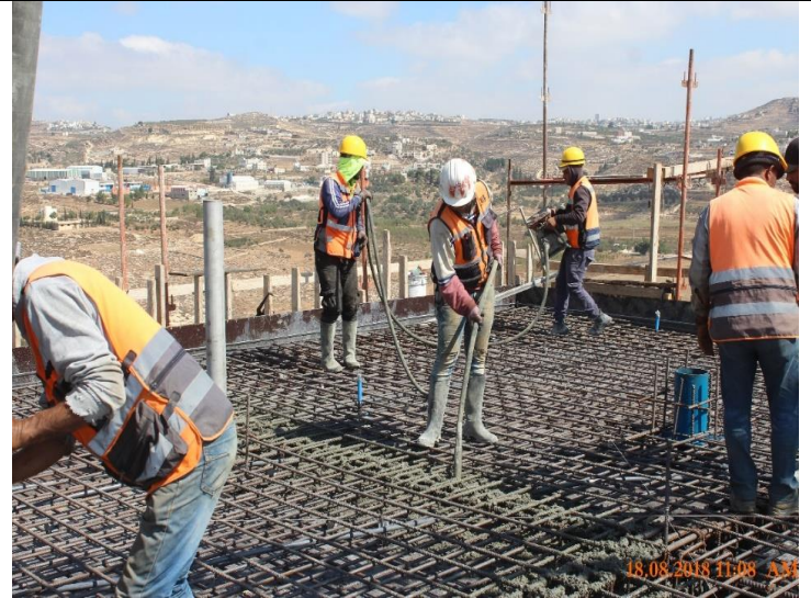
Photo #42 – Casting Concrete for the Reservoir's Top Slab
