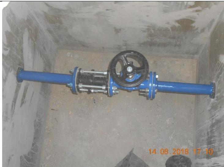
Photo #31 – Mechanical Work and Gate Valve Installation
