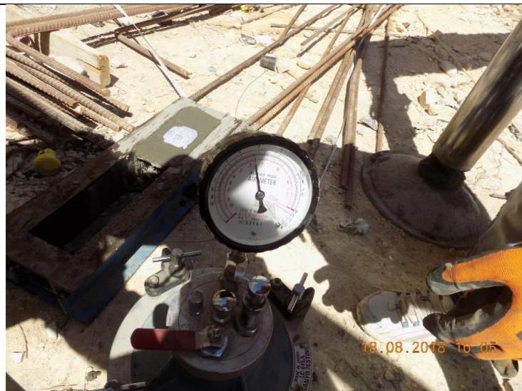
Photo #05 – Concrete Test
