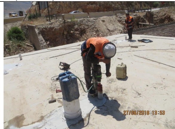
6. Conducting Core test for Box culvert slab (Part-1) @Sta.3+031.
