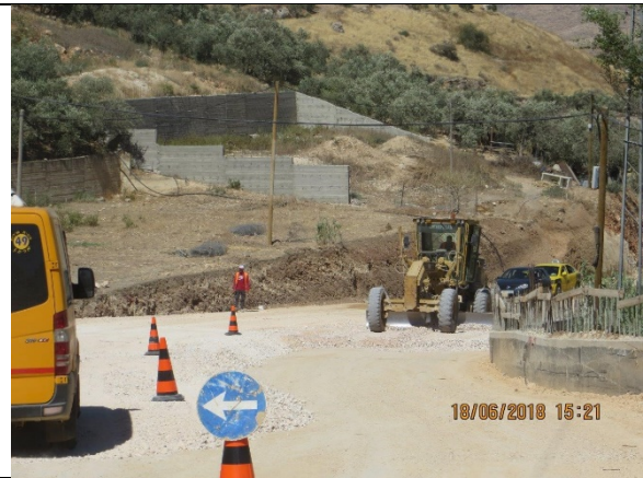
20. Start delivering and mixing Topping 4th layer from Sta.0+290 to Sta.0+320.
