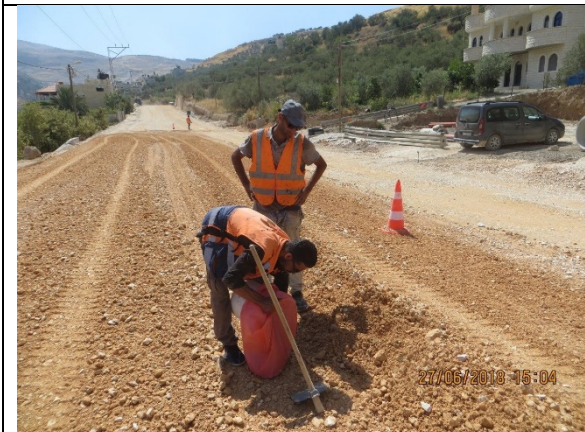
5. Conducting comprehensive test for basecourse final layer from Sta.0+990 to Sta.1+400.
