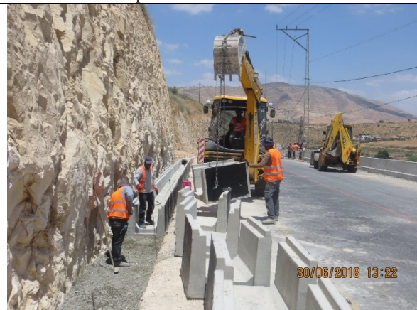
24. Start installing and fixing open channel from Sta.1+880 to Sta.1+780.
