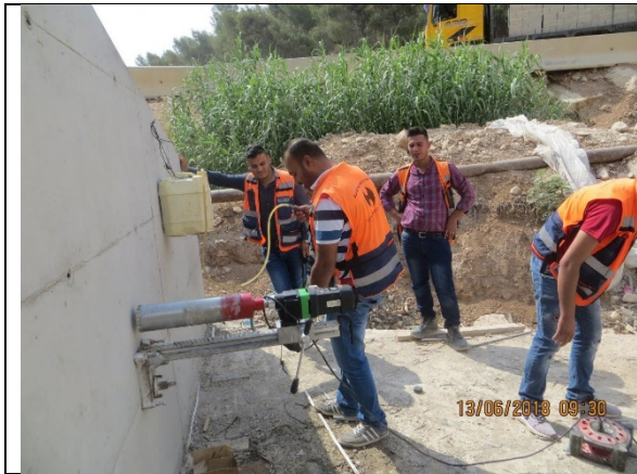
7. Conducting Core test for casted concrete B300 for Box culvert wings @ 3+031.
