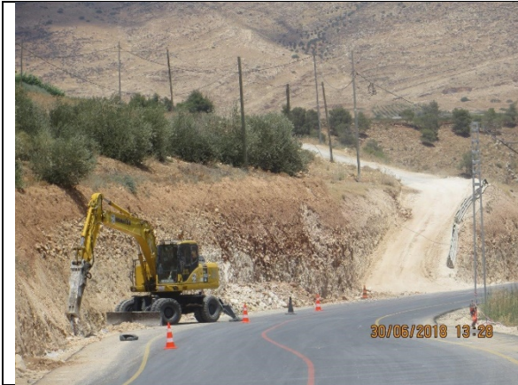
13. Excavation works for open channel from Sta.2+350 to Sta.1+880.
