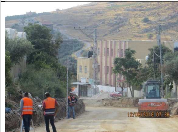
15. Handing over replacement 2nd layer (A-2-4) from Sta.0+080 to Sta.0+200.
