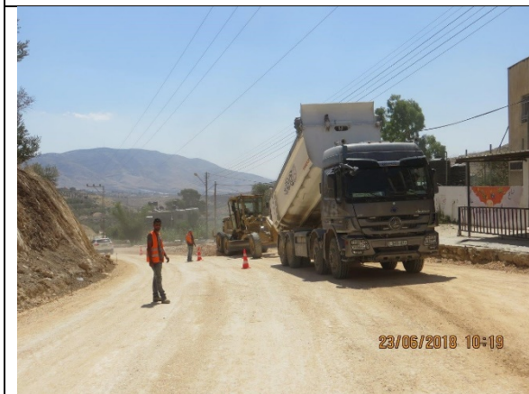
21. Start delivering and spreading Subbase 2nd layer from Sta.0+080 to Sta.0+290.
