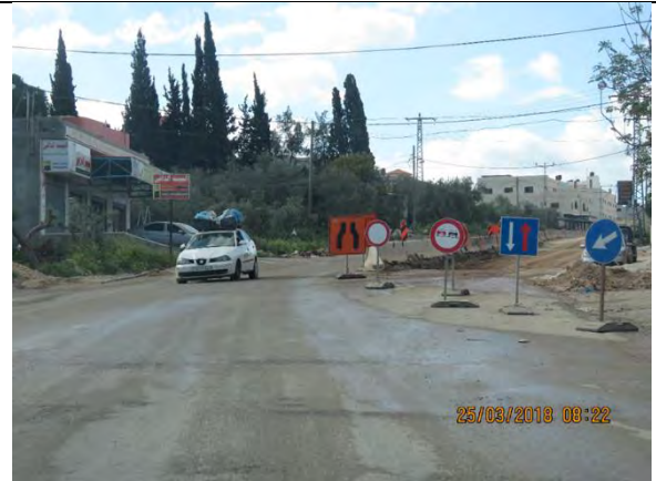
Photo 26: Applying safety measures
