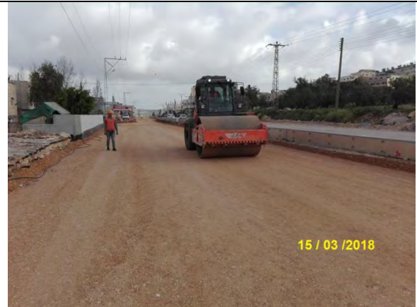
Photo 18: Compacting 3rd replacement layer from Sta. 0+430-0+540 LHS
