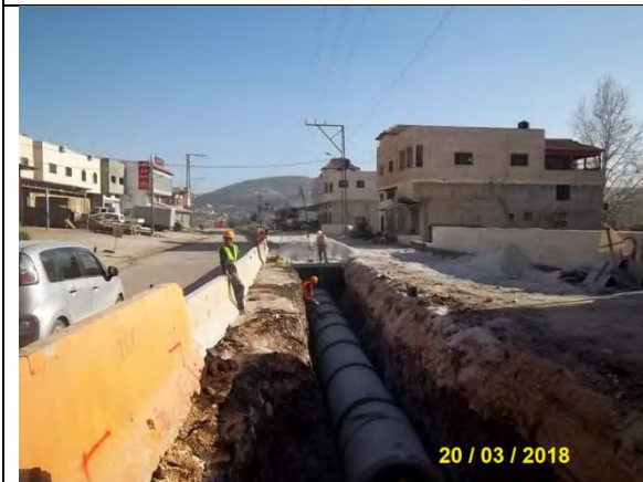
Photo 23: Installation of Storm Water pipeline from MH 15 to MH # 16
