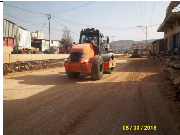
Photo03: Compacting 1st replacement layer 0+283-0+430LHS
