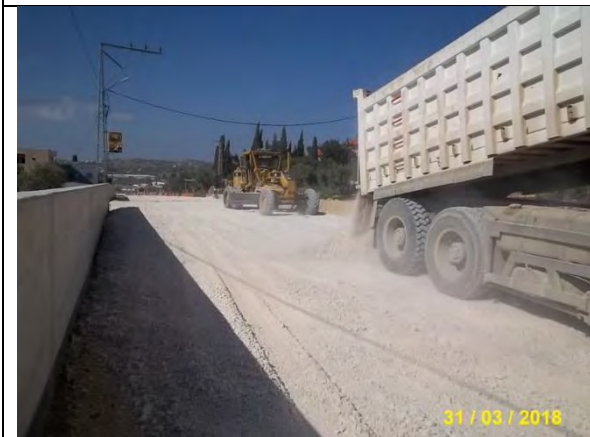
Photo 33: Delivering, grading base course layer from Sta. 0+820-0+980 LHS
