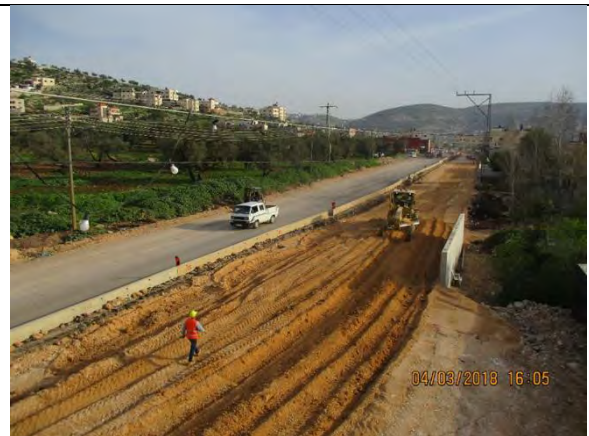
Photo 02: Grading 3rd replacement layer from Sta. 0+540-630 LHS
