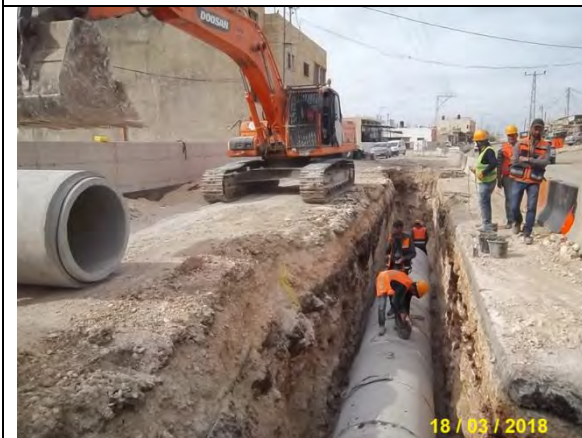
Photo 21: Installation of storm water pipeline from Sta. 0+188.45-0+217.03 LHS
