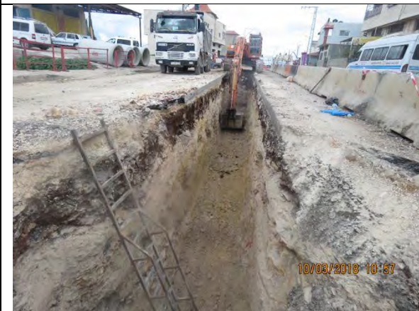
Photo 09: Excavation works for Storm water pipeline from Sta. 0+107-0+136
