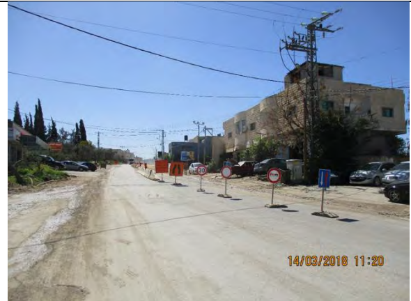
Photo 14: Implementation traffic safety plan from Sta. 0+980-1+080 LHS
