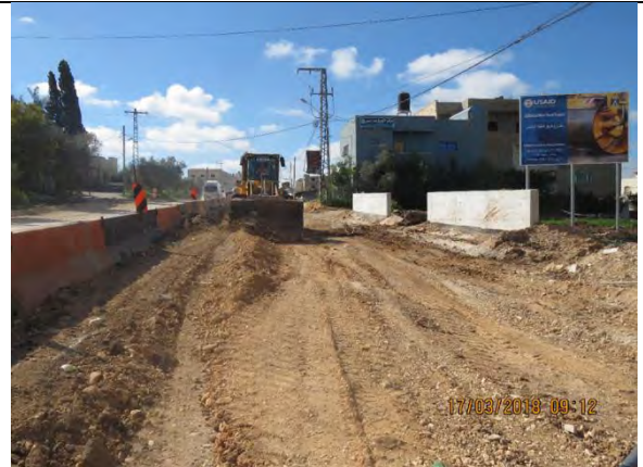
Photo 20: Road excavation from Sta. 0+980-1+080 LHS
