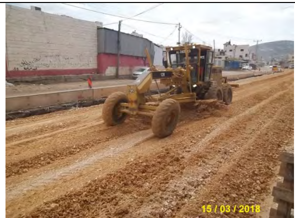
Photo 16: Grading 1st sub base layer from Sta. 0+290-0+430 LHS
