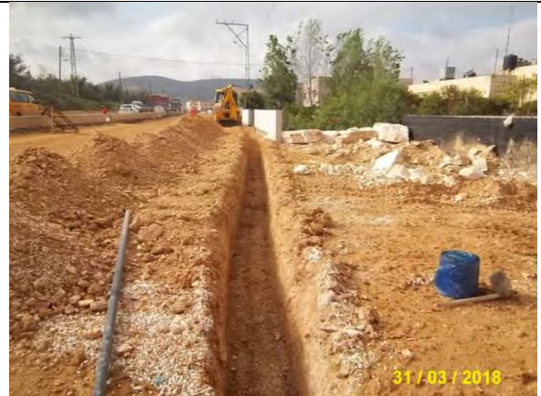
Photo 32: Excavation works for 2" water pipeline from Sta. 0+430-0+580 LHS
