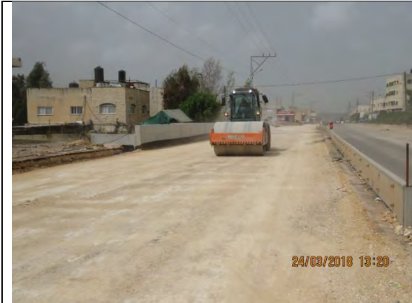
Photo 25: Compacting 1st sub base Layer from Sta. 0+430-0+540 LHS
