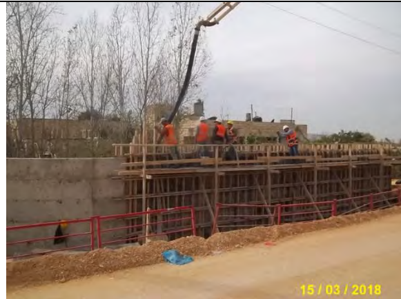
Photo 17: Casting concrete for RW stem wall from Sta. 0+535-0+545 LHS
