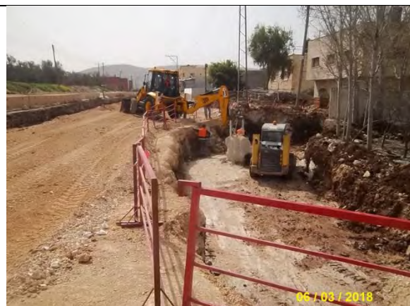
Photo 05: Excavation works for RW foundation from Sta. 0+525-0+545 LHS
