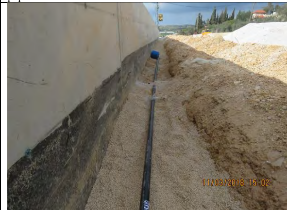
Photo 11: Installation of 2" water pipeline from Sta. 0+669-0+834LHS
