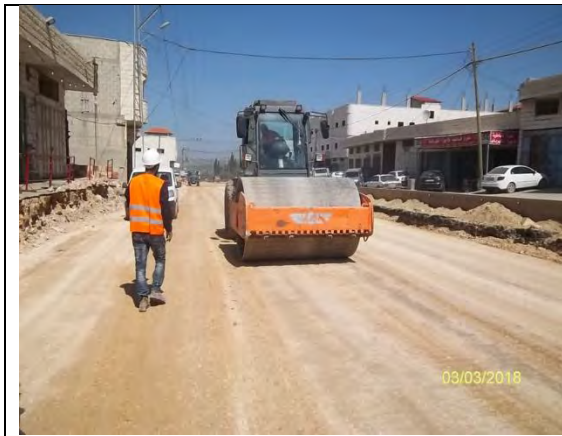
Photo 01: Compacting 3rd replacement layer from Sta. 0+640-0+775 LHS
