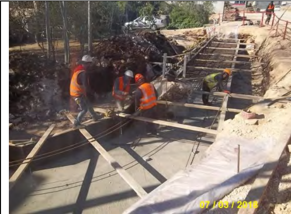
Photo 07: Formwork, steel reinforcement for RW foundation from Sta. 0+525-0+545 LHS
