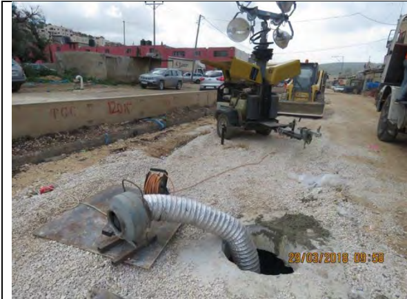
Photo 31: Cleaning and concrete benching for storm water manholes
