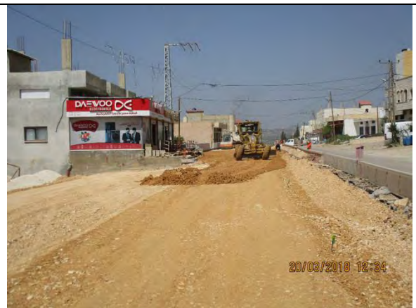
Photo 22: Grading 2nd sub base layer from Sta. 0+540-0+640 LHS
