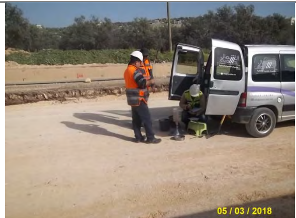
Photo04: QC-conduct field density test 1st replacement 0+430-0+540 LHS
