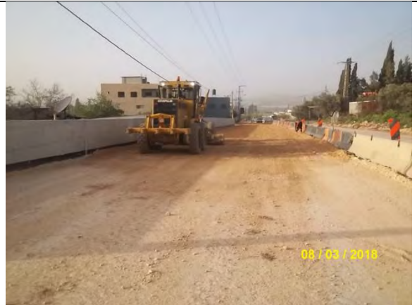
Photo 08: Grading 2nd sub-base 0+920-0+980
