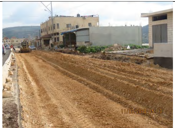
Photo 12: Grading 2nd replacement layer from Sta. 0+430-0+540 LHS
