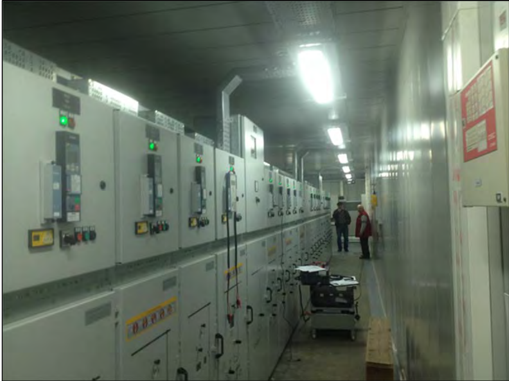
Installation of switchgears at Gardbani Substation
