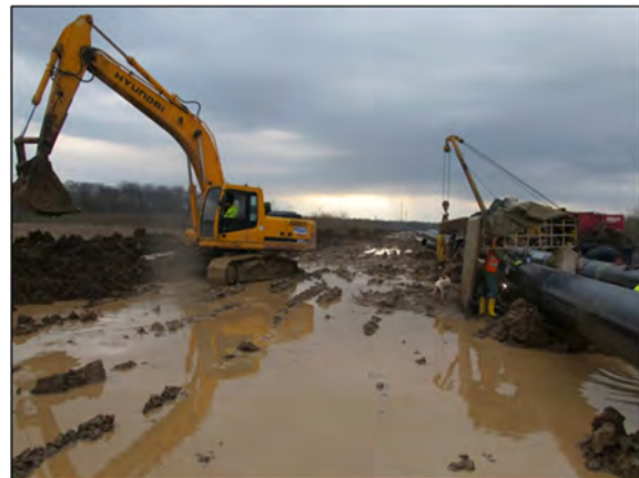
Welders working on a pipeline segment, Zestaphoni-Kutaisi
