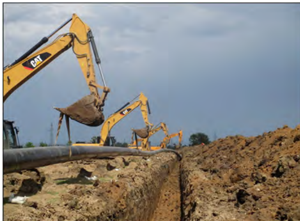
Pipeline lowering using excavators, Zestaphoni-Kutaisi pipeline segment
