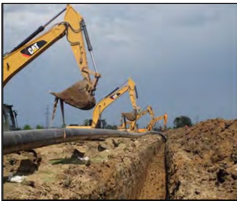
Pipe segments being lowered into an open cut trench, Zestaphoni-Kutaisi segment
