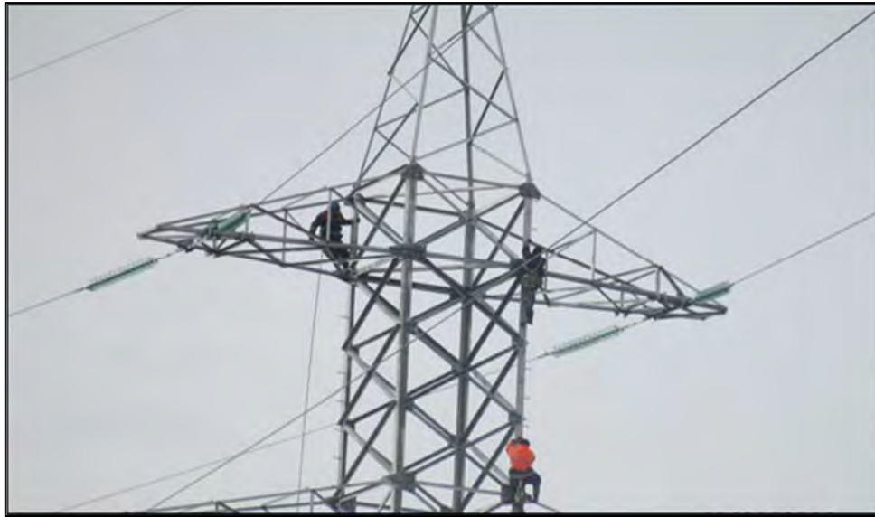
Workmen constructing a 220 kV tower in the Imereti Region
