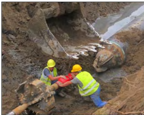
Horizontal directional drilling of the Rioni River, Kutaisi-Abasha pipeline segment
