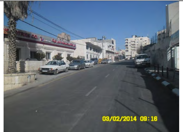
Road marking and curbside paint finished – Road #7 at St. 0+100
