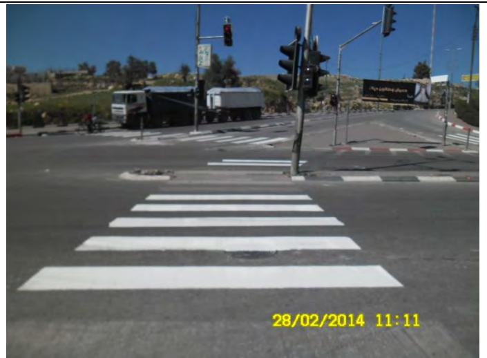
Road marking - Al Salam Road
