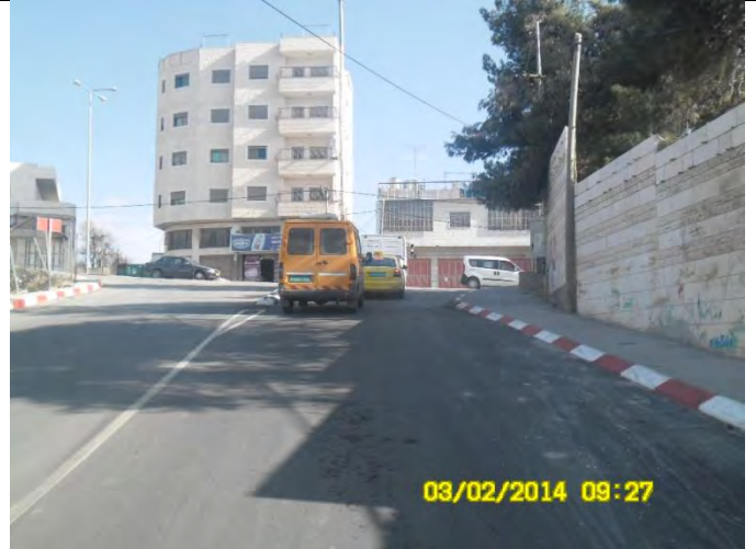
Road marking and curbside paint finished – Road #7 at St. 0+550
