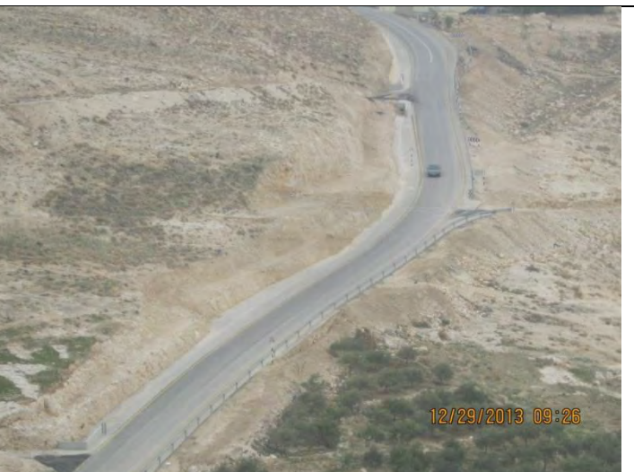
After finishing construction – From St. 0+200 to St. 0+500
