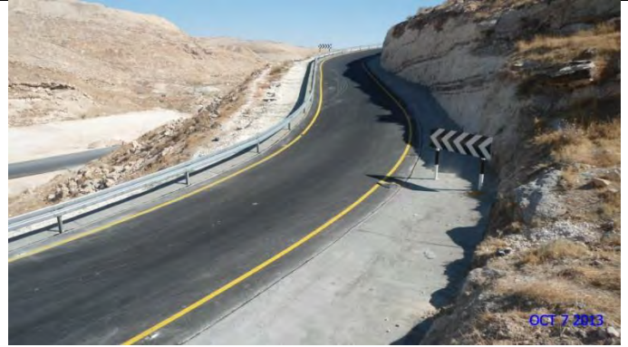
After finishing construction – From St. B0+200 to St. B0+250
