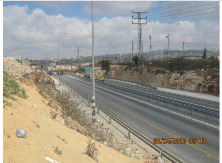
Project completed– New Guardrail installed at the C.L, road marking and cat eyes were installed and finished.
