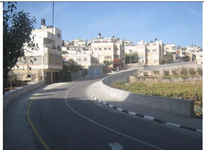
After finishing construction – Segment A – at St. 0+040 LHS
