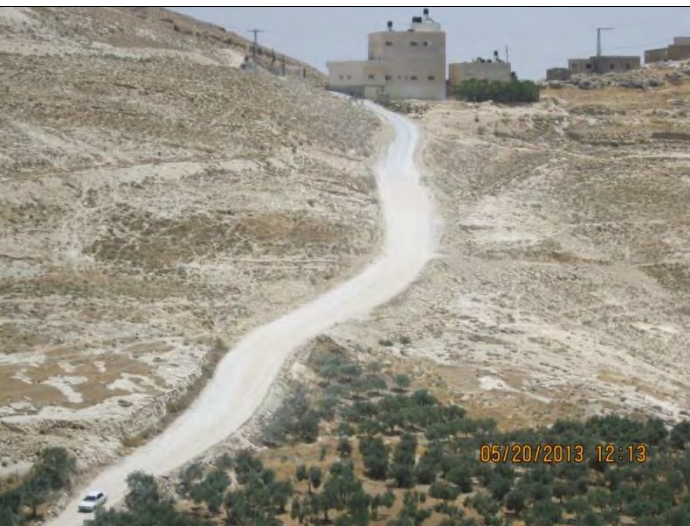
Before construction – From St. 0+200 to St. 0+500
