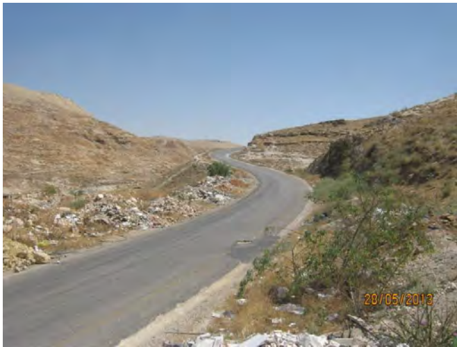
Before construction – From St. A0+220 to St. A0+460
