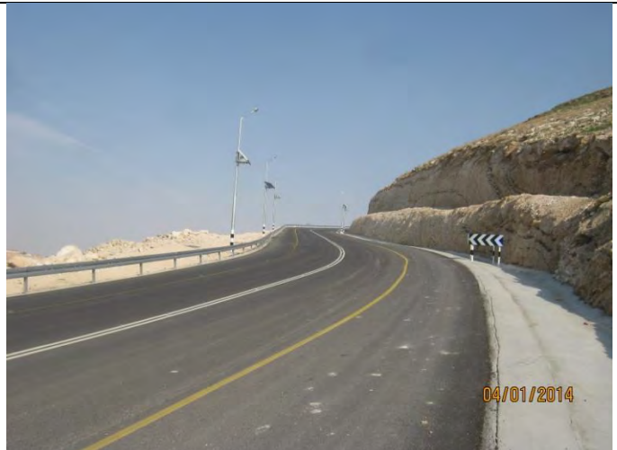
After finishing construction.
