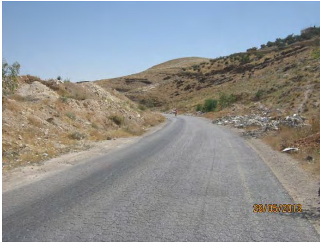
Before construction – From St. A0+120 to St. A0+220
