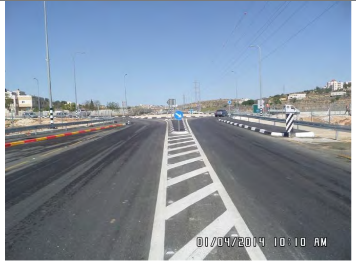
Beit Enon- St. A0+070- After completion construction works.
