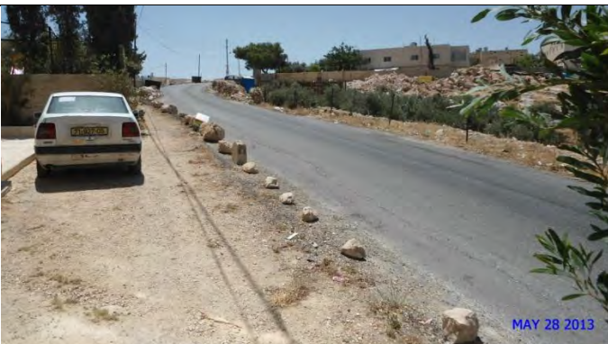
Before construction – From St. B0+840 to St. B0+920
