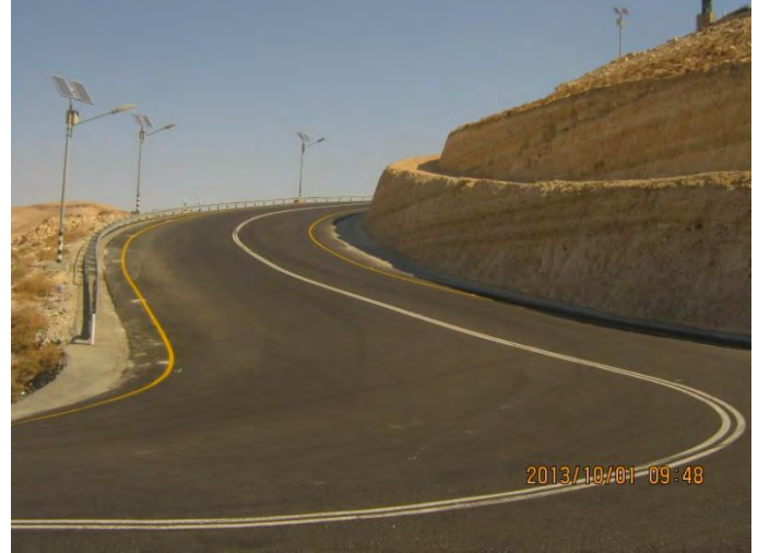
Project completed – New Guardrail installed, road marking and cat eyes were installed and finished – St. 0+170 Forward.
