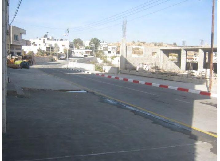
After finishing construction – Segment A – at St. 0+440 LHS
