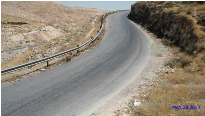
Before construction – From St. B0+200 to St. B0+250
