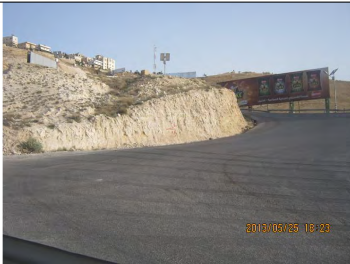
Before construction – St. 0+325 Forward.
