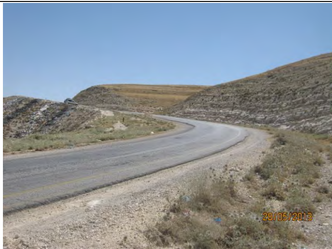
Before construction – From St. A1+100 to St. A1+300
