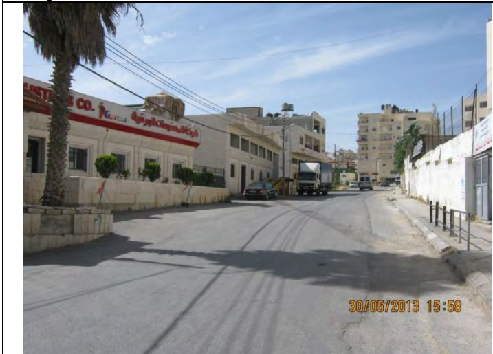
Before Milling – Road #7 at St. 0+100
