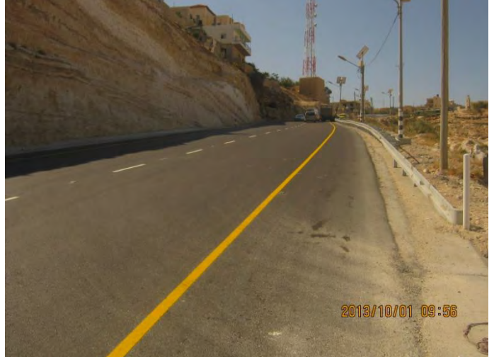
Project completed – New Guardrail installed, road marking and cat eyes were installed and finished – St. 0+787 Forward.
