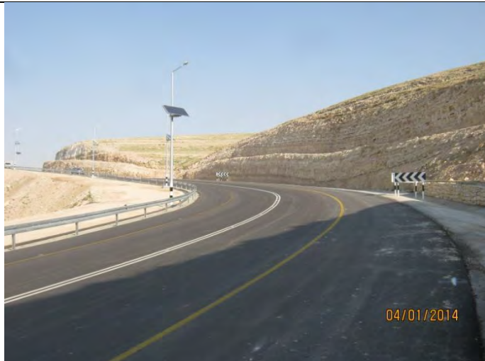
After finishing construction.
