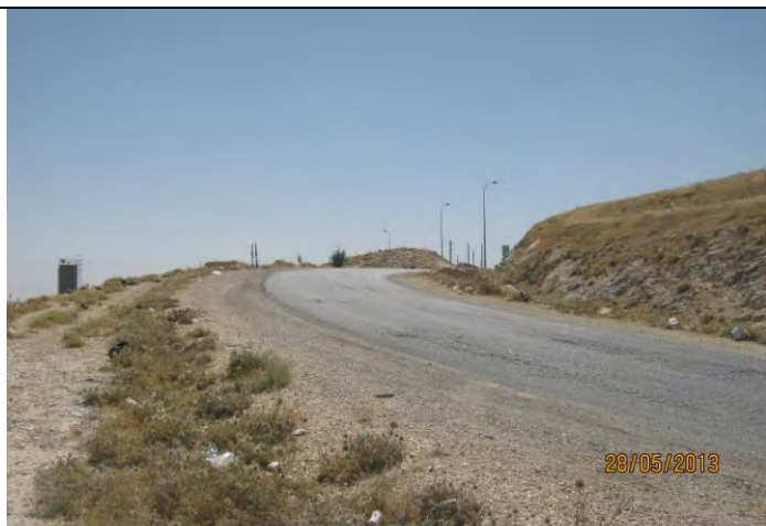
Before construction – From St. A1+300 to St. A1+420
