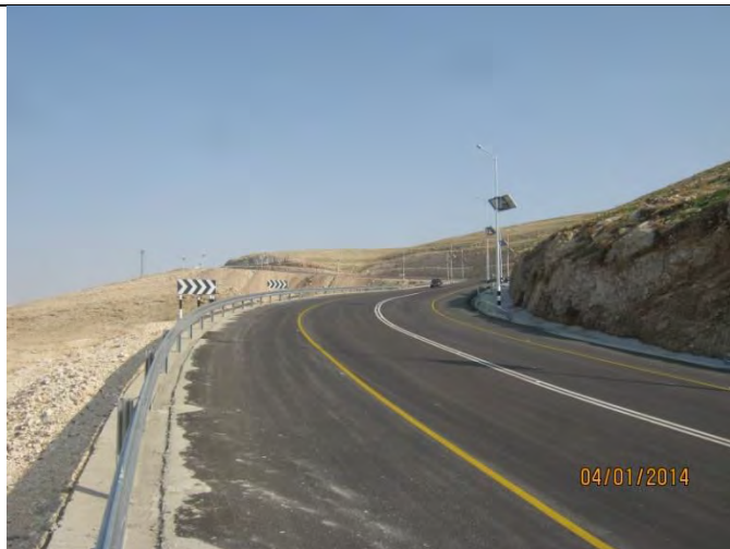
After finishing construction.
