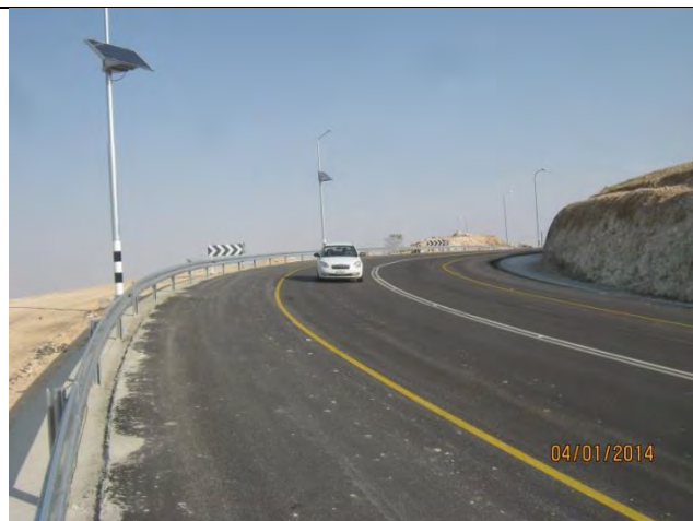
After finishing construction.
