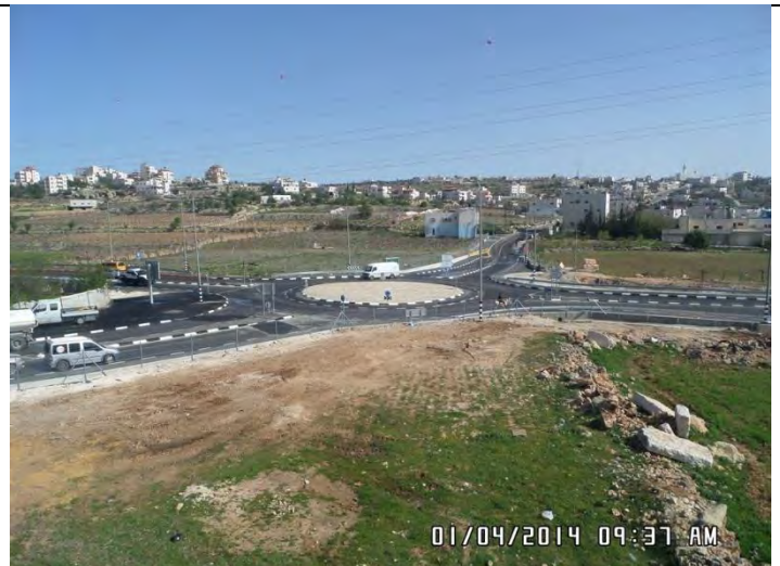
Beit Enon Roundabout – After completion construction works.
