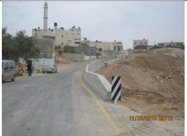
After finishing construction – From St. 0+936 to St. 1+057
