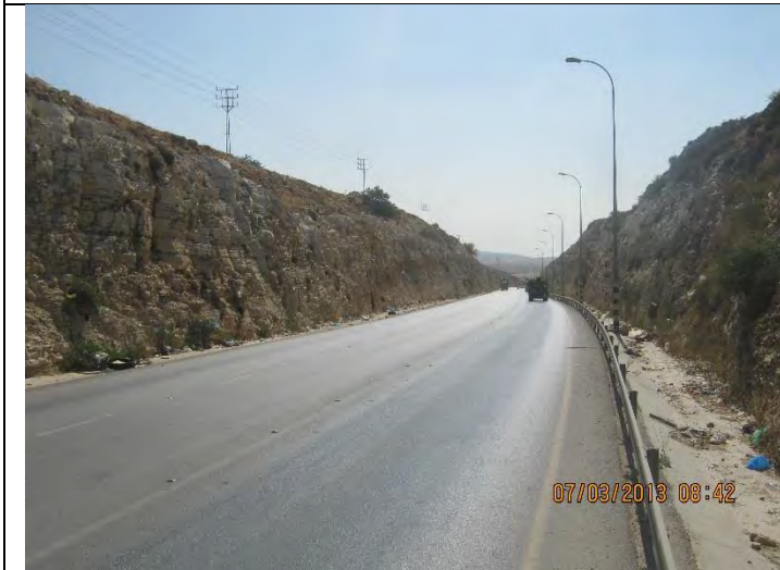
Before construction –St. 1+600 forward.
