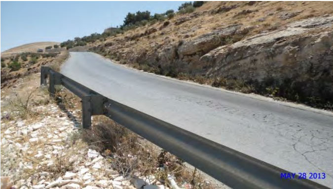
Before construction – From St. B0+250 to St. B0+330
