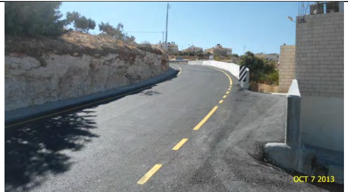
After finishing construction – From St. B0+560 to St. B0+680
