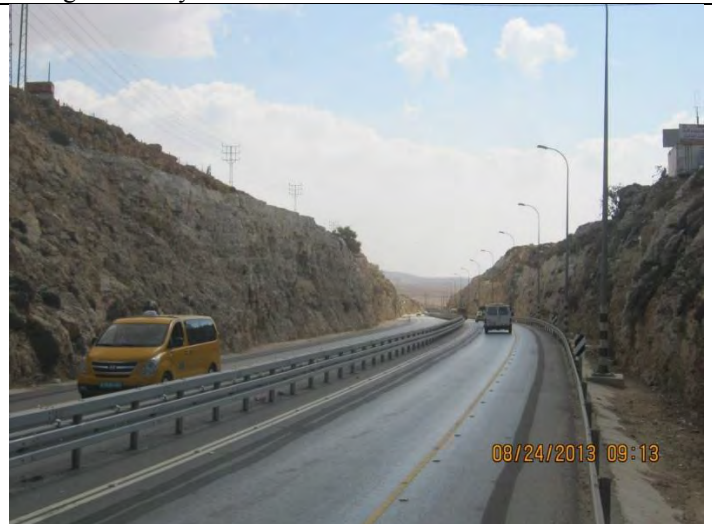
Project completed – New Guardrail installed at the C.L, road marking and cat eyes were installed and finished.
