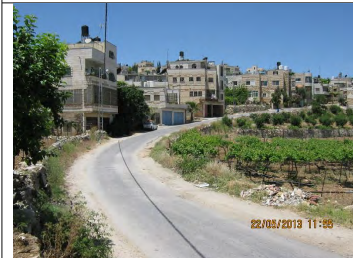
Before construction – Segment A – at St. 0+040 LHS
