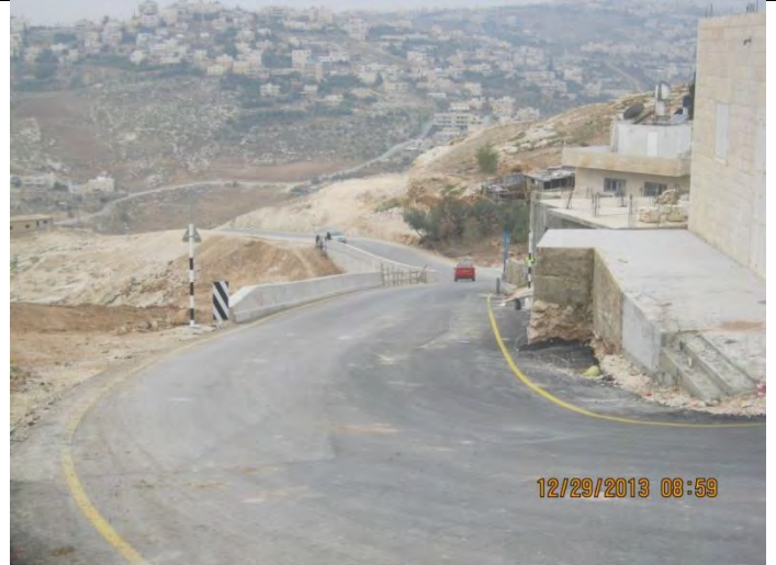
After finishing construction – From St. 0+980 to St. 1+080
