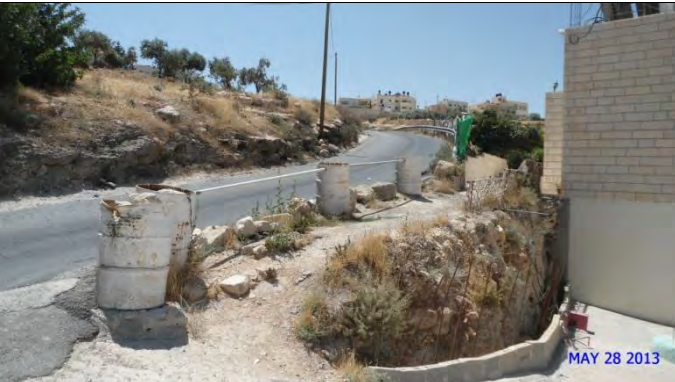
Before construction – From St. B0+560 to St. B0+680
