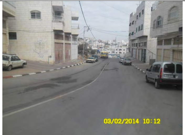
Road marking and curbside paint finished – Road #8 at St. 0+520
