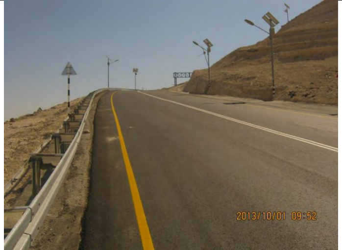
Project completed – New Guardrail installed, road marking and cat eyes were installed and finished – St. 0+480 Forward.
