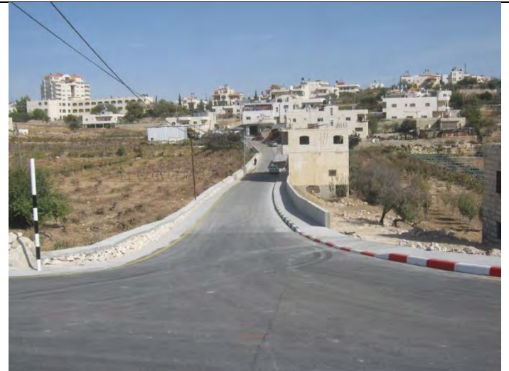
After finishing construction – Segment C – at St. 0+000
