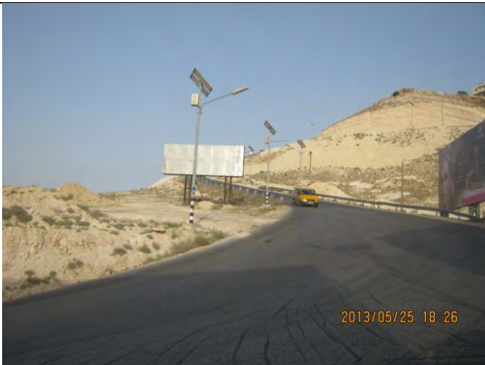
Before construction – St. 0+380 Forward.
