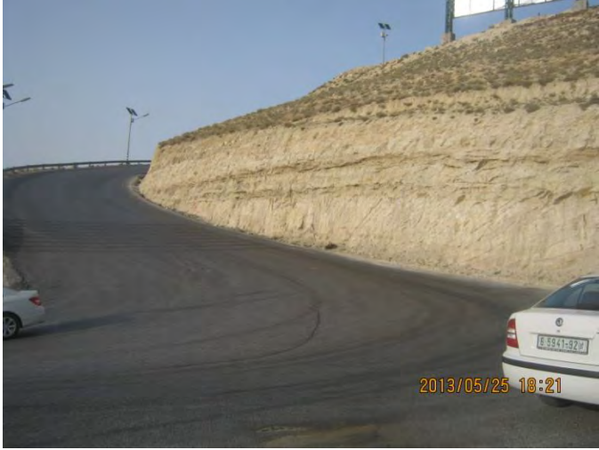
Before construction – St. 0+170 Forward.
