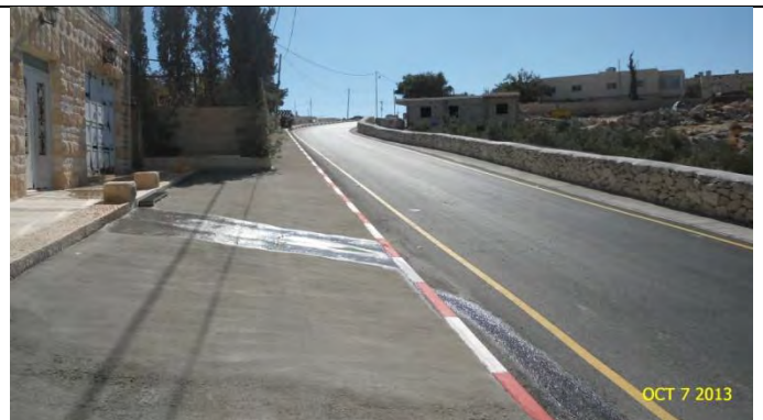
After finishing construction – From St. B0+840 to St. B0+920
