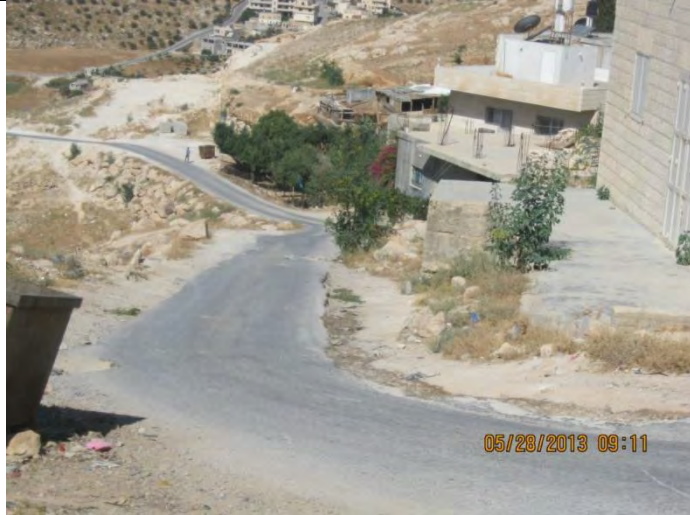
Before construction – From St. 0+980 to St. 1+080
