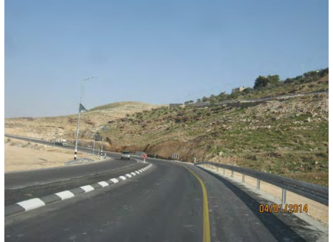
After finishing construction.
