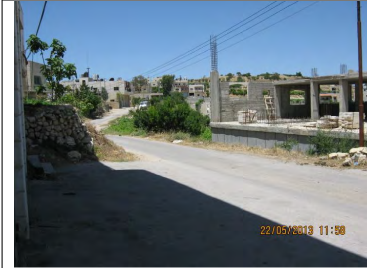
Before construction – Segment A – at St. 0+440 LHS
