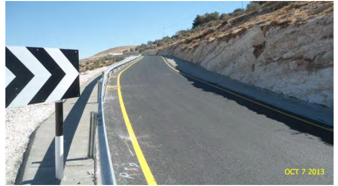
After finishing construction – From St. B0+250 to St. B0+330
