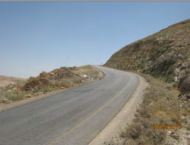
Before construction – From St. A0+600 to St. A0+800
