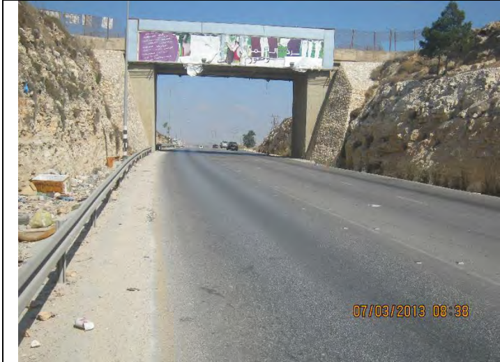
Before construction –St. 1+280 backward.
