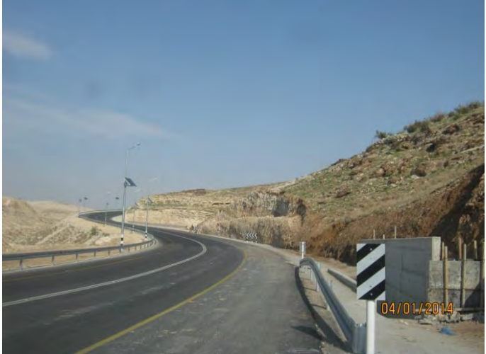
After finishing construction.
