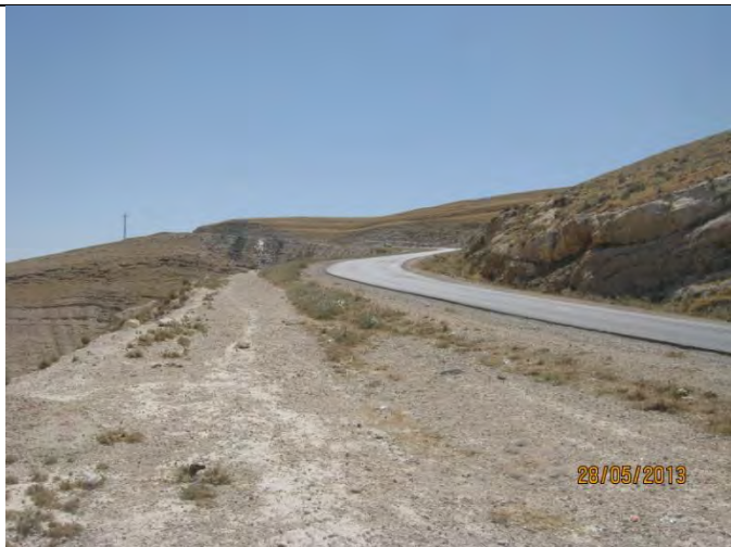
Before construction – From St. A0+800 to St. A1+100
