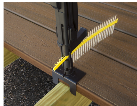
Quik Drive installation of DCU screws.
