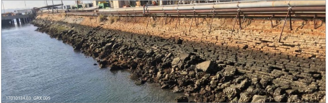
Source: Photograph by Anchor QEA, LLC in 2020.
