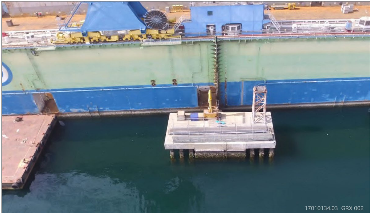
Figure 2-5 View Looking North Showing Existing Dolphin Supporting the Dry Dock
