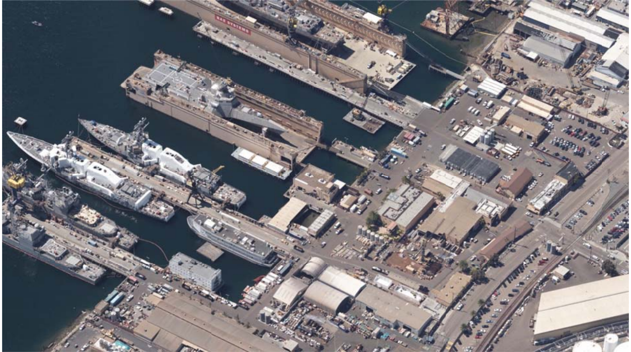
An overview oblique aerial photograph shows the developed nature of the uplands within the study area. The site is nearly fully paved with only the northernmost lot being comprised of a gravel pad.
