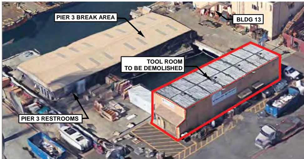
Location of existing tool room to be demolished and incorporated into proposed wharf structure building.
