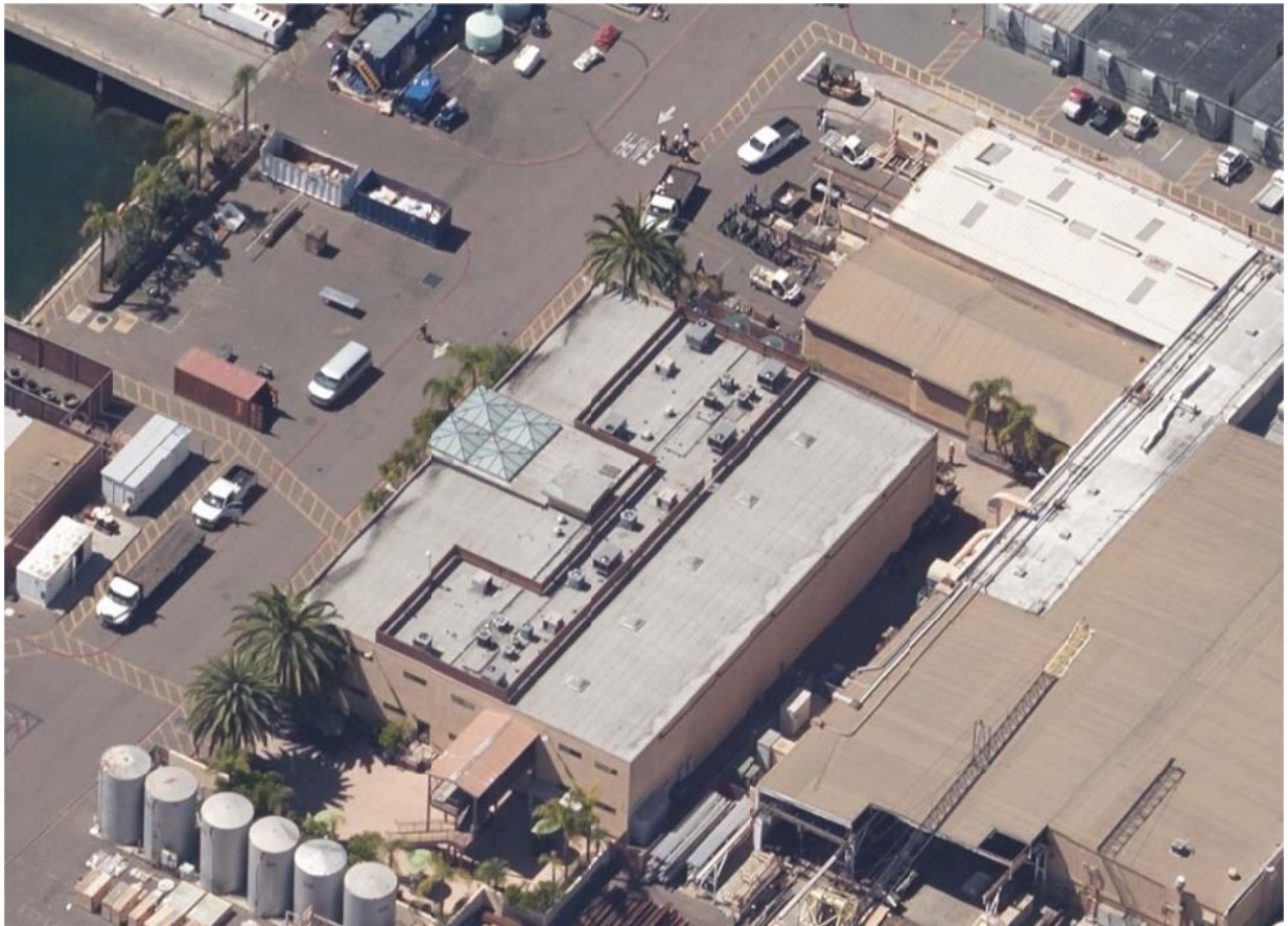
The photograph shows the most extensive collection of vegetated upland area within the shipyard. This consists principally of a variety of palm trees within raised planters.
