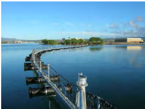
Representative PSB Barrier (float sections spanning waterway)
