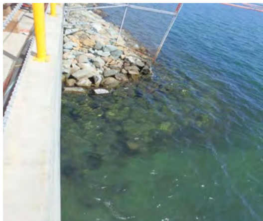
Subsurface and sloped revetment to be removed
