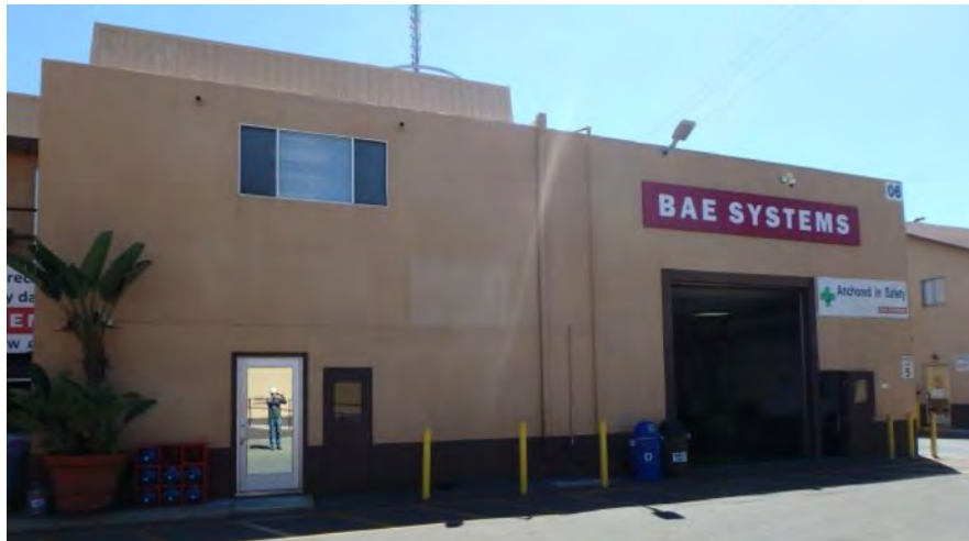
Bldg 6/7 (east) to be demolished in-way-of new prod. bldg.
