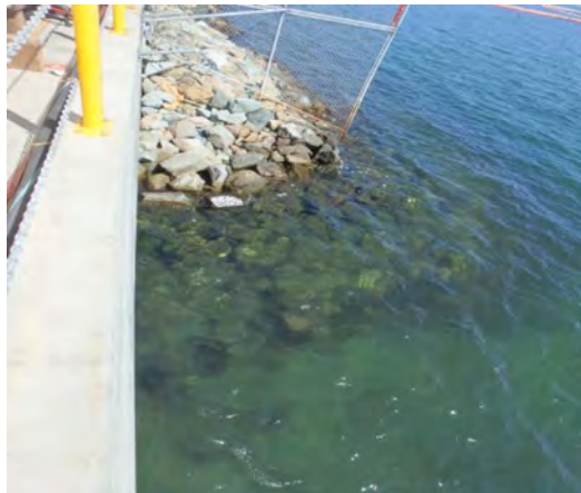
Subsurface and sloped revetment to be removed
