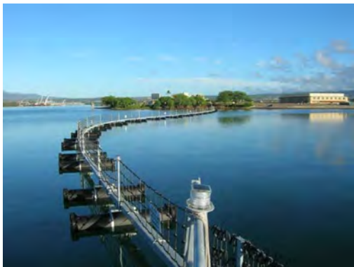
Proposed PSB Barrier (float sections spanning waterway)
