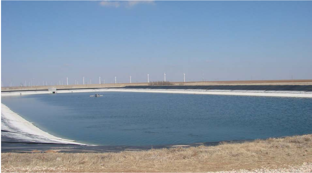
Figure 8.3 – East Wastewater Storage Lagoon
