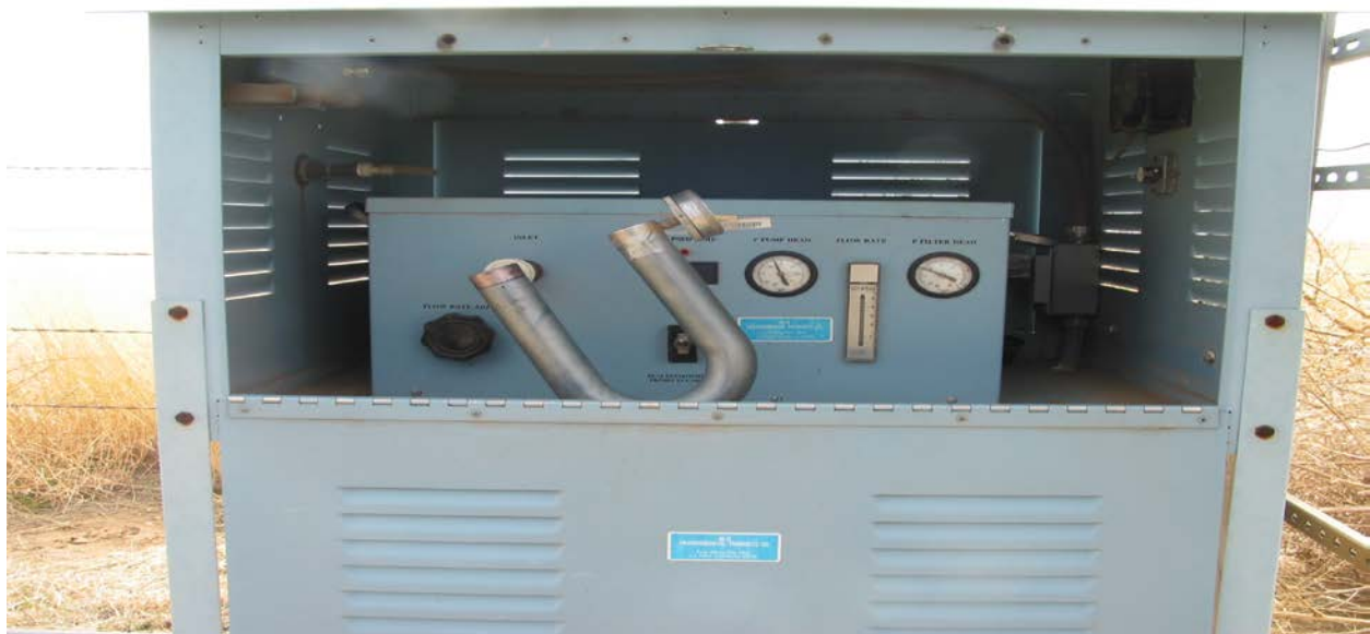
Figure 5.4 – Low-Volume Sampling Apparatus
