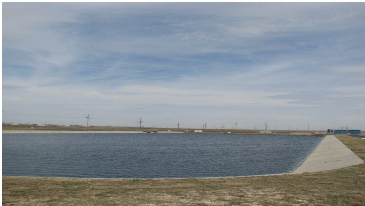
Figure 8.2 – Wastewater Treatment Facility, Facultative Lagoon
