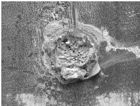
(a) Failure surface on the beam.
