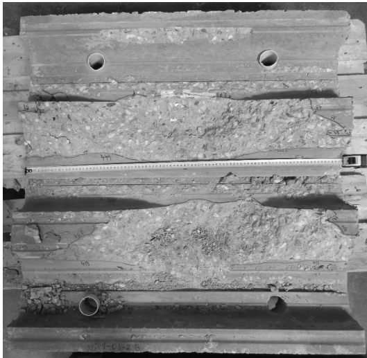
Figure 4.28: Failure cones shown on the slab.
