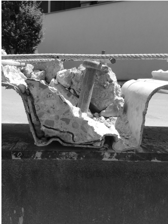
(a) Concrete failure and deformed stud.
