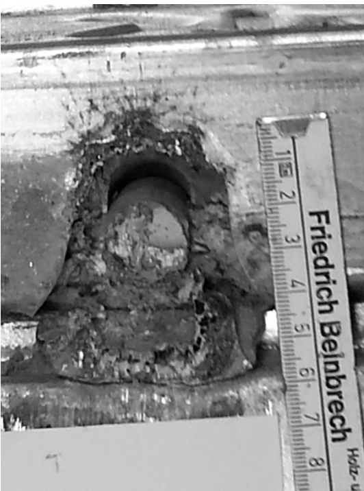
(a) Failure surface on the slab.
