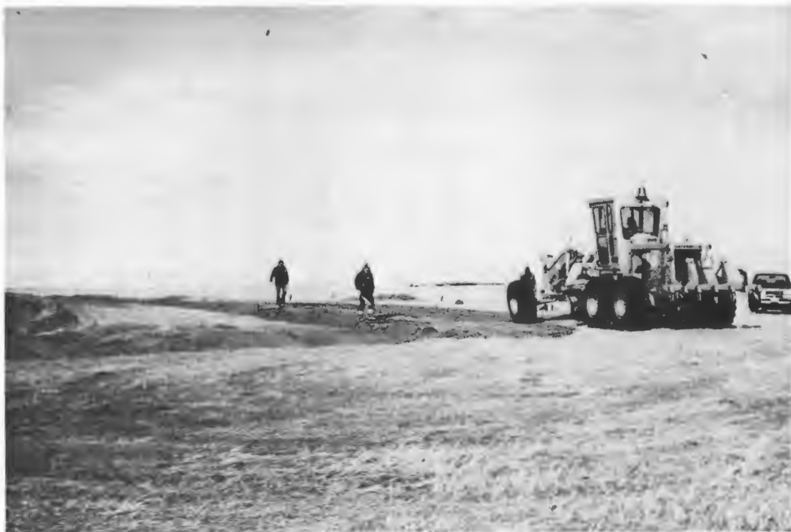
Figure 19: Controlled Surface Stripping in Progress on the Edge of Forty Mile Coulee.
