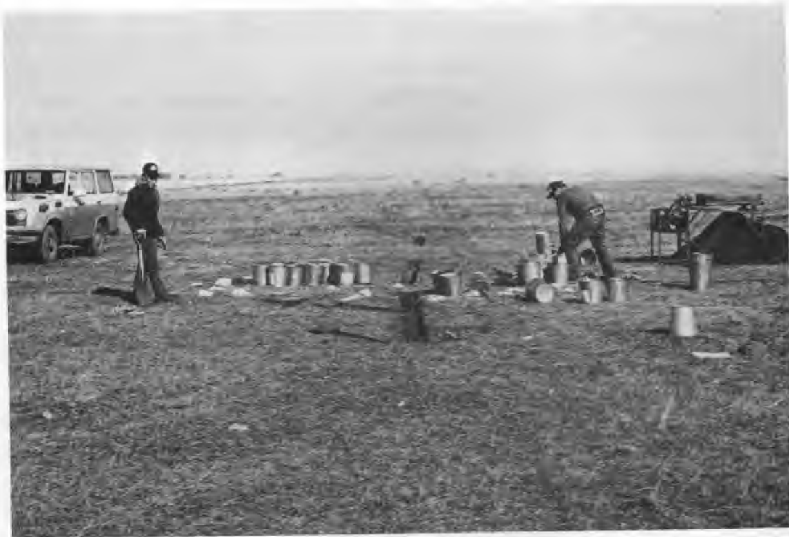
Figure 15: Test Trench Excavation in Progress.
