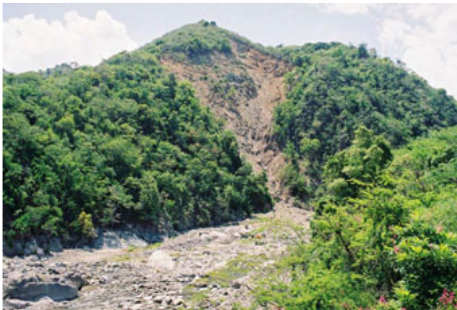
Figure G.15 – Shallow landslide induced by rainfall between Ramble and Somerset on the Yallahs River in St Thomas Parish, eastern Jamaica. The road followed the shoulder of the hill to either side of the landslide.
