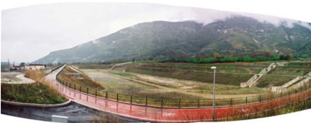
Figure 8.22 – Debris basin with a peripheral cycle track at Sarno in Italy.
