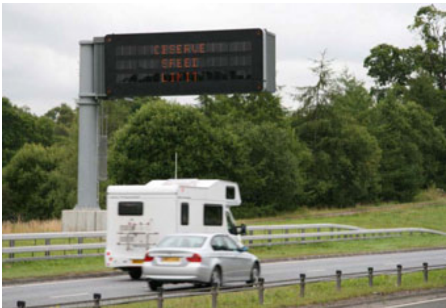
Figure 8.3 – A variable message sign located on the A9. The network of such signs in Scotland is being significantly increased and will form a crucial part of the strategy for warning road users of hazards including landslides.
