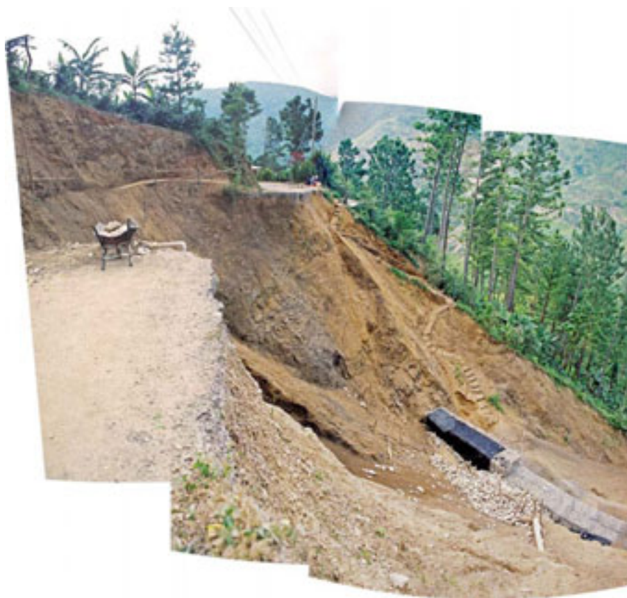
Figure G.17 – Deep rainfall-induced landslide on the B1 road at Section in Portland Parish, eastern Jamaica.
