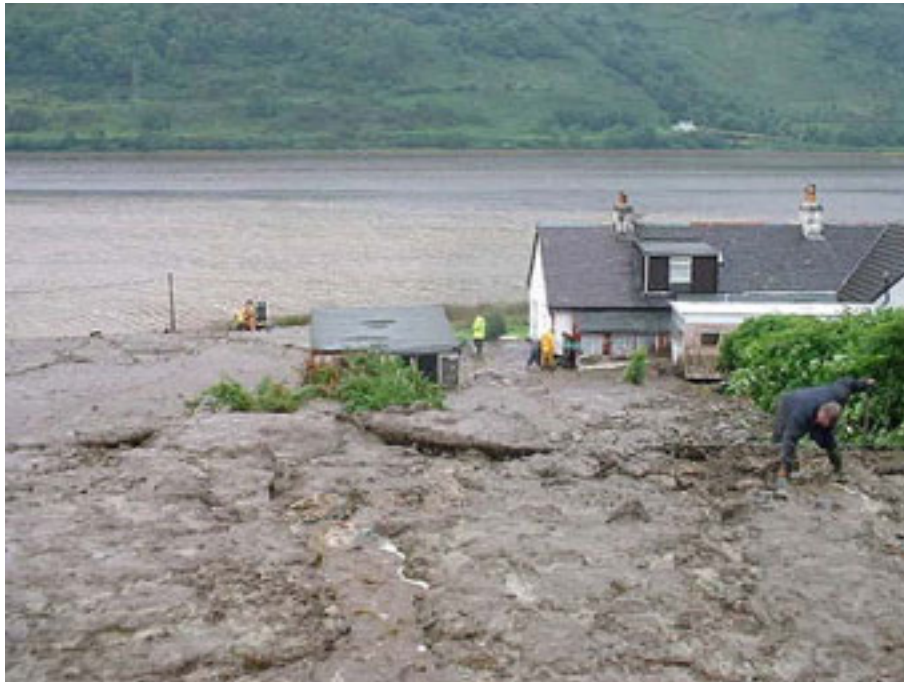
Figure 2.4 – Debris flow above the A83 to the west of Cairndow showing the effects on a roadside cottage and the trunk road immediately downslope from the cottage.
