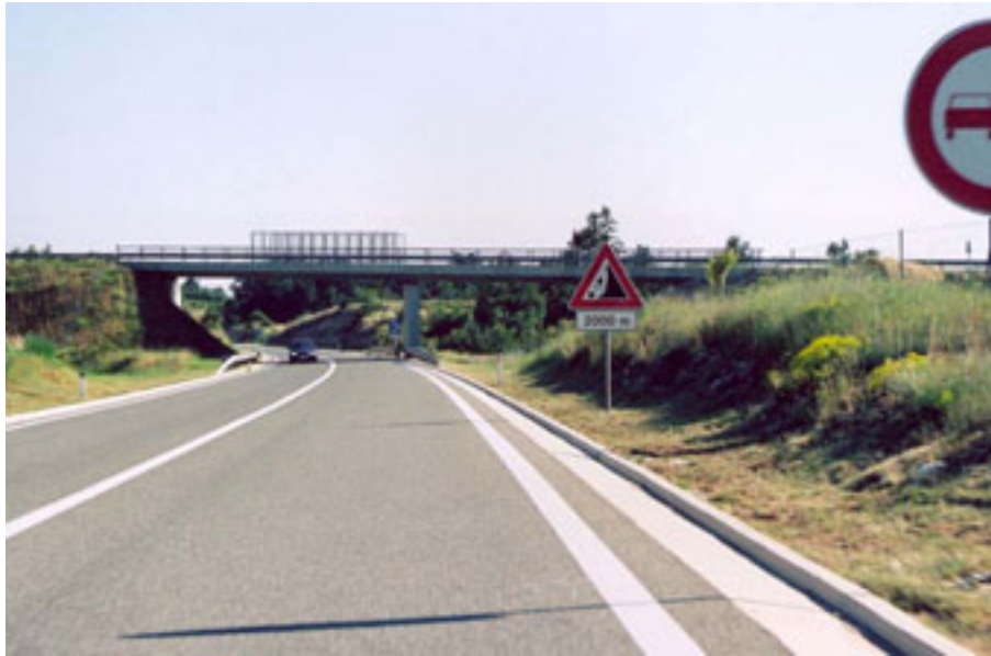
Figure E.12 – Rockfall sign in Croatia.
