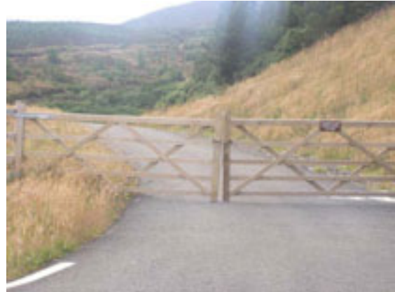
Figure C.35 – New road next to stream facing North NGR location ND040170.
