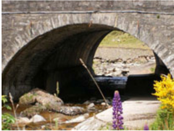
Figure C.43 – Old Masonry Bridge extended to form large culvert NGR location NN640730
