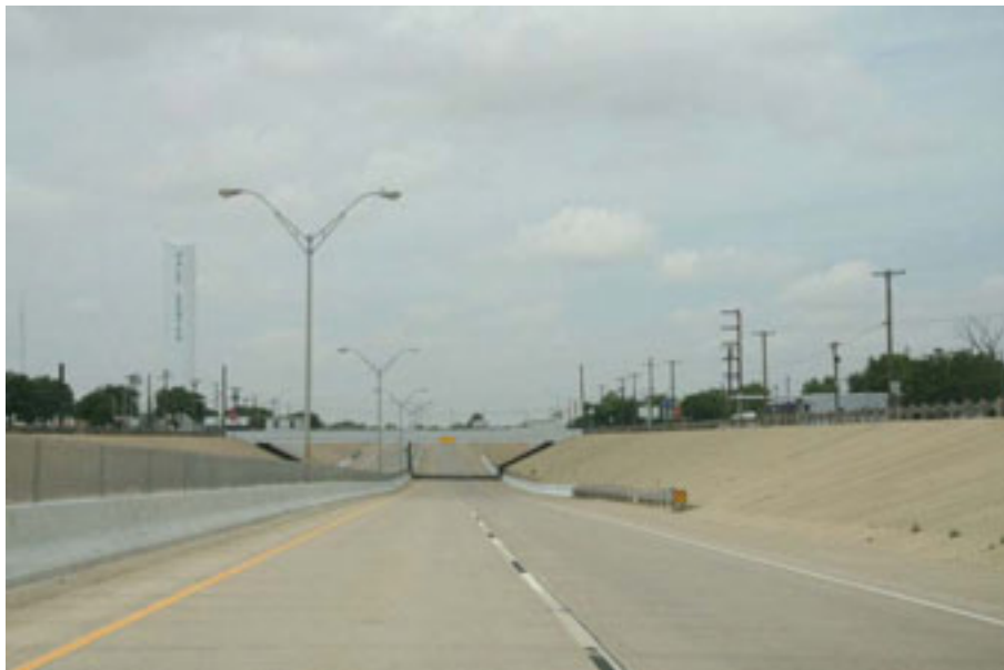
Figure E.20 – Water hazard associated with the signs illustrated in Figures E.18 and E.19, Interstate 28, Hale County, Texas.
