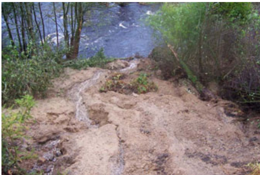
Figure 2.27 – Erosion and deposition below road, Struie.
