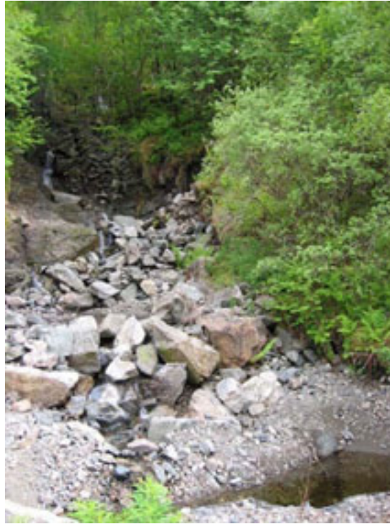
Figure 8.14 – Debris stilling basins at Frenchman’s Burn, A890 Stromeferry, Highland. (Courtesy of Ian Nettleton, Coffey Geotechnics.)
