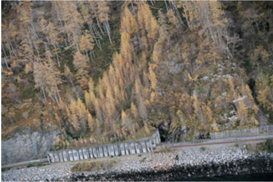
Figure 8.18 – Stone shelter on A890 north-east of Stromeferry.
