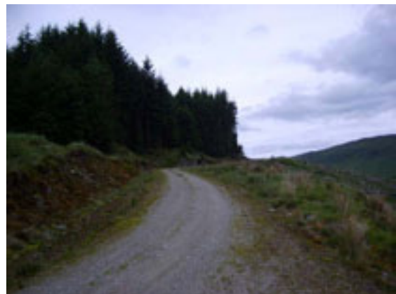
Figure C.16 – NGR location NN440270 (forest road).
