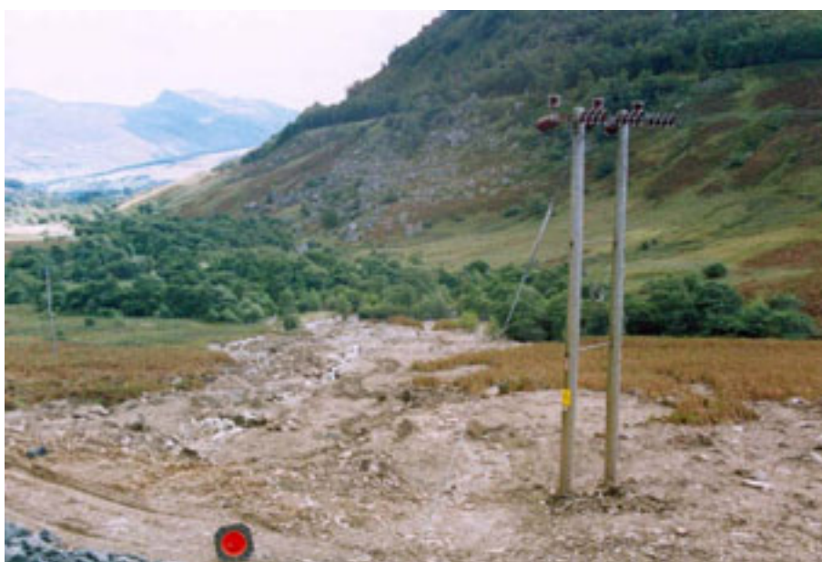
Figure 2.13 – The debris fan formed by the northern debris flow in Glen Ogle viewed from the A85 trunk road, looking towards Glen Ogle Burn and down the valley towards Lochearnhead.
