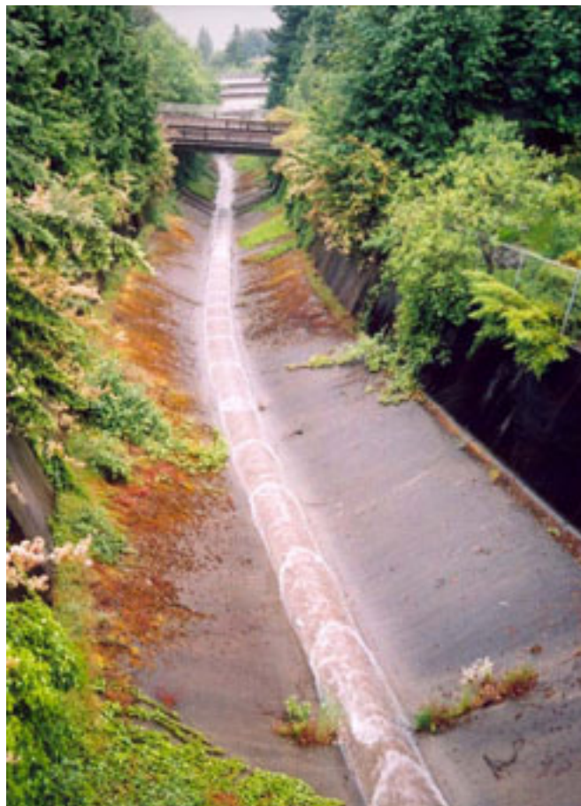
Figure 8.15 – Stream/debris channel, Alberta Creek, Sea-to-Sky Highway, British Columbia, Canada.
