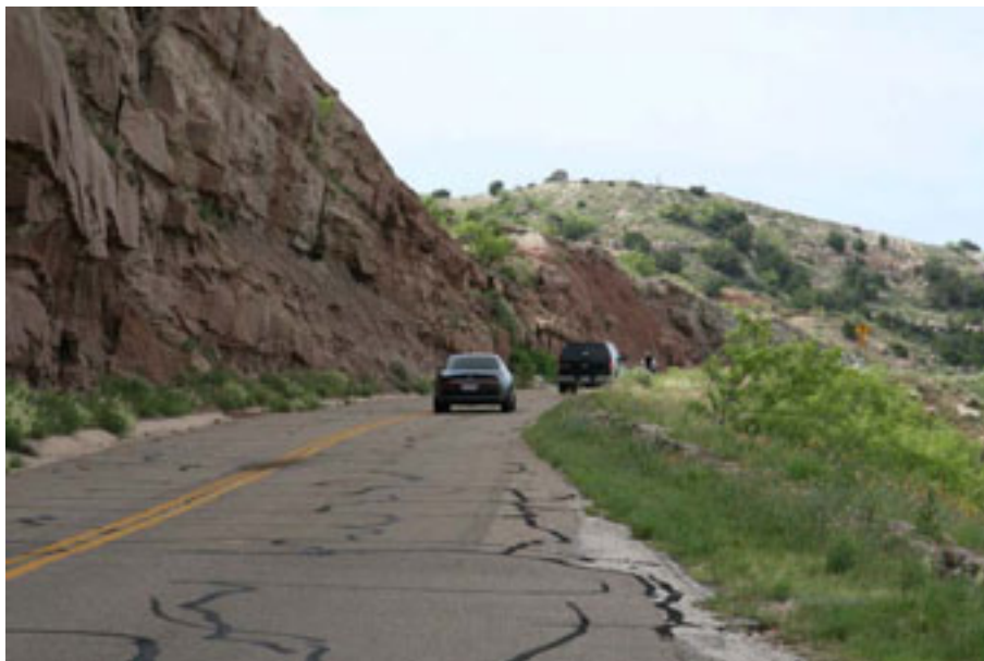
Figure E.15 – Rockfall hazards associated with the sign illustrated in Figure E.14, Palo Duro Canyon State Park, Texas.
