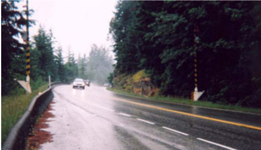
Figure 8.2 – Gates used to effect road closure following landslide events on the Vancouver to Whistler, Sea-to-Sky Highway, British Columbia, Canada.
