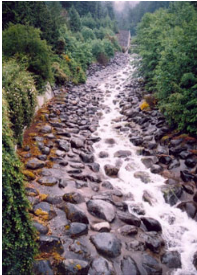
Figure 8.16 – Stream/debris channel, Harvey Creek, Sea-to-Sky Highway, British Columbia, Canada.
