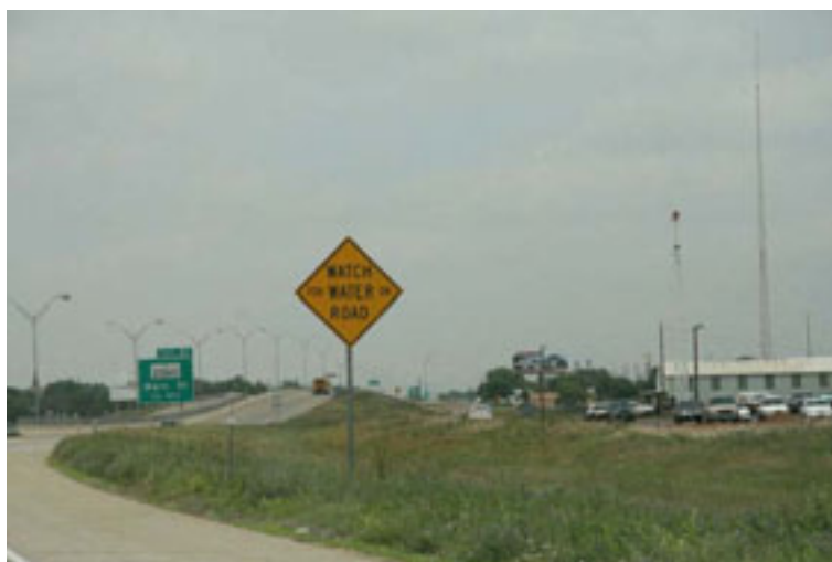
Figure E.18 – Water hazard sign Interstate 28, Hale County, Texas.
