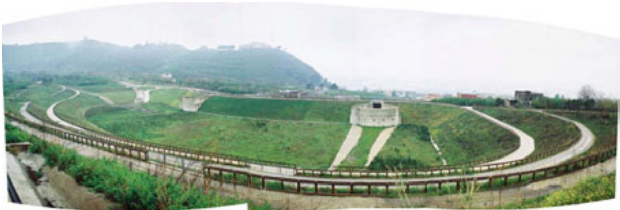
Figure 8.21 – Debris basin with a capacity of approximately 176,000m 3 at Sarno in Italy.
