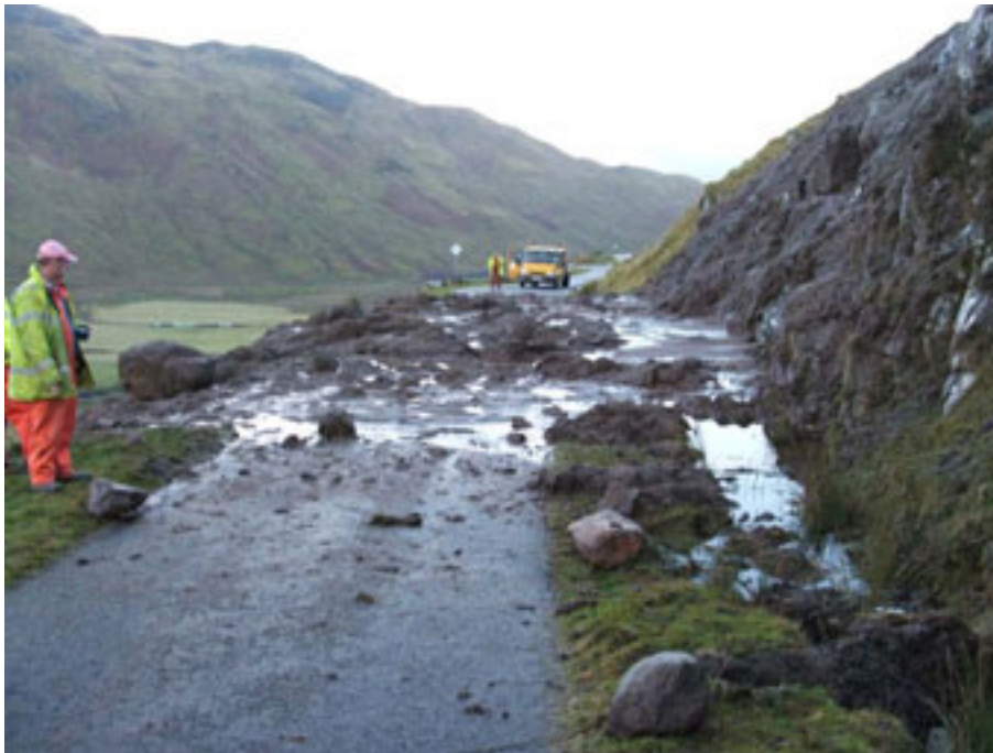
Figure 2.20 – Debris causing road closure at Glenelg.
