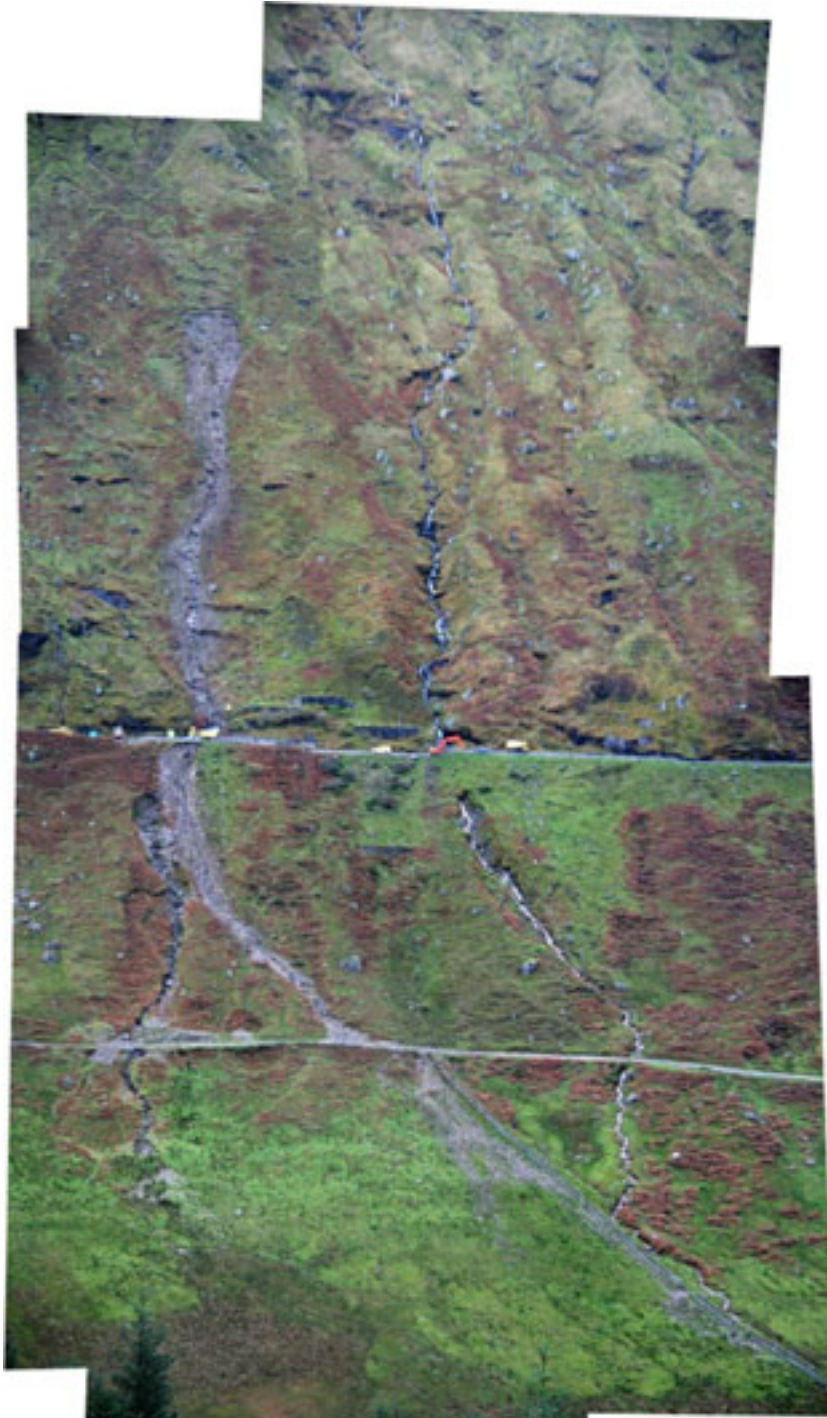
Figure 2.15 – View of the debris flows above and below the A83 on the approach to the Rest and be Thankful (from NGR NN 23160 06559 on the opposite side of Glen Croe). The head scar is at approximately 370m AOD, the A83 at 240m AOD and the old road at 180m AOD.
