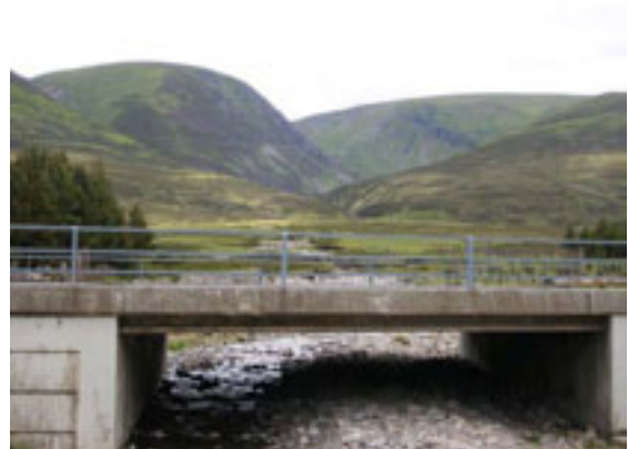
Figure C.42 – Bridge NGR location NN630800.
