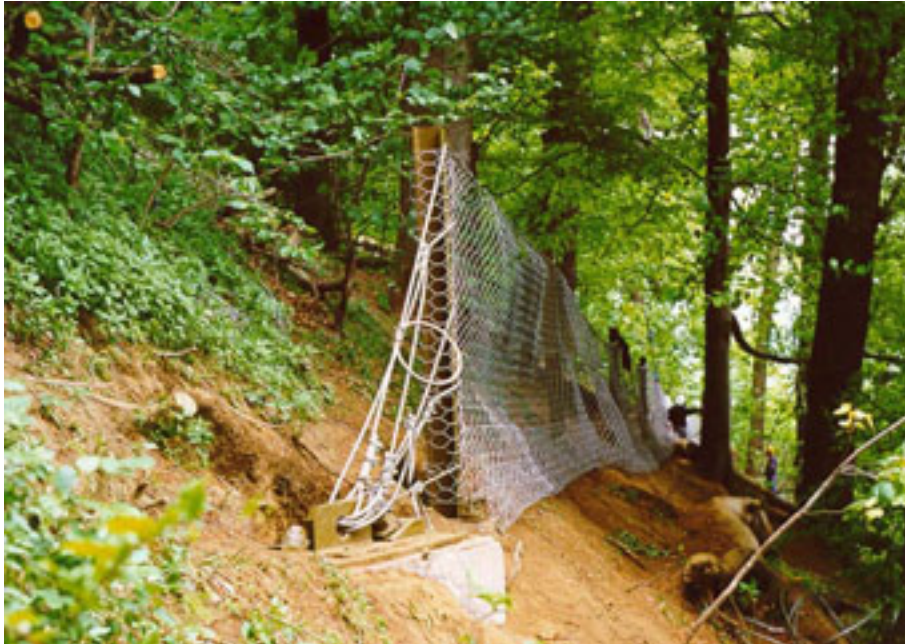
Figure 8.19 – Flexible rockfall catch fence, Abbey Craig, Stirling.
