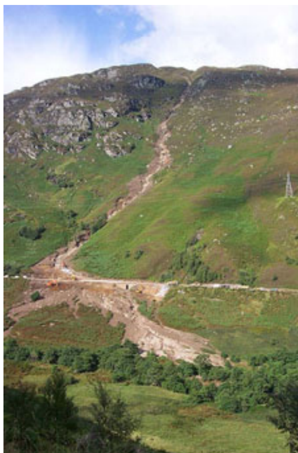
Figure 2.11 – View of the northern A85 Glen Ogle debris flow two days after the event, showing the sharp bend in the channel just above road level.
