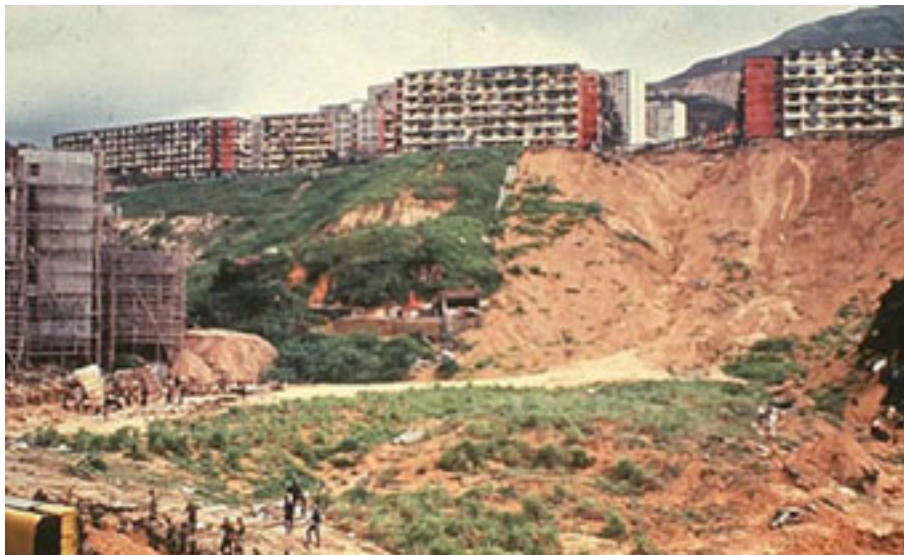
Figure G.3 – Sua Ma Ping Estate landslide, 18 June 1972. A 40m high road embankment collapsed after 232mm of rain.
