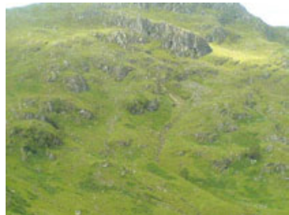
Figure C.21 – Recent instability (below lower outcrop in centre of picture), taken from NGR location NG962 149 looking west.
