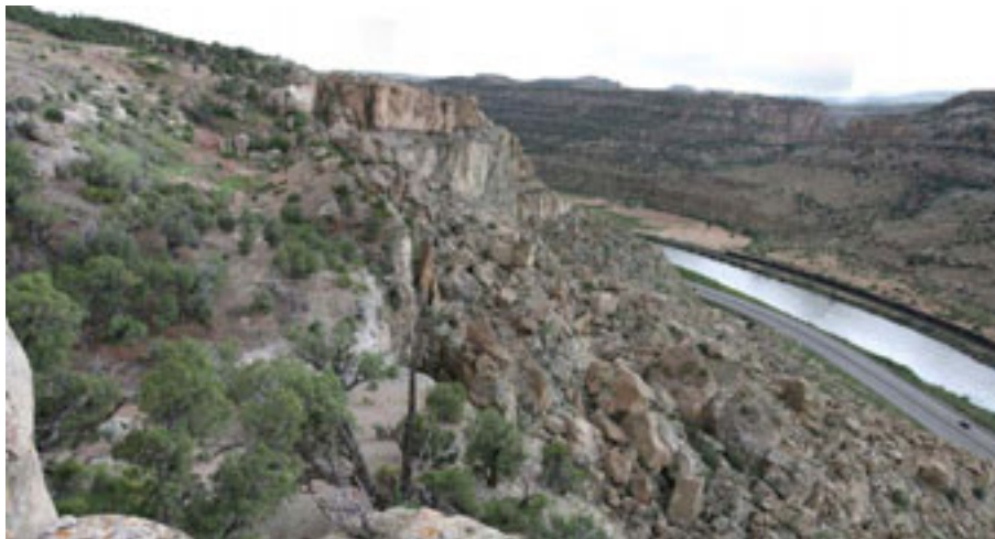
Figure 3.2 – DeBeque Canyon landslide showing Interstate 70 passing over the toe.
