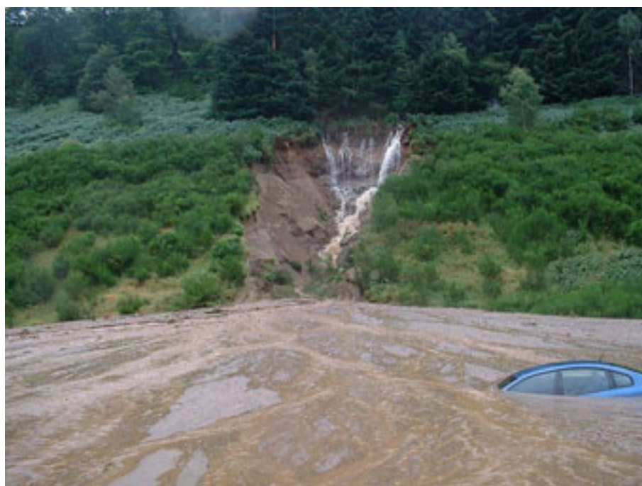
Figure 2.9 – The southerly debris flow at the A9 north of Dunkeld. The flow has formed its own channel by erosion. Photograph dated 12 August 2004. (Courtesy of Alan Mackenzie, BEAR.)
