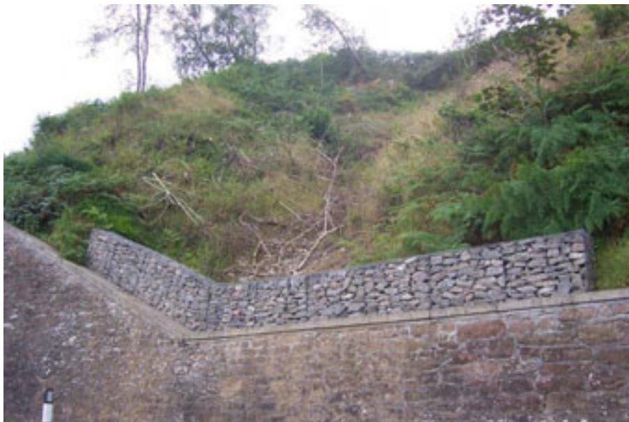
Figure 2.28 – Gabion debris trap, Struie.
