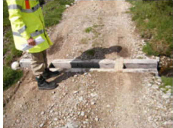
Figure C.40 – Drainage installed on tracks present behind Drumochter lodge NGR location NN630790.
