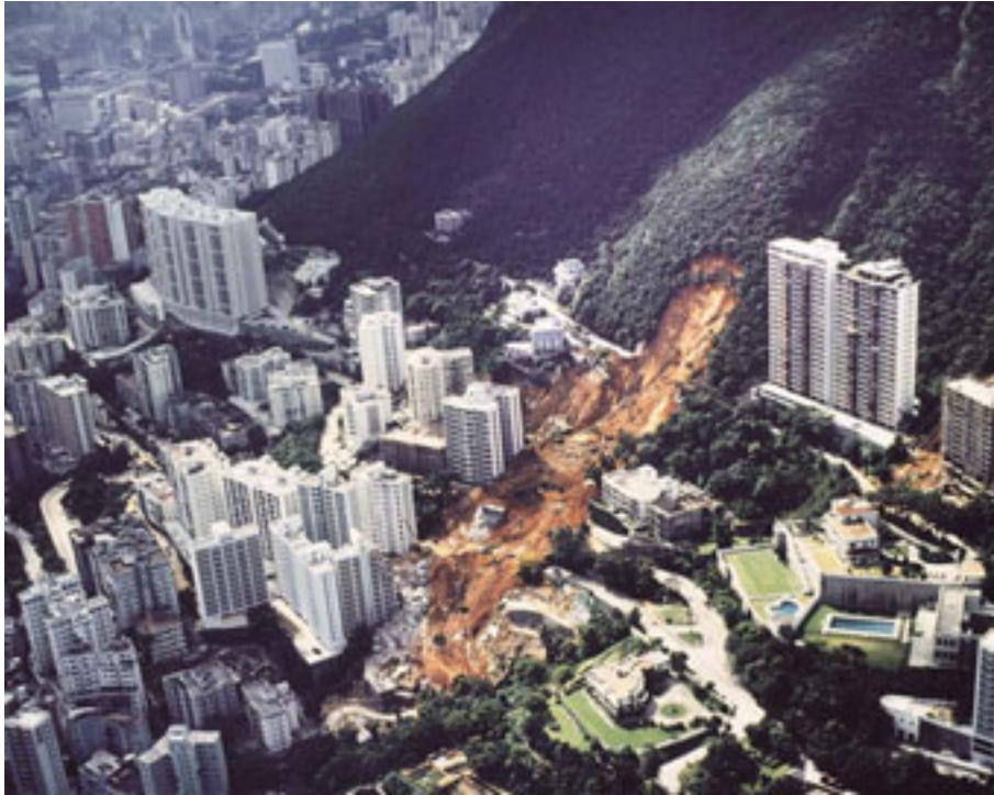
Figure G.4 – Po Shan Road Landslide, Mid-Levels, Hong Kong Island 18 June 1972. The landslide occurred on a steep hillside above a temporary excavation and demolished a 12-storey building.
