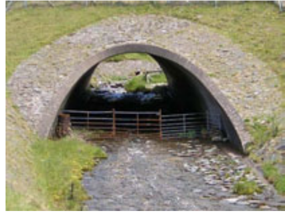
Figure C.44 – Large Culvert NGR location NN630750.
