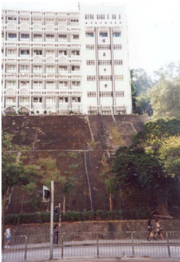
Figure 3.4 – A shotcrete slope in Kowloon, Hong Kong SAR.
