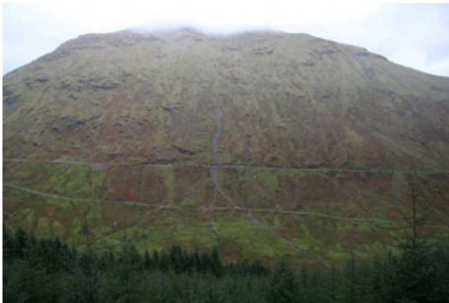
Figure 2.14 – View of the hillside above and below the approach from the east to the Rest and be Thankful (from NGR NN 23160 06559 on the opposite side of Glen Croe). Not only can the event dated 28 October 2007 be clearly seen but evidence of numerous past events can be seen on the surrounding hillside.
