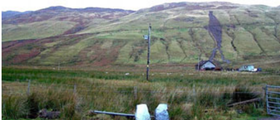
Figure 2.22 – Slips on hillside above and below road at Glenelg.
