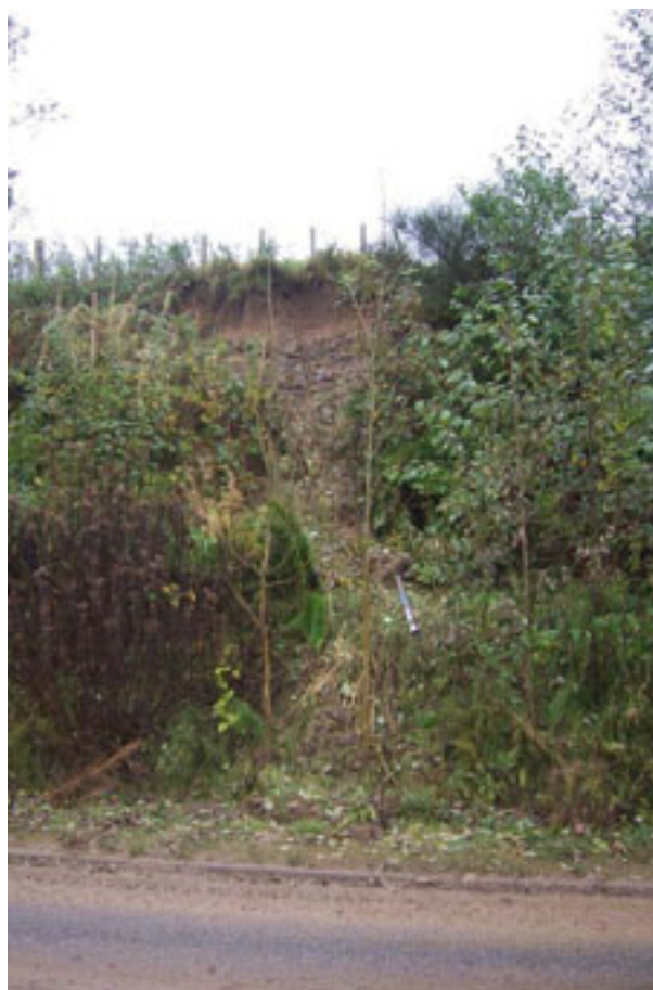
Figure 2.29 – Ardullie slip above road.
