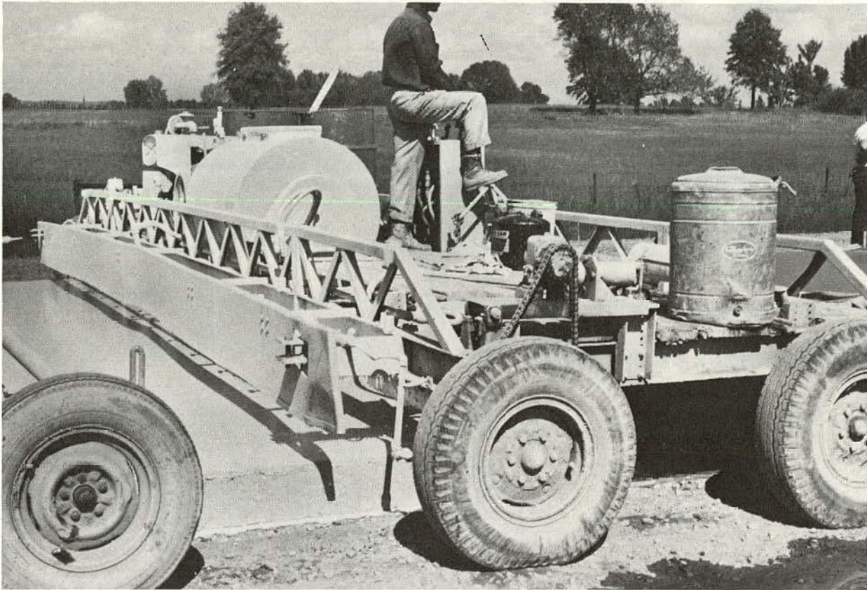
Figure 19. Machine-placed white-pigmented curing compound.
