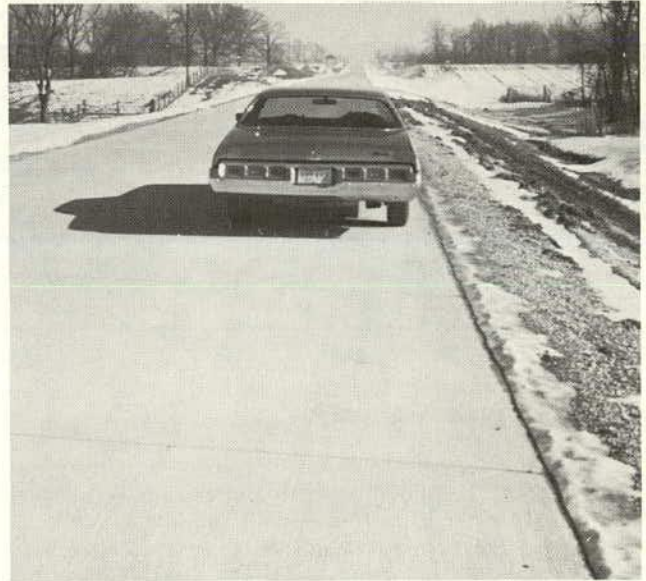
Figure 3. Example of an Illinois low-volume county road built using 6- and 7-in. plain concrete with no base.
