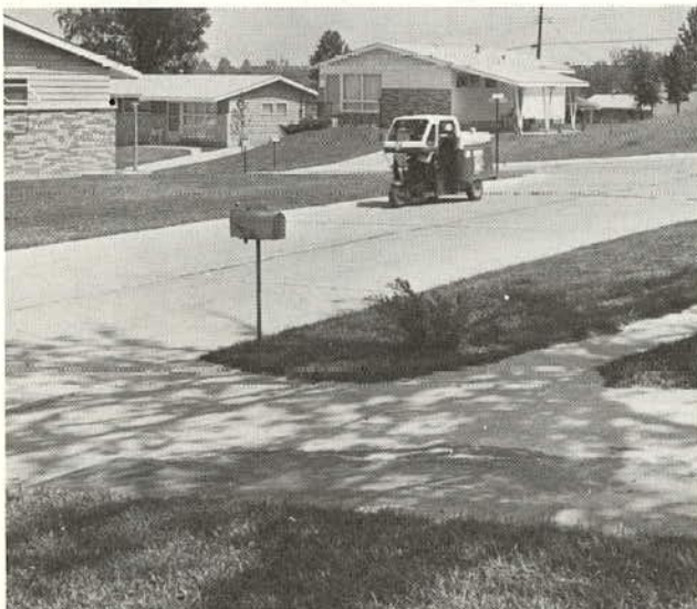
Figure 4. Example of low-volume residential street paved with concrete having integral curb and gutter.
