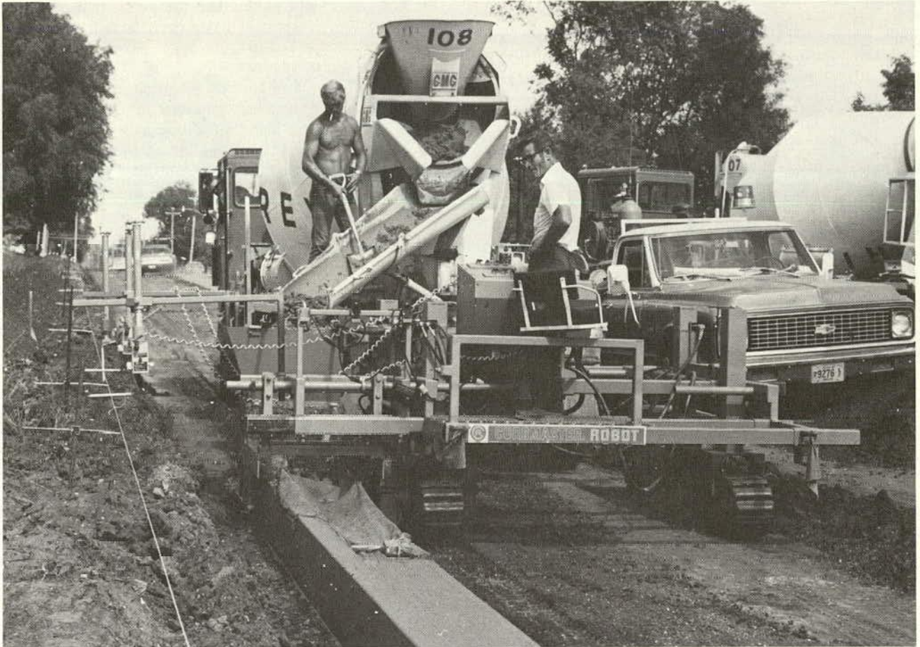
Figure 14. Slip-forming curb and gutter.
