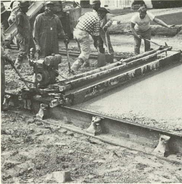
Figure 16. Vibrating hand screed used on a city street project.
