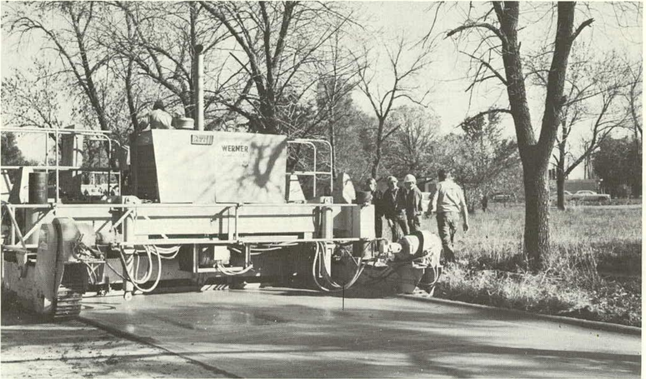
Figure 7. Slip-form paving a city street with integral curb.
