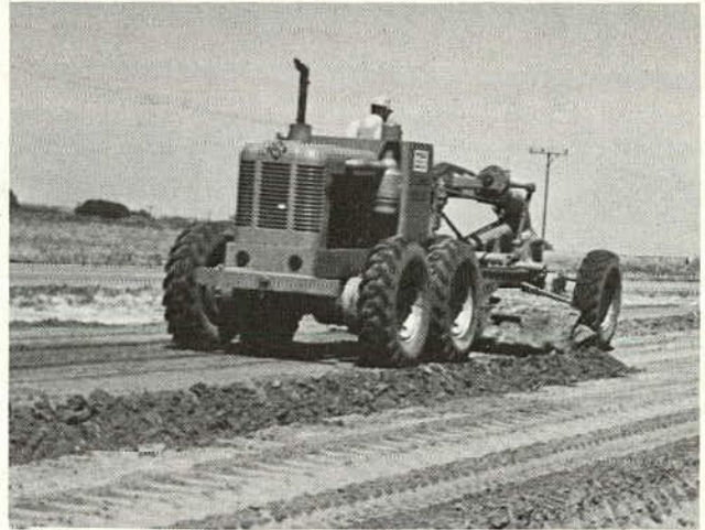
Figure 11. Subgrade shaping.
