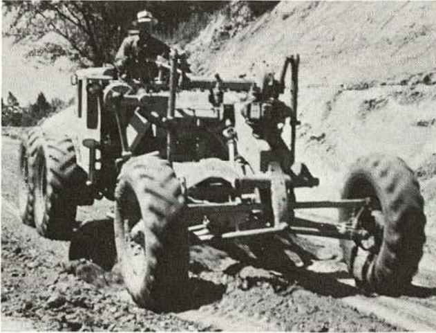
Figure 10. Scarifying and blending varied subgrade soils.
