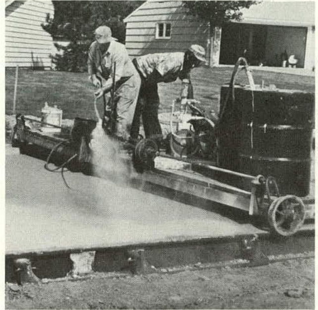
Figure 20. Hand-sprayed white-pigmented curing compound on city street.
