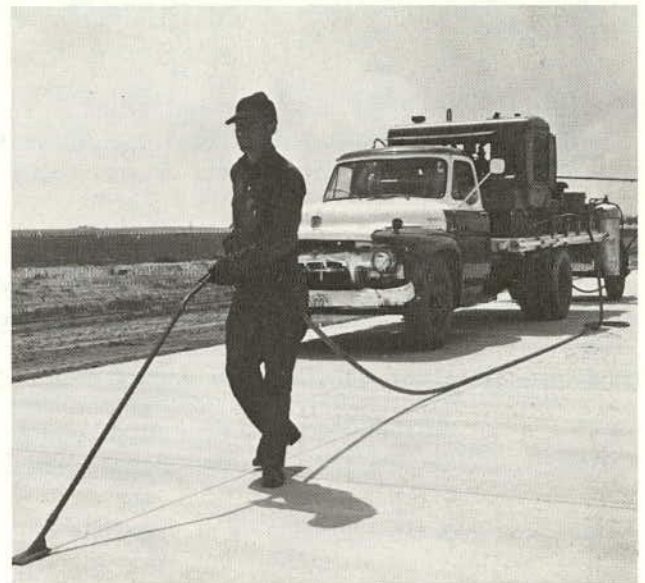
Figure 18. Sealing joints with pressure applicator.
