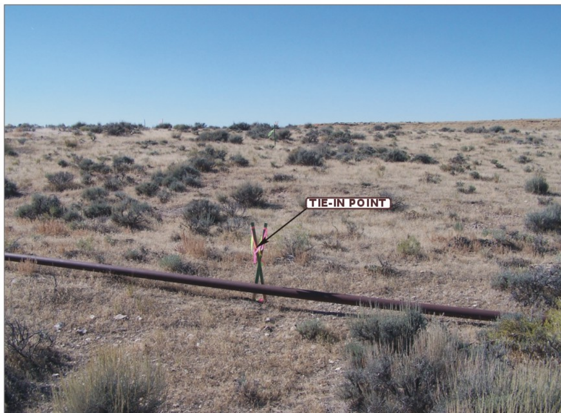
PHOTO: VIEW FROM TIE-IN POINT
