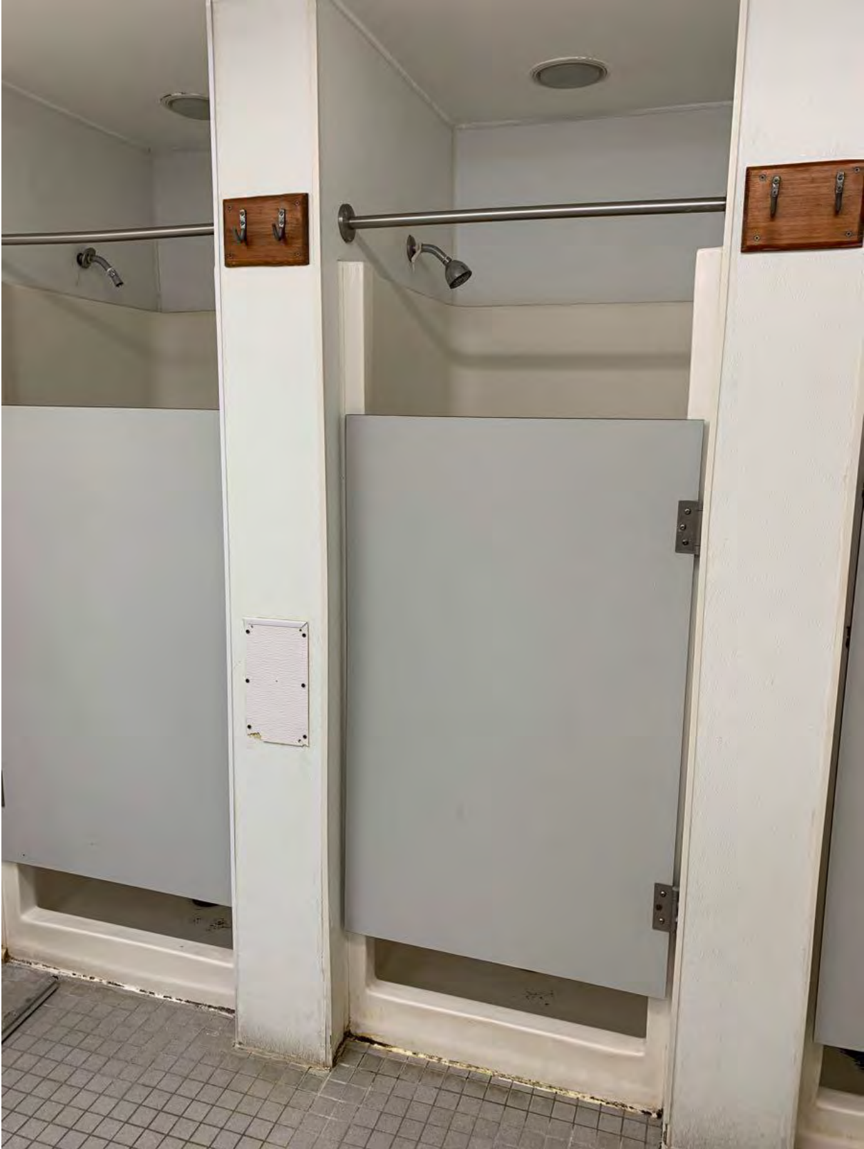
CCCC Olympic Bathroom and Shower
