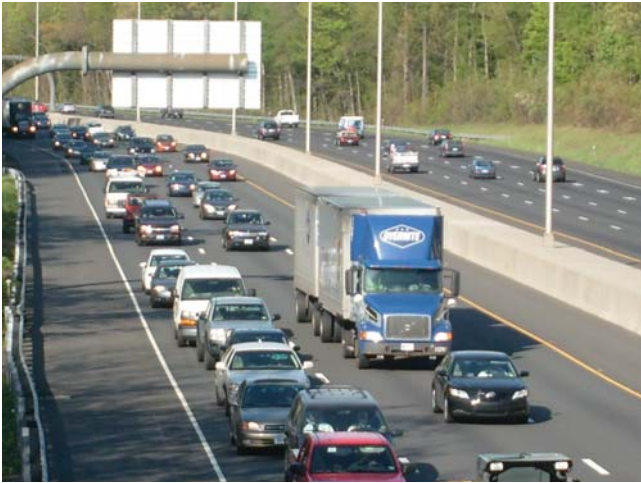
I-84 westbound, Waterbury
