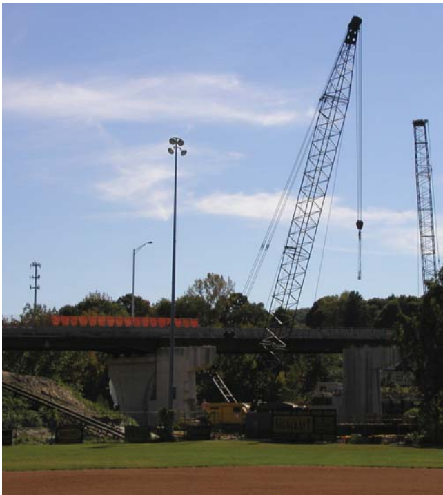
Bridge over Naugatuck River on Route 63, Naugatuck
