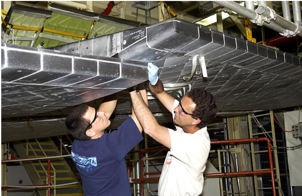
Figure 21. Thermal Protection Repair Activity Around Orbiter Elevon Aerosurfaces
