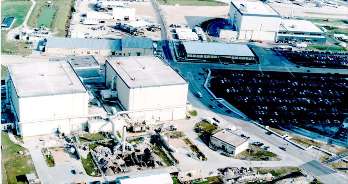
Figure 20. Orbiter Processing Facilities at Launch Complex 39
