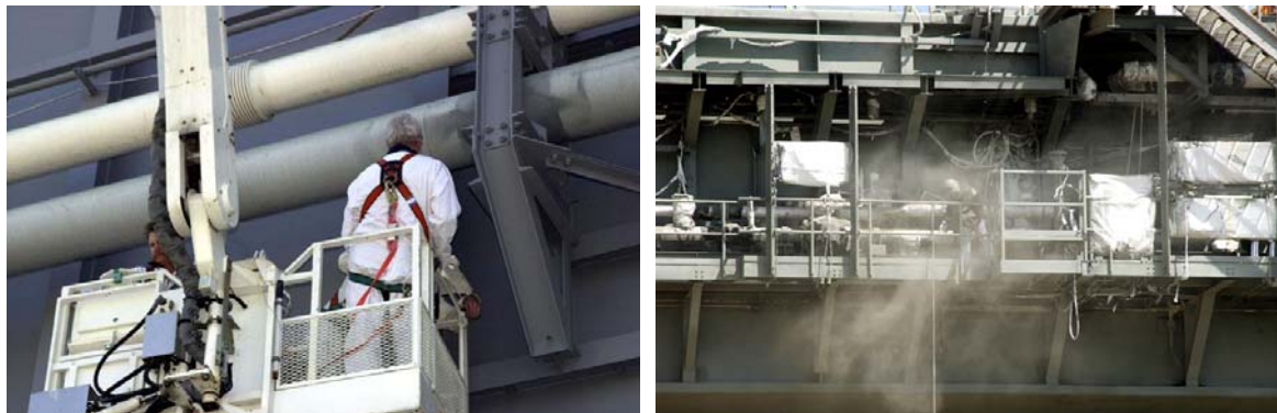
Figure 27. MLP Propellant Line Repair and Routine Sandblasting
