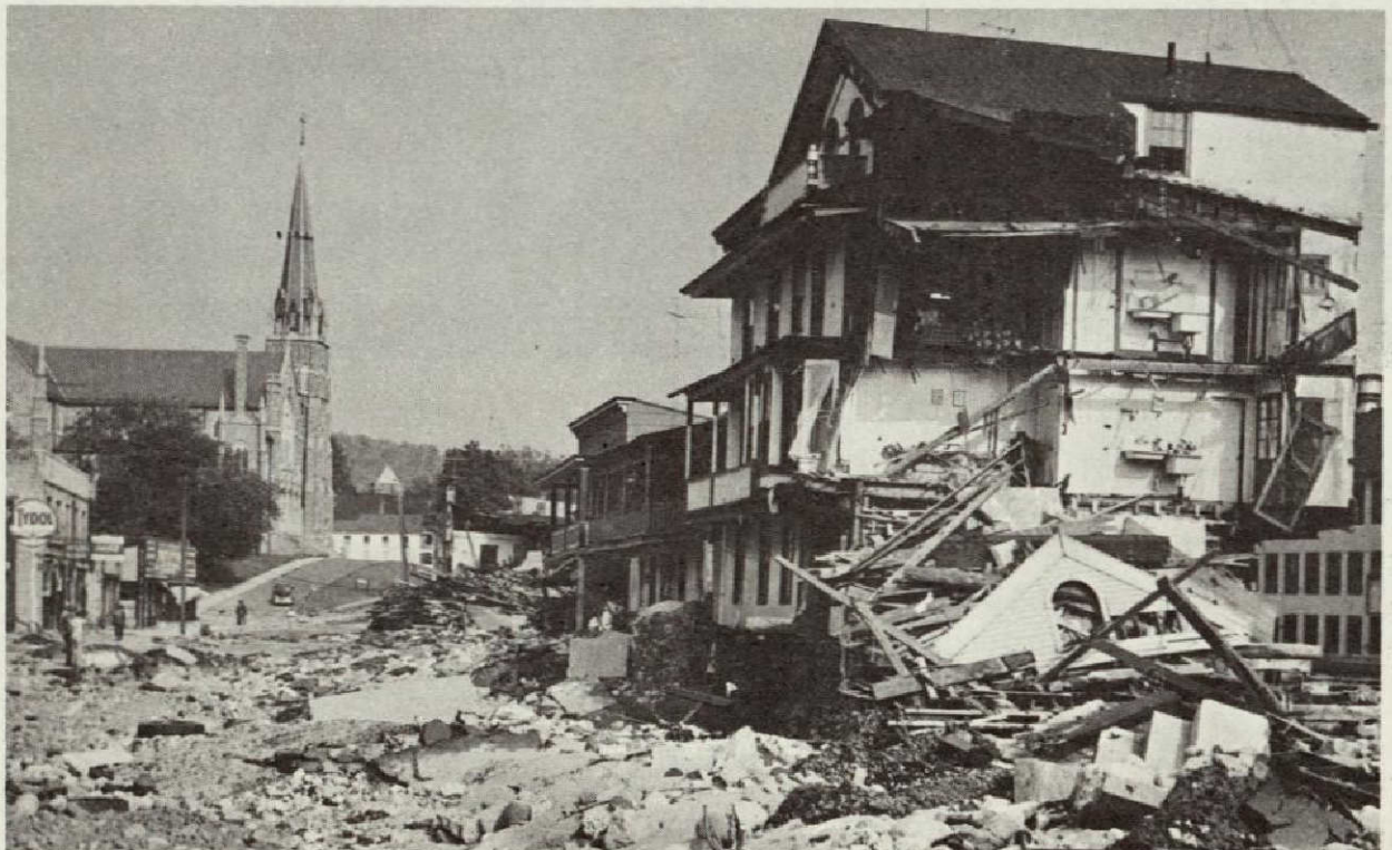
AUGUST 1955 FLOOD DAMAGE AT WINSTED, CONNECTICUT
