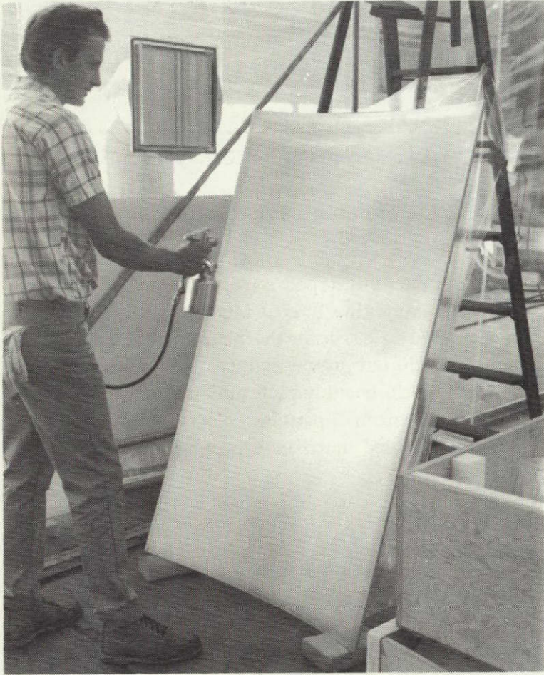
Figure 5-5. Priming An Insulation Panel
