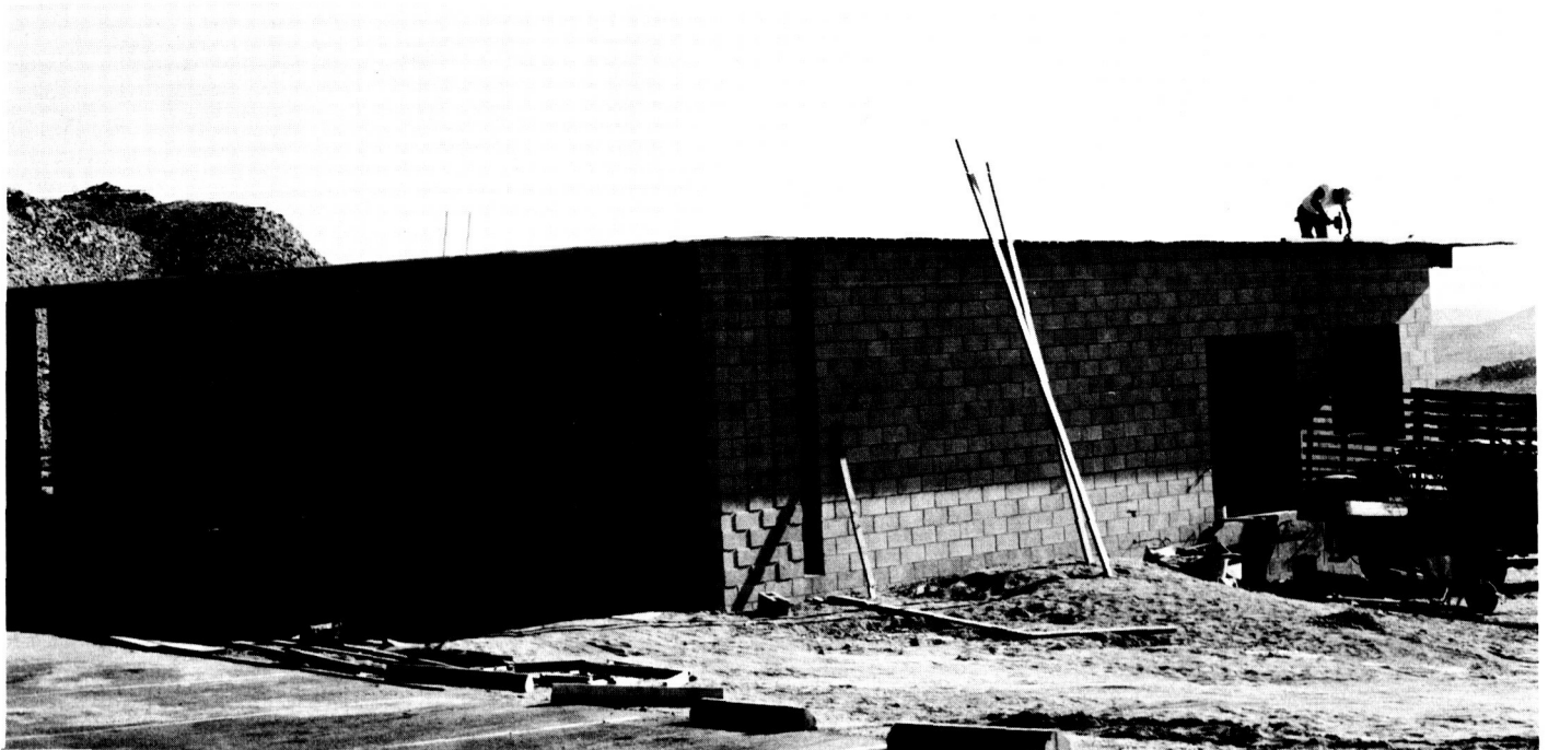
Fig. 7. Laboratory and office building, G-60, at Venus DSS
