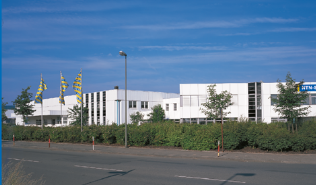
German production facility in Bielefeld
