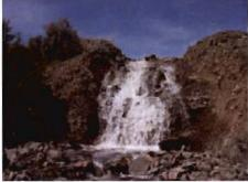
$\underline{\text{Modification 10}}$  – This is another earthen dam that is located upstream of modification 9. It is approximately ten to fifteen feet in height and has an outlet around the east side of the reservoir that is a fast water natural substrate chute.
