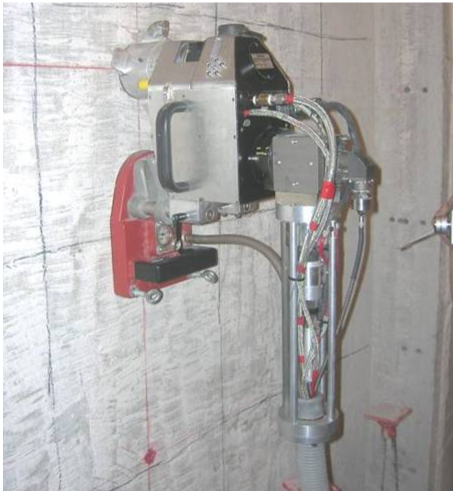
Figure 44. EWI Laser Cement Drilling Head on Cement Wall
