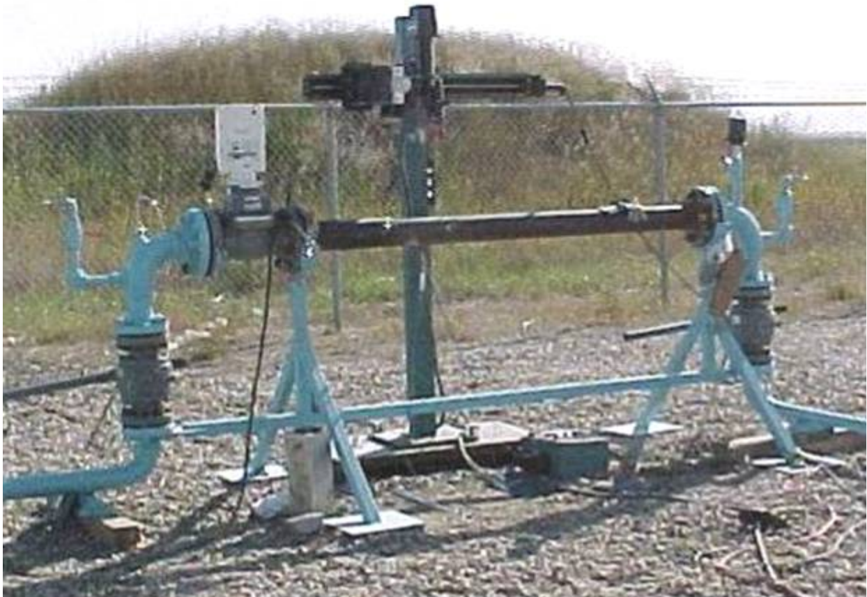
Figure 20. Set-Up for Welding Thin Wall Pipe with Pressurized Methane Gas
