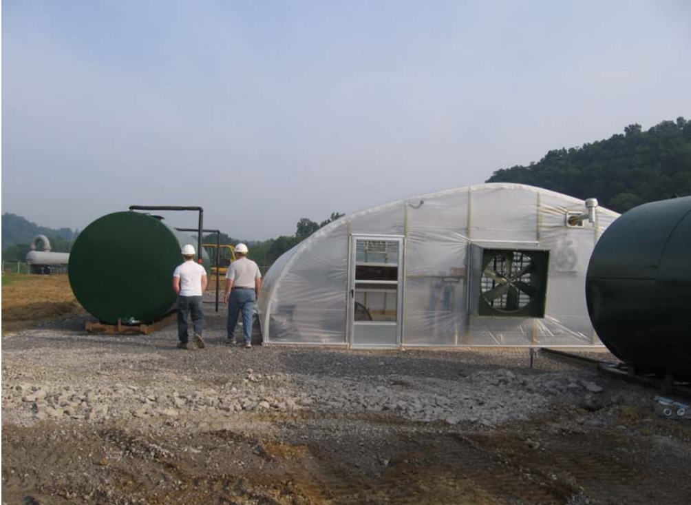
Figure 7. Exterior of greenhouse and tanks. Inflow tank is to the right, effluent tank is to the left.
