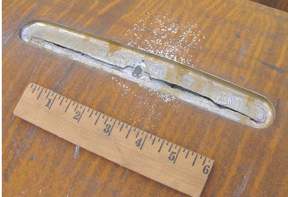
Figure 40. Simulated Corrosion Area after Burst Test
