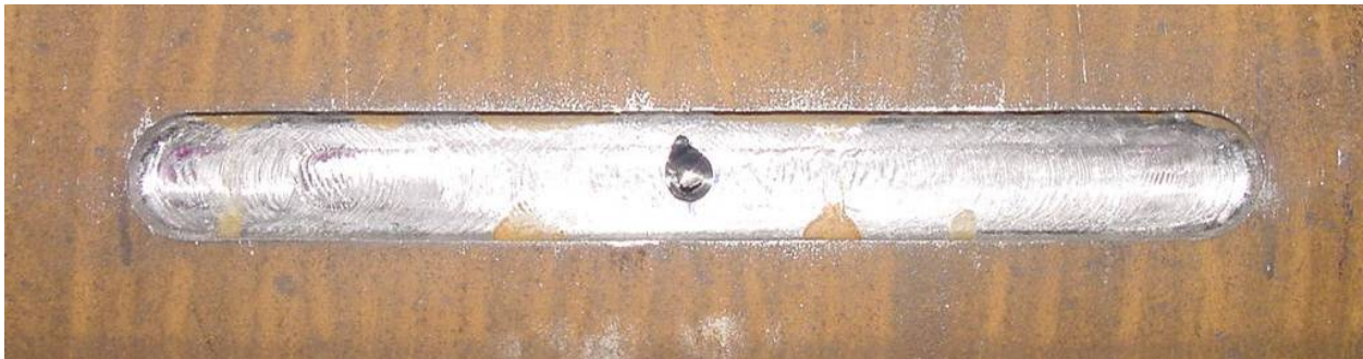
Figure 38. Short, Extra Deep Damage with Through Hole for 609.6 mm (24 in.) Pipe
