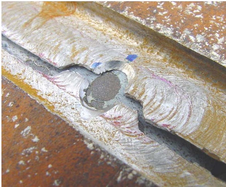
Figure 41. Close-Up of Simulated Corrosion Area after Burst Test
