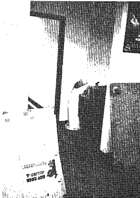
Figure 4-51: At a small electronics manufacturing facility, affected by the 1984 Morgan Hill Earthquake, a cantilevered, vertical section of HVAC duct broke from its horizontal header and fell.
