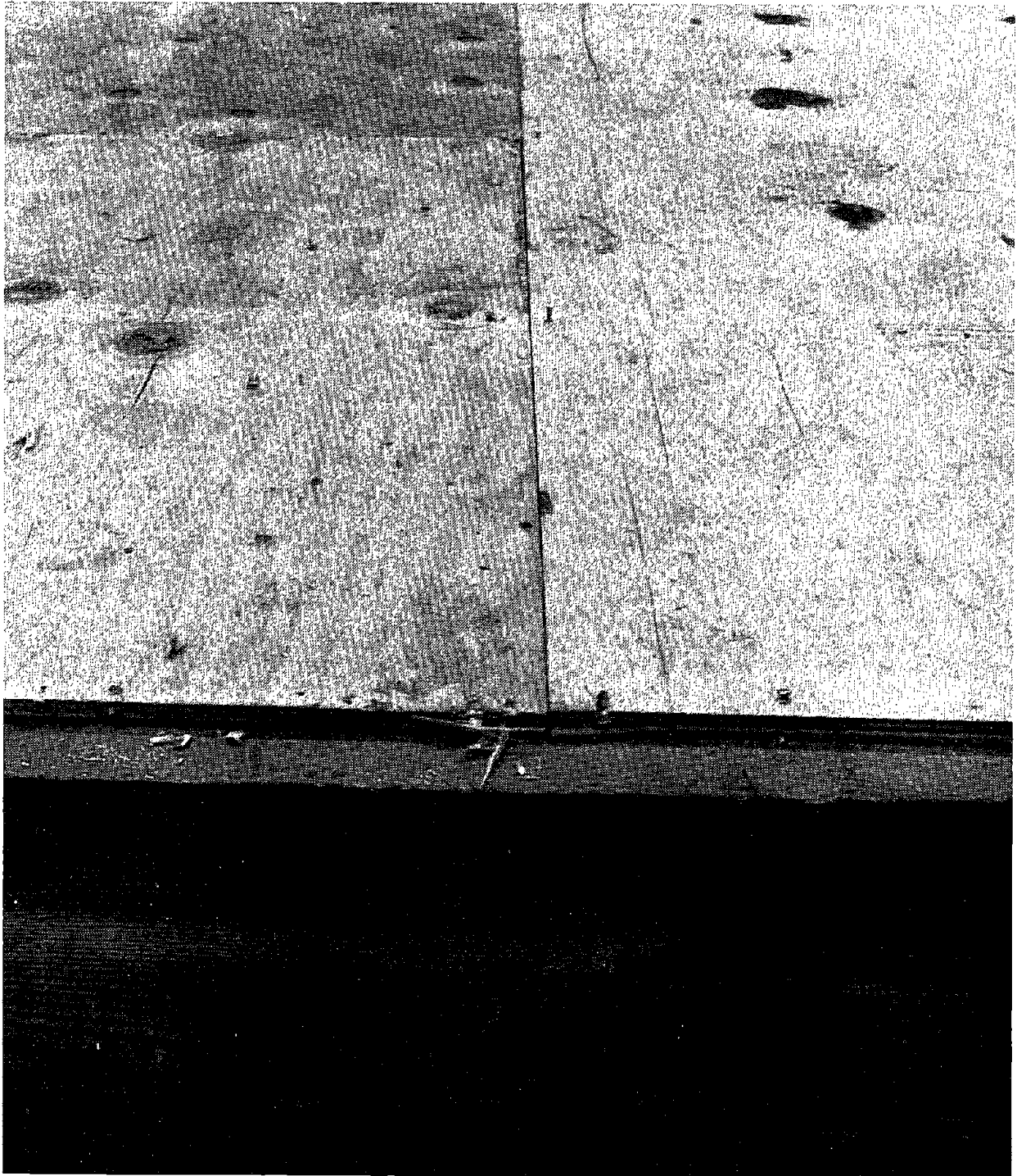
FIGURE 4-1. DIAPHRAGM B AFTER TESTING.
