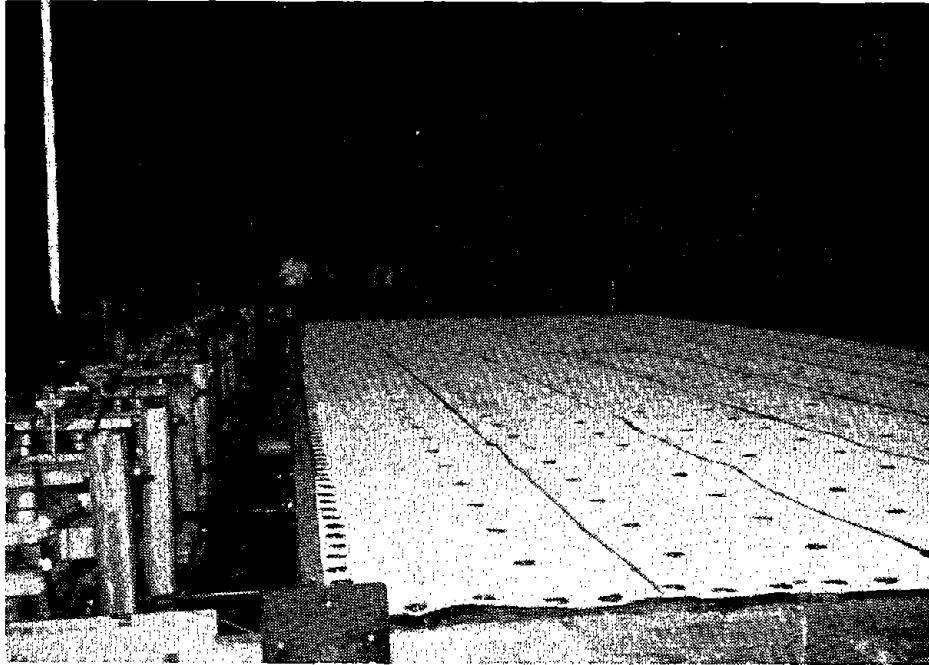
FIGURE 4-6. DIAPHRAGM I SHOWING SMALL BUCKLING WAVES IN ROOFING .
