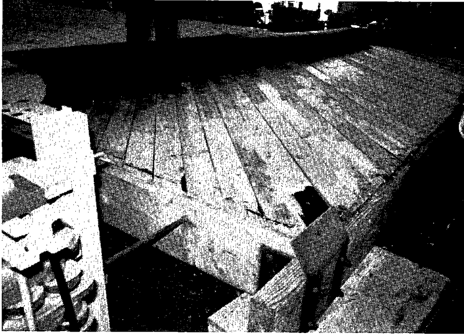
FIGURE 3-10. SOUTHEAST CORNER OF DIAPHRAGM I AFTER TEST.
