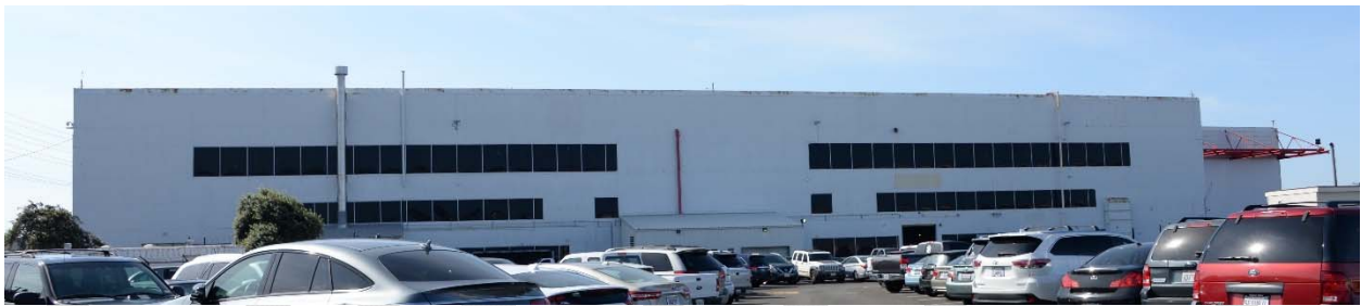
Photo: View of Facility 3 from the North side.
