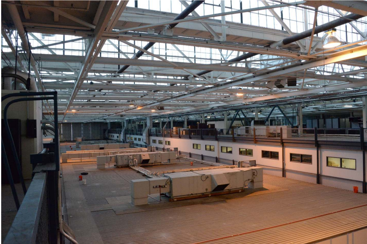
Photo: Interior view of Facility 2 showing roof trusses, machines and equipment.
