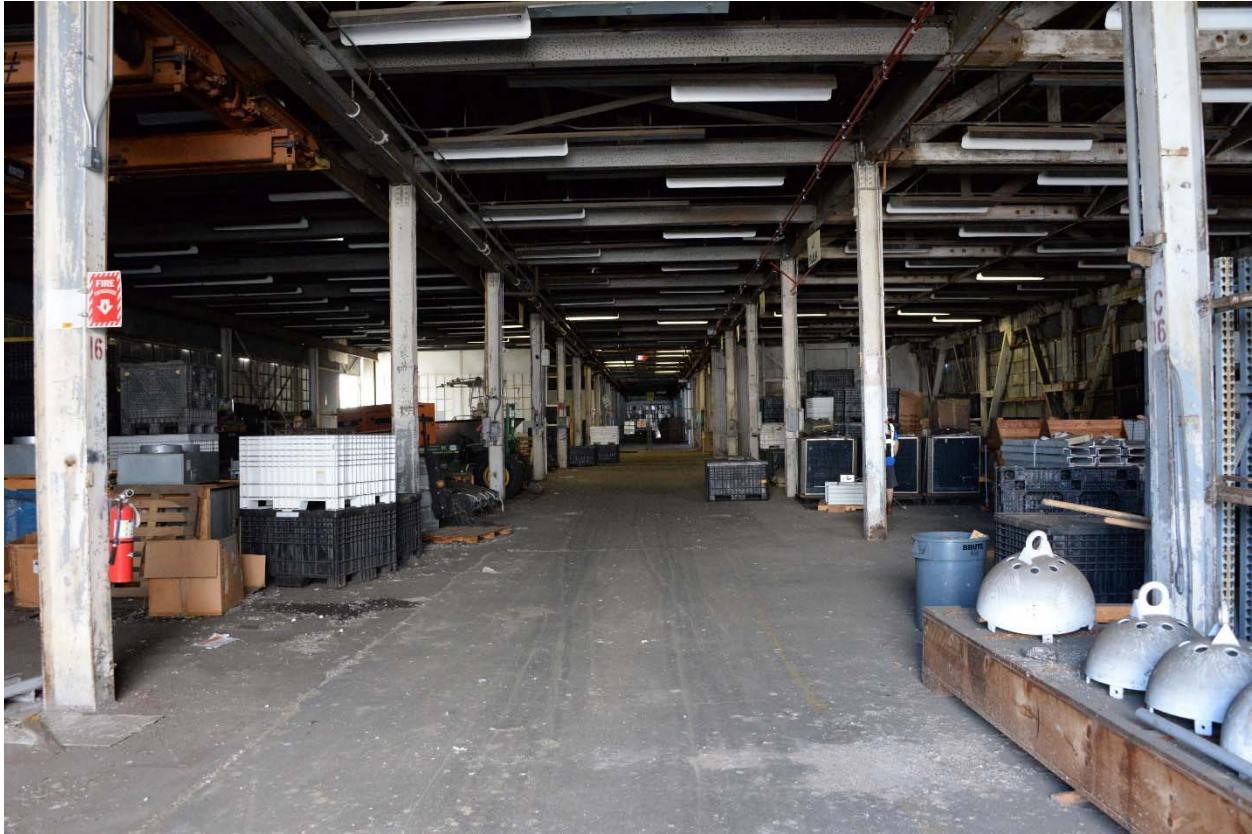
Photo: Interior view of Facility 8.
