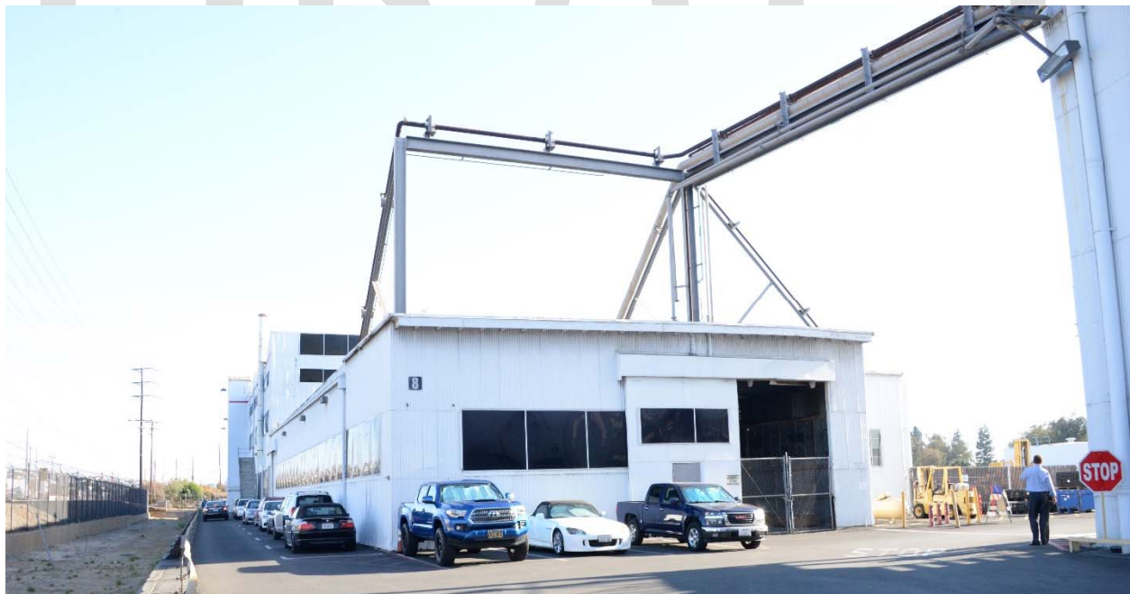
Photo: Northside view of Facility 8 with the railroad tracks to the east.
