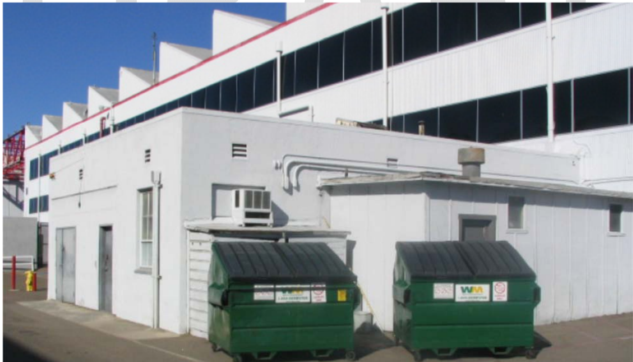
Photo: View of Facility 30 adjacent to Facility 2.
