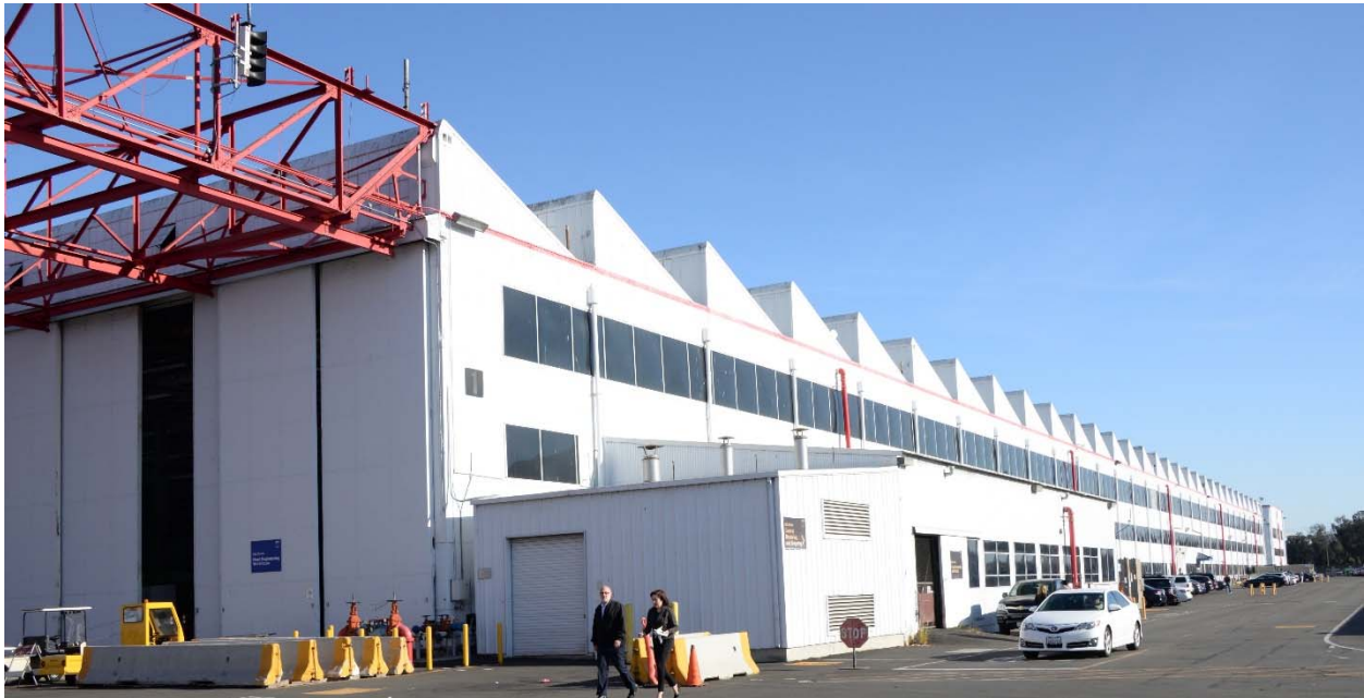
Photo: Northwest corner of Facility 1 looking south.
