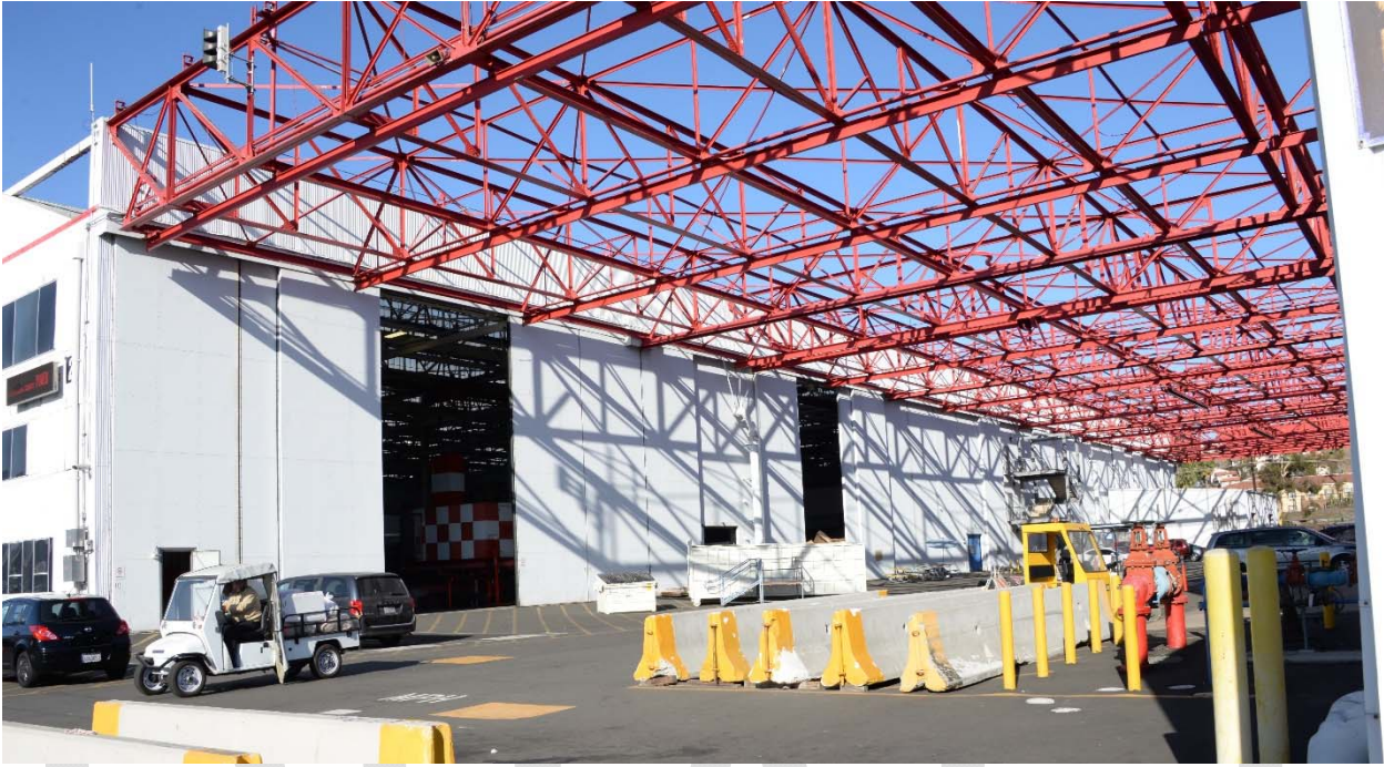
Photo: View of Facility 2 from the South.
