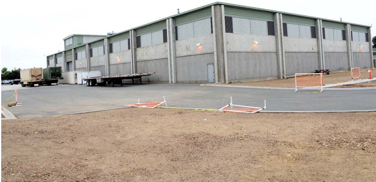
Photo: Southwest exterior view of Facility 2555.
