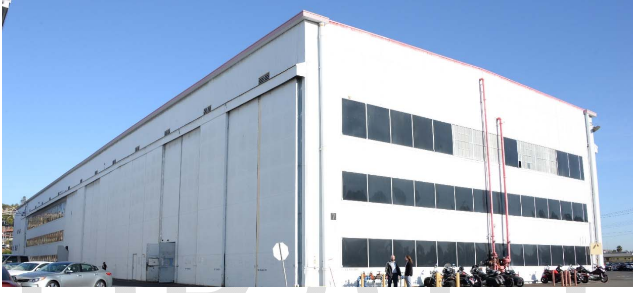
Photo: Northeast corner of Facility 7.
