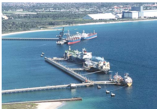
Fremantle Outer Harbor—Kwinana Oil Refinery Jetty
