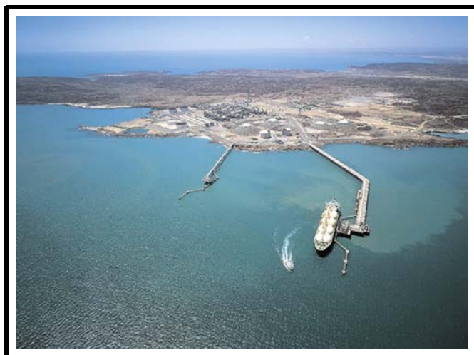
Copyright 2003 North West Shelf Australia LNG Pty Withnell Bay Loading Terminal
