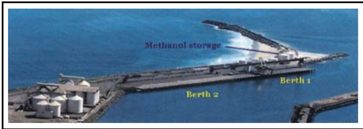
Bunbury—Berth No. 1 and Berth No. 2
