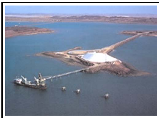
Courtesy of Dampier Port Authority Mistaken Island Salt Wharf
