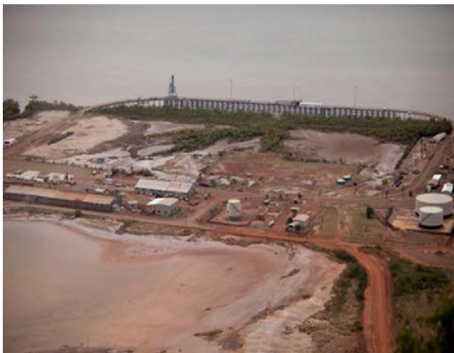
Wyndham Port Facility
