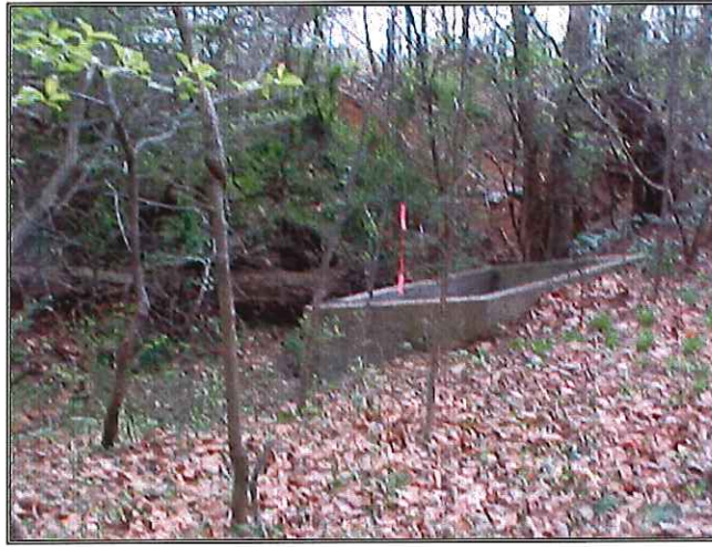
Photo #1 - Looking northeast – View of pump house foundation (A1).
