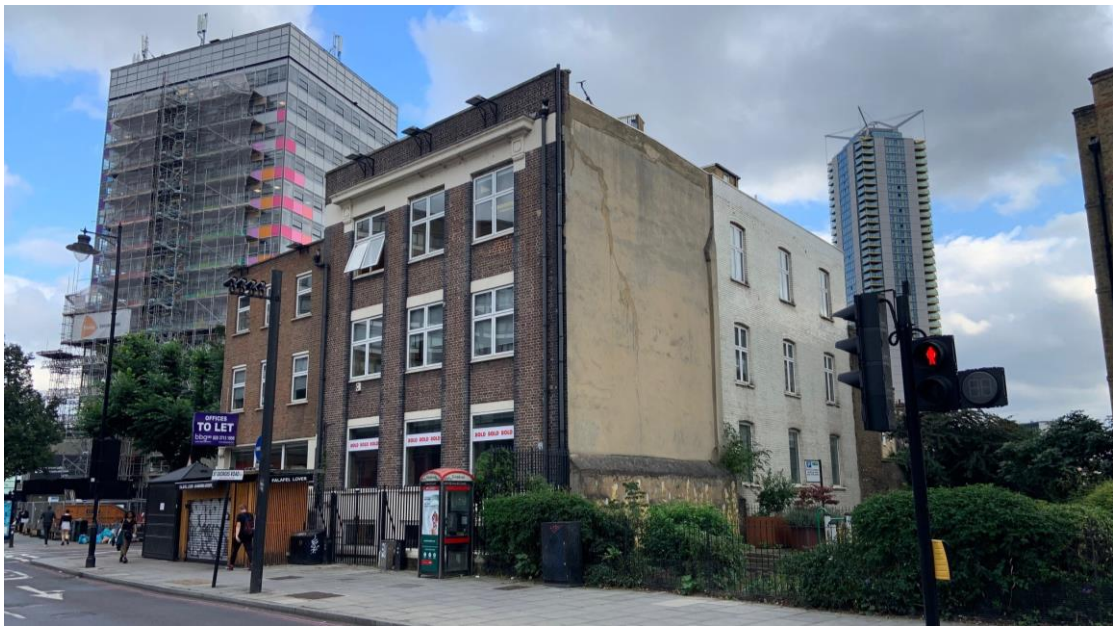
Image 02 (above): Photograph of the existing site, taken from St George's Road.
