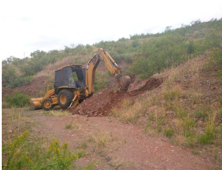
Photograph 9-2: Near continuous chip sample were collected in road cuts (Webb, 2014)
