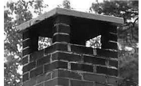
Concrete Cap Chimney Top
