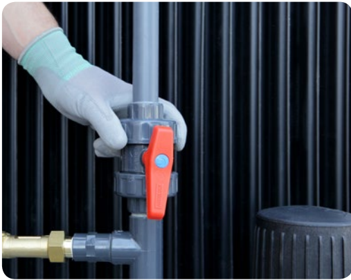
Unscrew the DN20 PVC-U ball valve fitting
